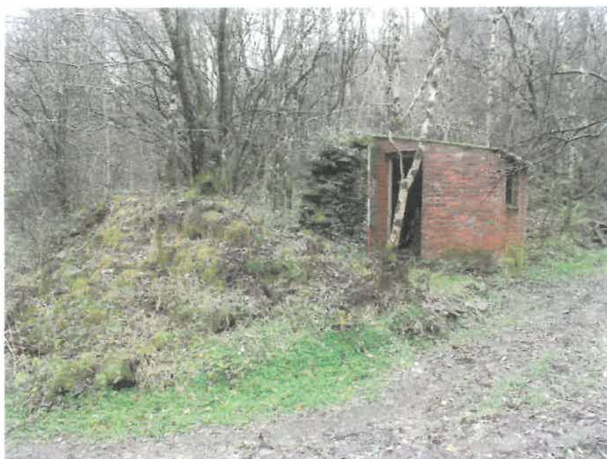
PRN 62320 Erw-lŵyd building. Photo CPAT 2282-013
