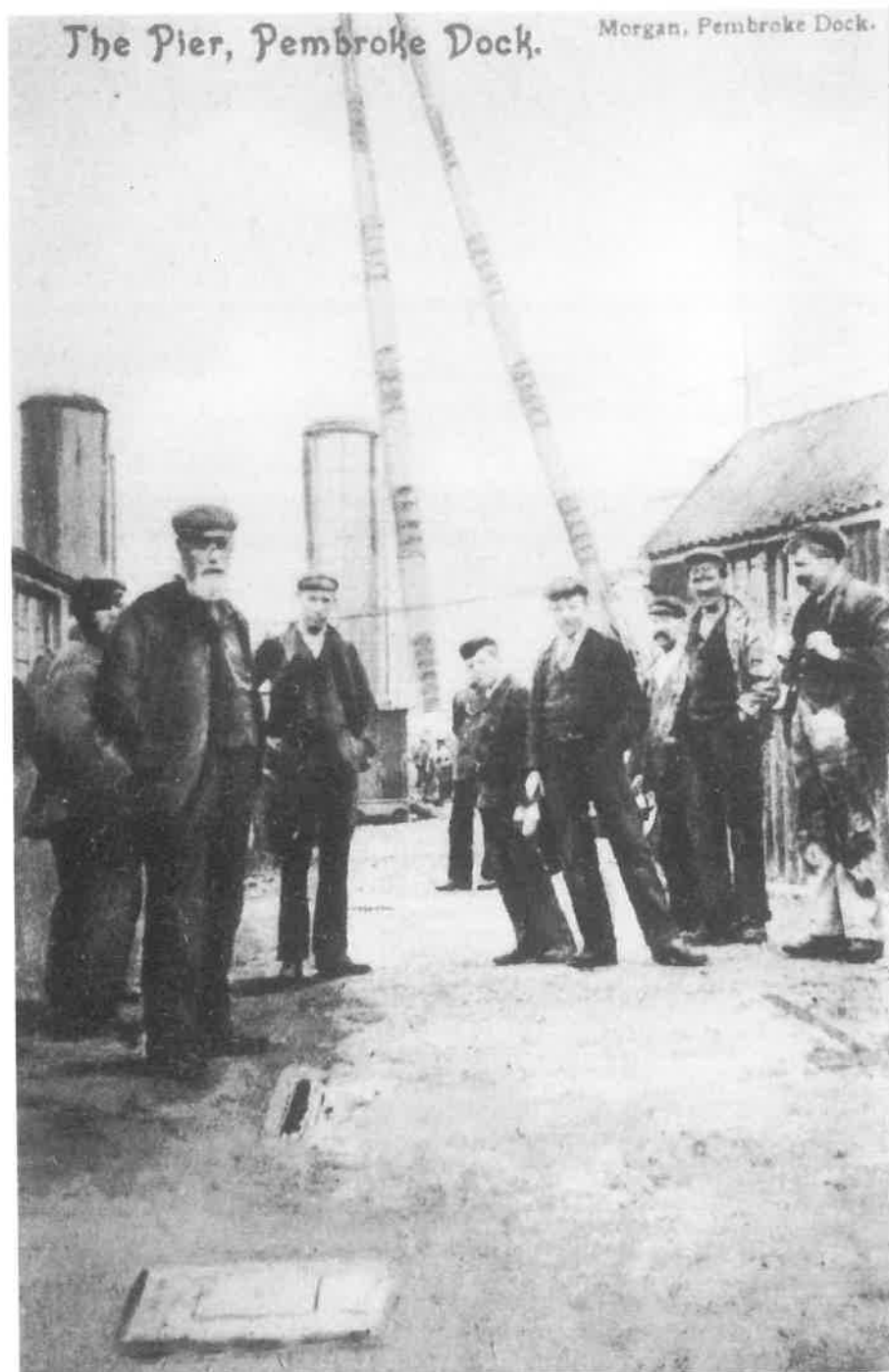
This view of dockyard workers at Hobbs Point was produced by the photographer Morgan (christian name unknown) who worked in the town for many years. Notice the huge sheer legs which were used to hoist heavy machinery into the newly launched ships.
