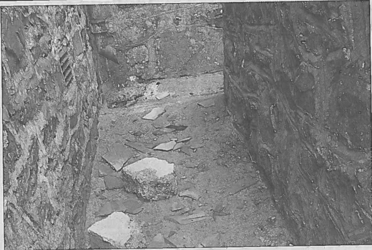
Some of the slates have fallen from the roof after being damaged.
