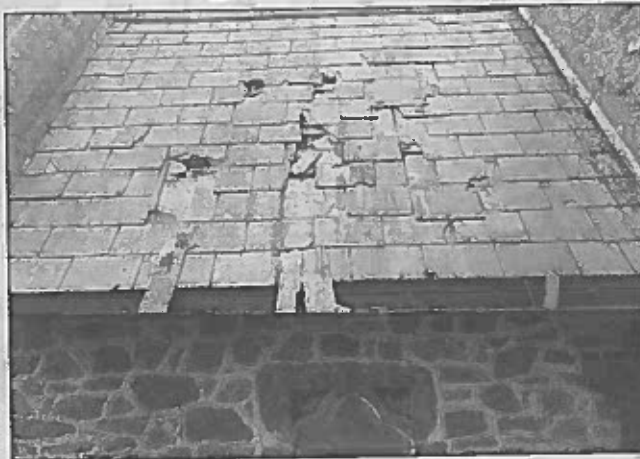
Damage to the roof of St David's Church, caused by stone throwing.
