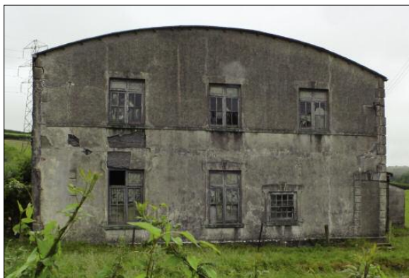
Figure 20. A building constructed with Belfast roof trusses which came from Pembrey munitions factory.
