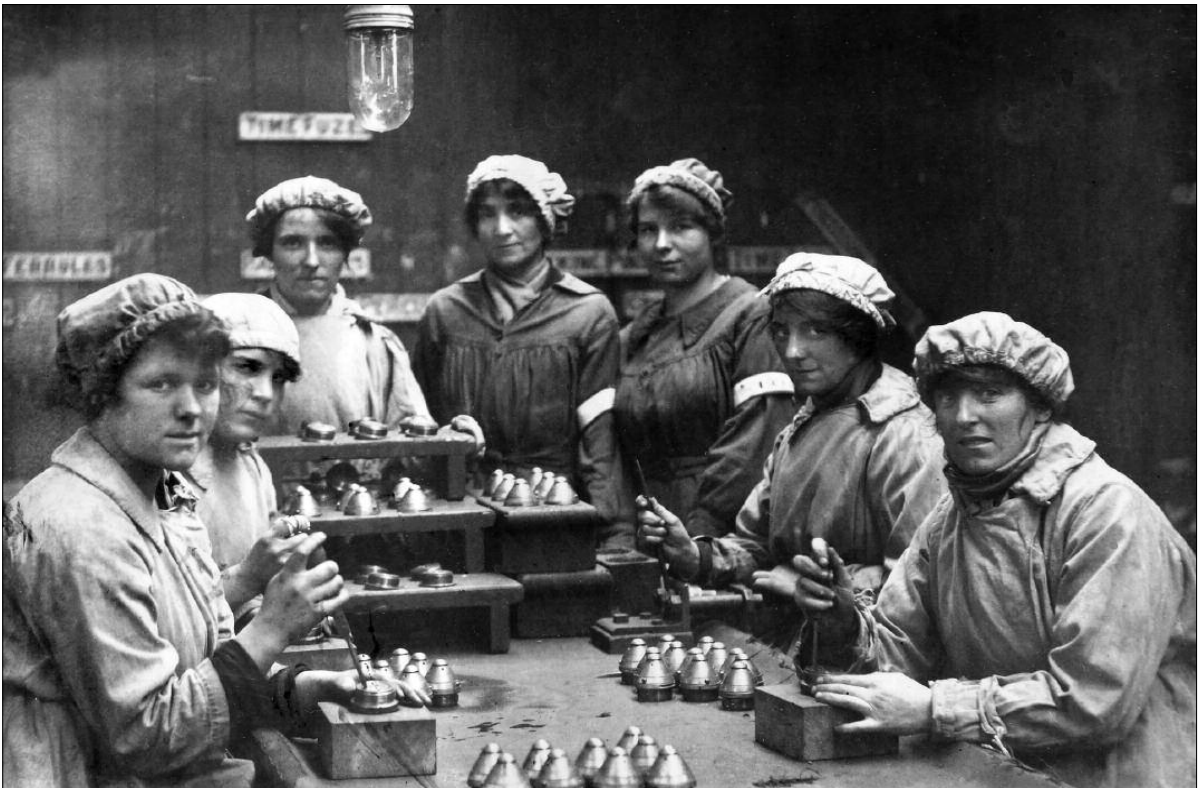
Figure 22. Removing plugs from time fuzes. (National Archives, MUN 5-155)
