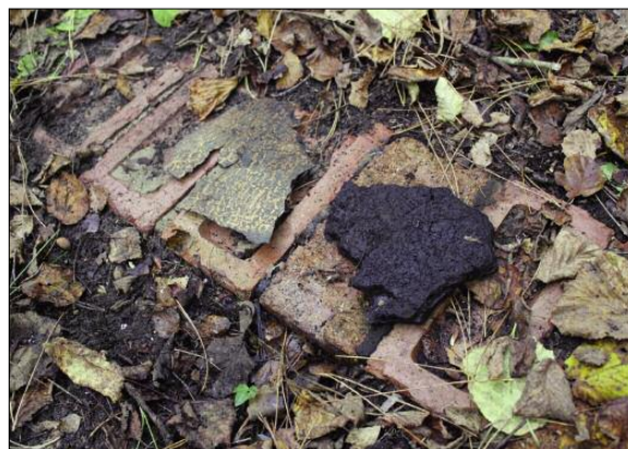
Figure 9. A brick foundation course for a timber structure
