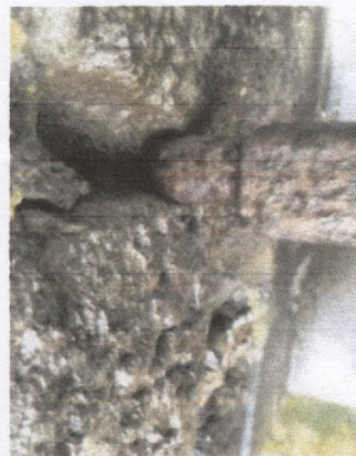
Photo 8 Detail of N side bearing of bell: the engagement with the bellcote masonry is minimal and precarious.
