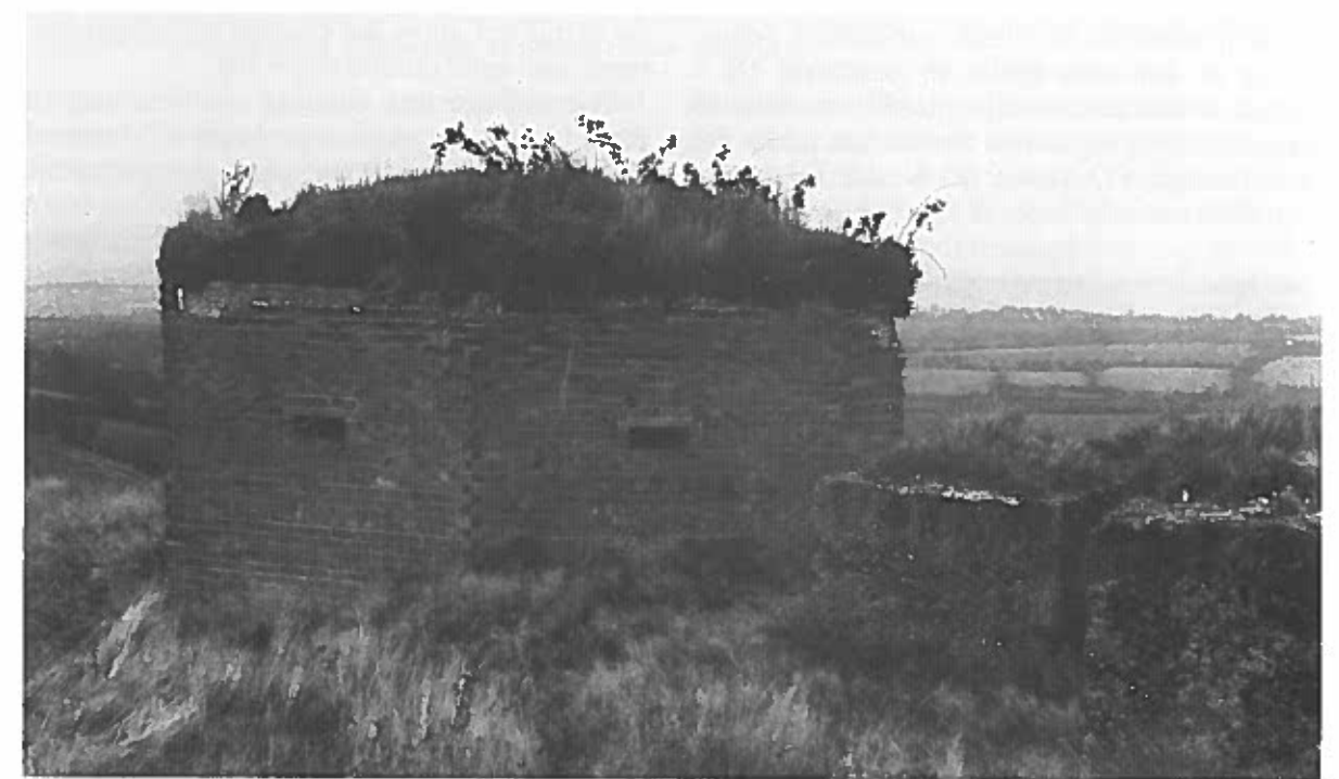
Fig. 3. Strong Post of hexagonal design, with 15 inch walls and shuttered with bricks, approved by the War Office as permanent shuttering on the exterior walls, due to the timber shortage. Located in the line of fortifications on Rhos Llangeler. (Photograph: de Gruchy-Glover collection).
