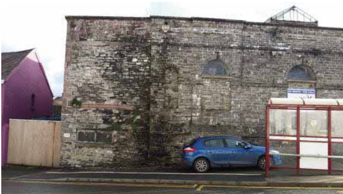
Figure 28 above: Contrasting market stonework along north west elevation highlighting different periods of construction and style
