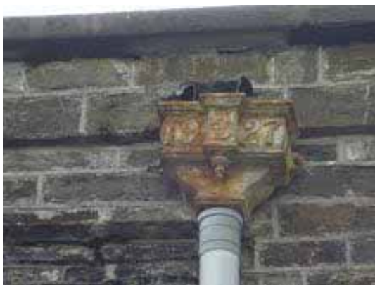
Figure 34 above: Hopper to market north west elevation
