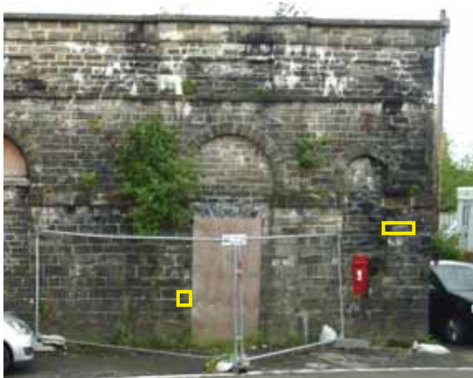
Figure 73 above: Missing stones highlighted in yellow and boarded up door to be replaced on southern end of market south west elevation
