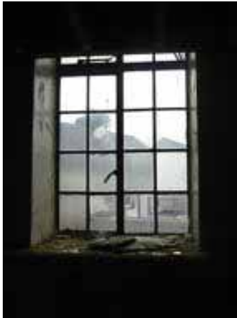
Figure 43, (left) Figure 44 (centre) and Figure 45 (right) above: typical rectangular metal windows inserted into the upper ground floor level of the north east elevation
