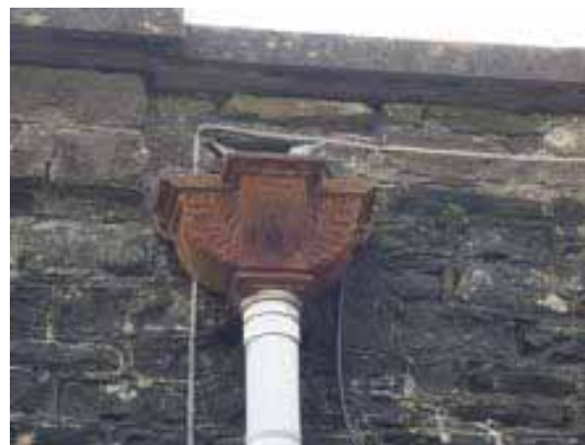
Figure 35 above: Hopper to market south east elevation
