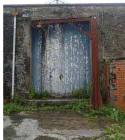
Figure 96 above: Solid door to be replaced with glazed door on market south east elevation with hoist retained
