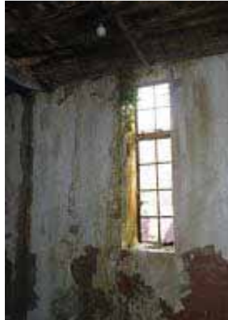
Figure 43, (left) Figure 44 (centre) and Figure 45 (right) above: typical rectangular metal windows inserted into the upper ground floor level of the north east elevation
