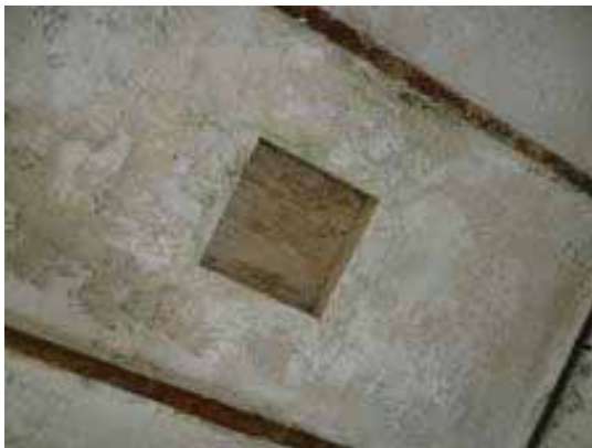
Figure 62 above: Boarded aperture to market flat roof
