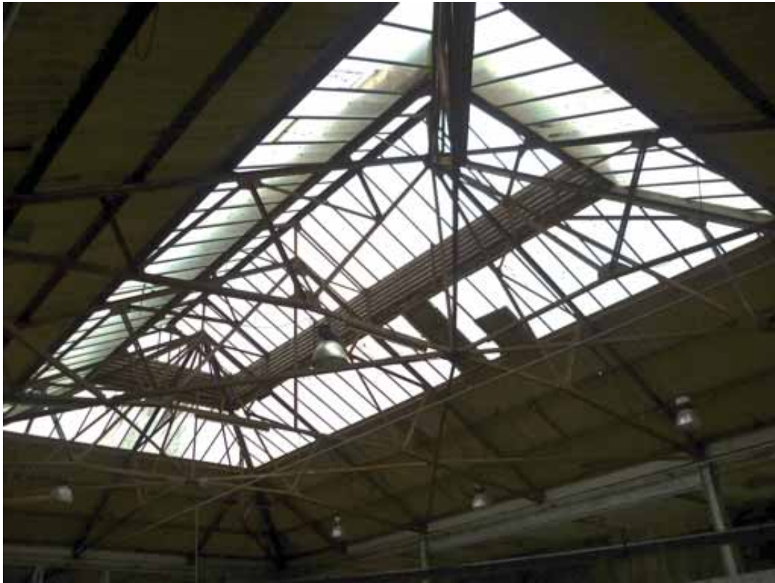
Figure 61 above: Glazed roof above market with early C20 steel trusses and uneven thickness glass panes
