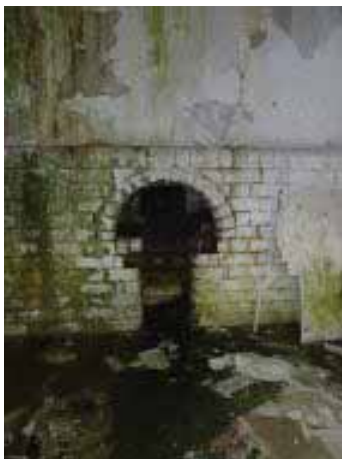
Figure 51 (left), Figure 52 (center) and Figure 53 (right) above: Market glazed bricks found in the central area of the north east wall only
