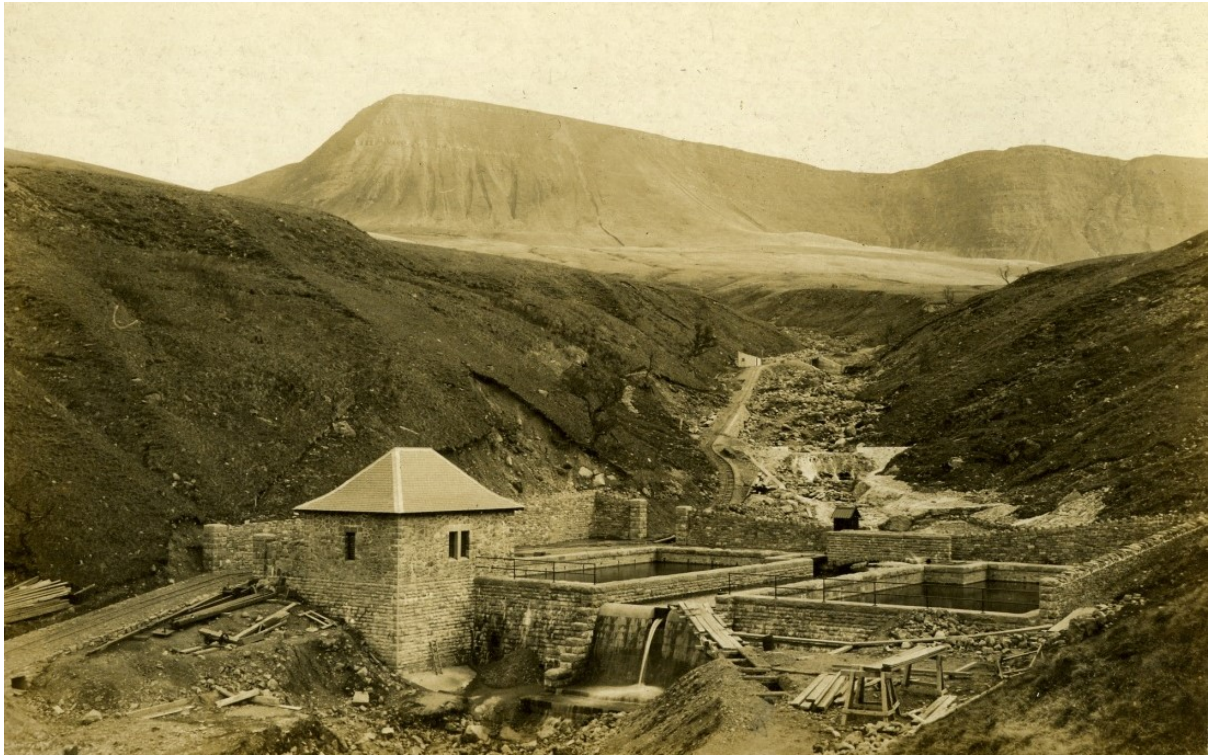
Figure 5: The valve house and filter beds under construction (Peter Davies collection)
