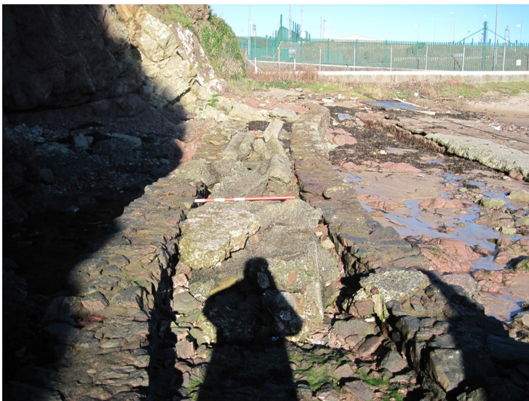
Photo 1: Inland part of slipway with broken up concrete repairs. View N. Scale 1m Modern slipway to right (East)
