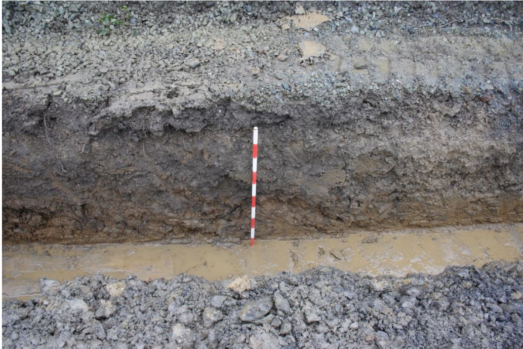
Photo 12: West facing section of drainage trench showing road make-up layers above natural ground
