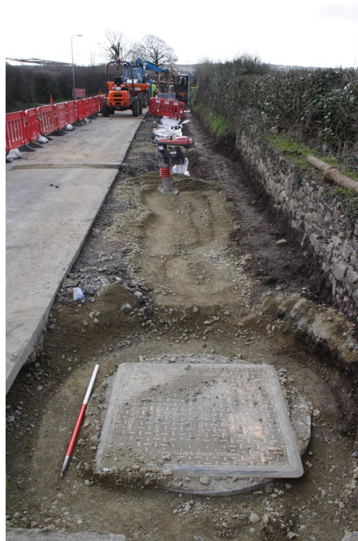
Photo 14: backfilling of drainage trench and inspection chamber cover, viewing south
