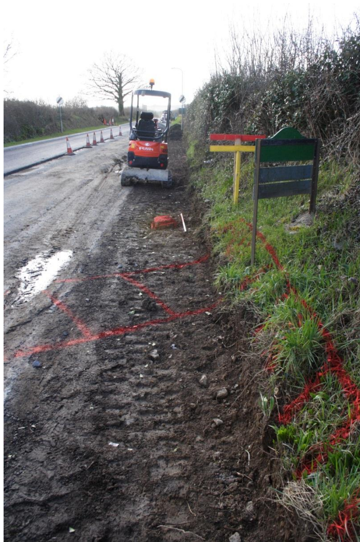
Photo 7: View south along western side of road showing removal of eastern edge of hedgebank and tarmac road surface
