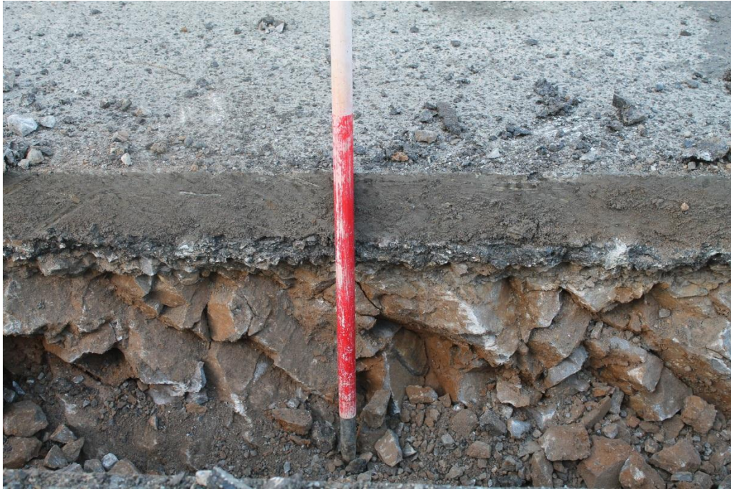
Photo 17: Drainage trench between Carew Castle and Carew Inn at the northern end of the road improvements showing road surface directly upon bedrock
