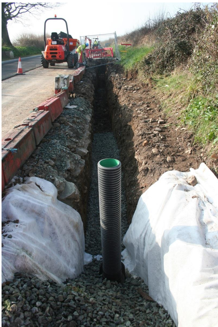
Photo 13: Backfilling of the drainage trench, viewing south
