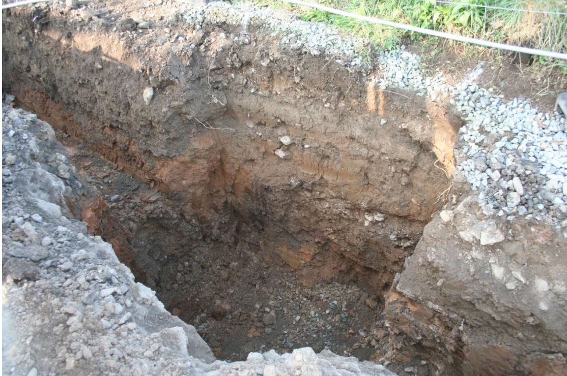
Photo 10: Excavated area for inspection chamber
