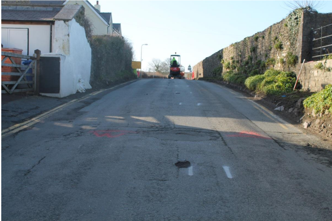
Photo 15: View south along A4075 showing white lines marking line of drainage trench through existing road surface
