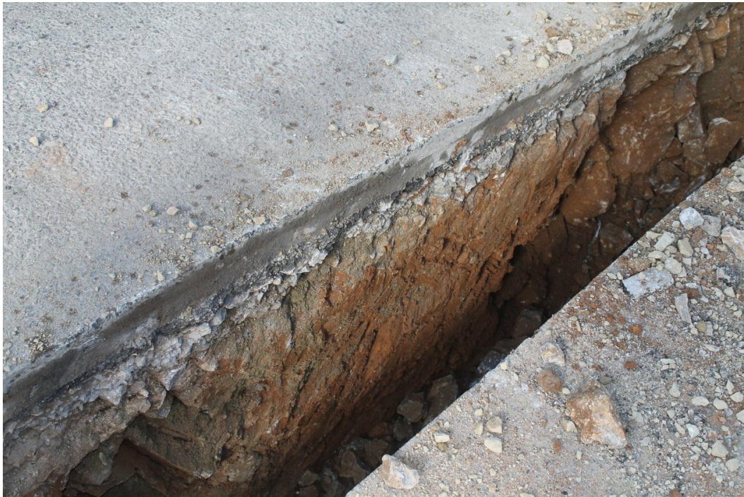
Photo 16: Drainage trench between Carew Castle and Carew Inn at the northern end of the road improvements showing road surface directly upon bedrock
