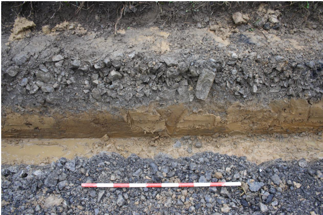
Photo 11: East facing section through drainage trench showing depth of stone backfill for former water pipe
