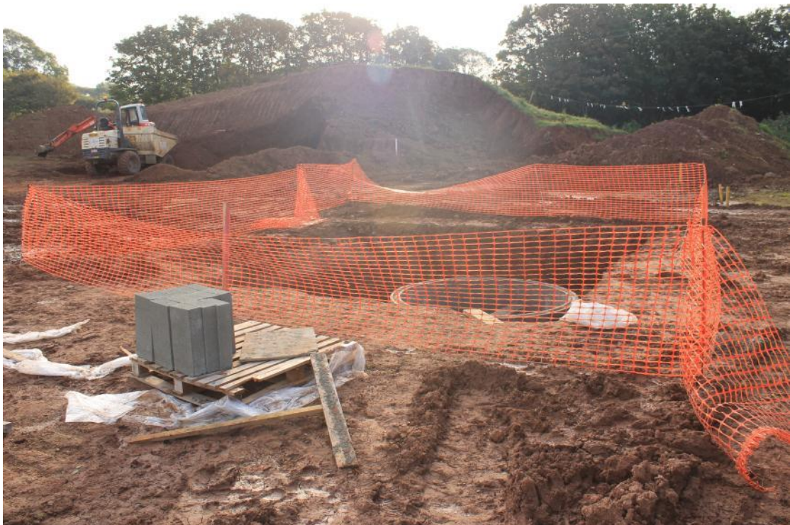
Photo 10: View southeast across area of attenuation pond with culvert connection in foreground and spoil heap to rear
