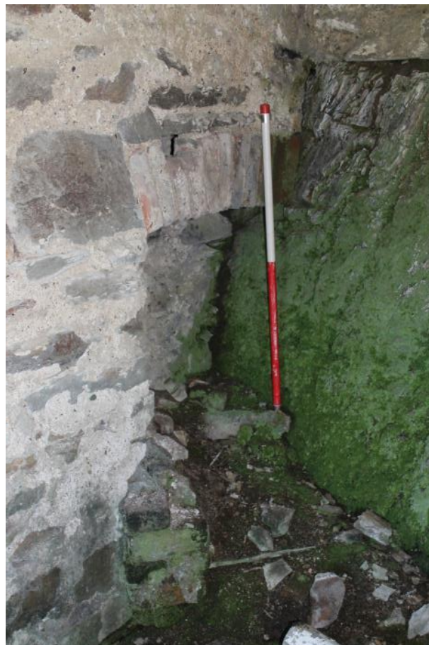
Photo 19: Possible former leat opening (in northwest gable end wall) for channelling water in/out of mill. Later converted to a fireplace.
