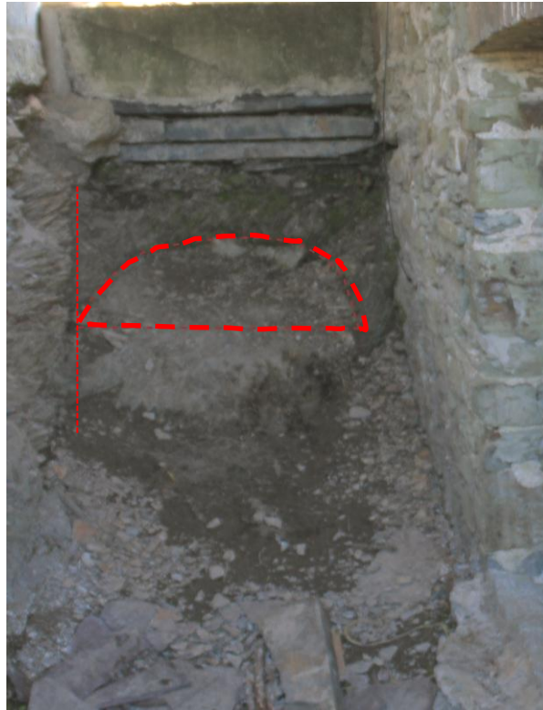
Photo 15: Rock-cut possible leat (red semicircle) at back of former wheelpit. Vertical line indicates the edge of the possible wheelpit cut.
