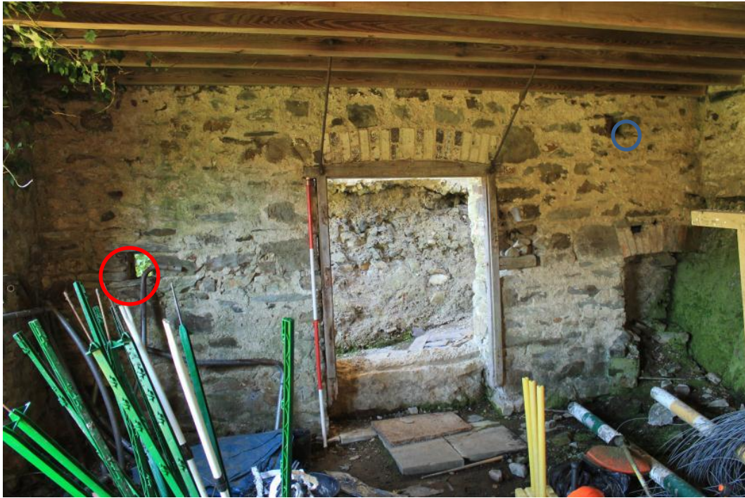
Photo 20: Interior ground floor southeast facing wall with wide opening to wheelpit. Note possible drive-shaft hole to left (circled in red) and niche for beam (circled in blue).
