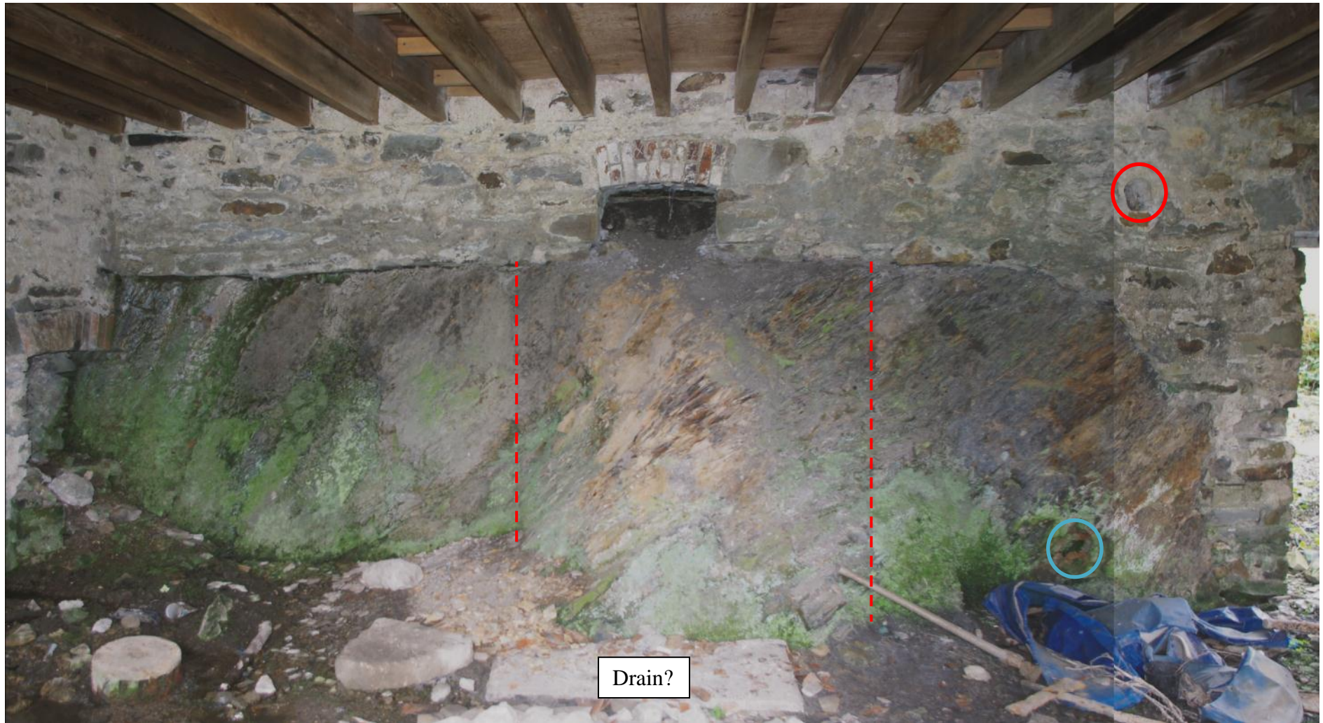
Photo 17: Natural shale bedrock foundation to the northeast wall (southeast facing). Note niche for beam (circled in red) and vertical cut faces (dashed lines)
