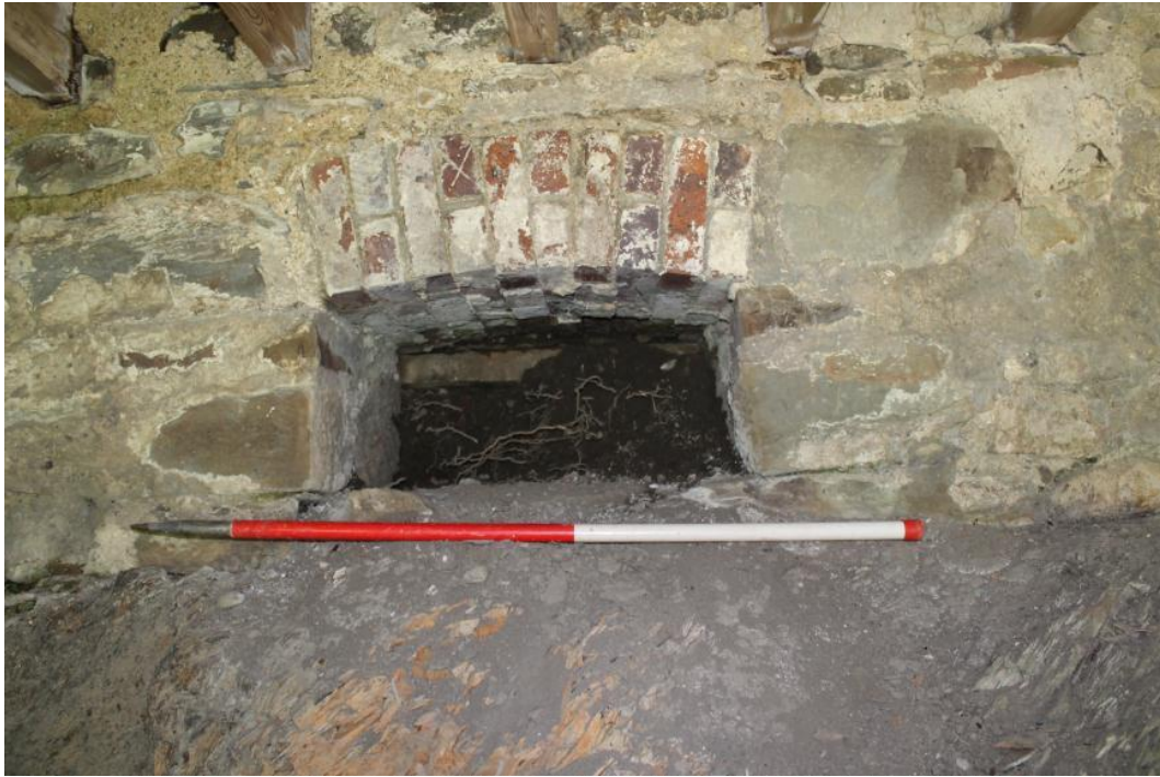
Photo 18: Inlet in northeast wall from main leat into mill building
