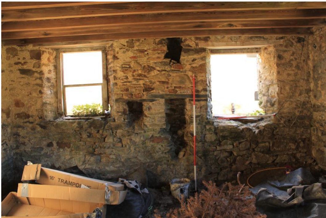
Photo 21: Northwest facing interior ground floor elevation (southeast gable end). Small hearth, recess and void in chimney breast (above).
