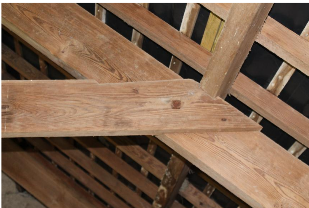
Photo 26: Detail of tie beam
