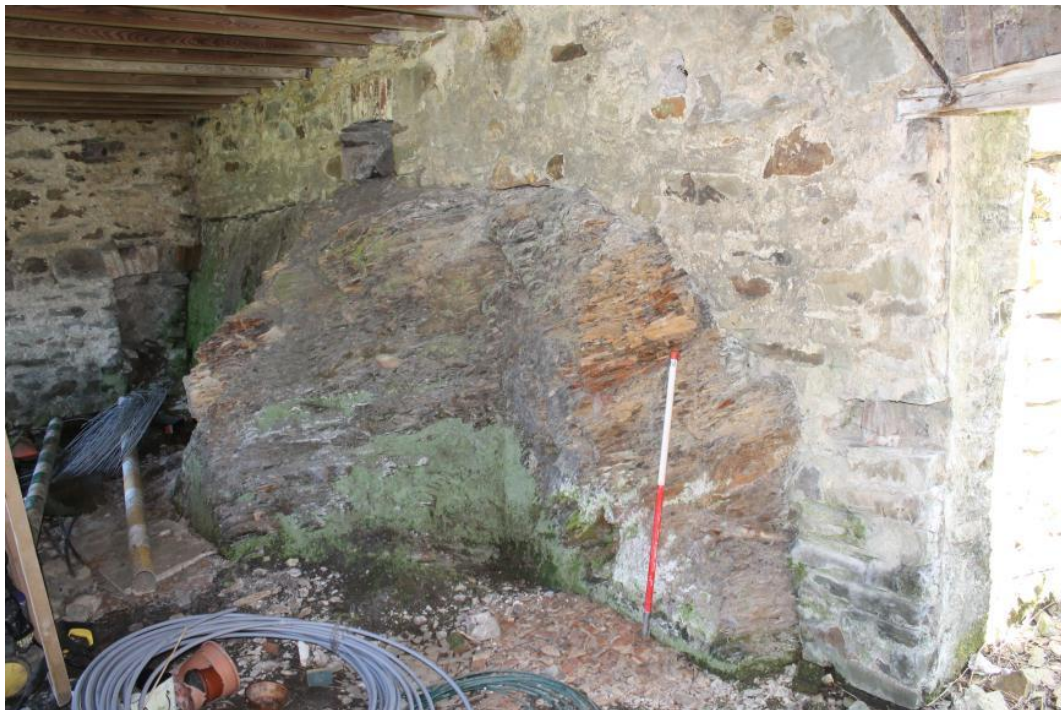
Photo 16: Bedrock outcrop on ground floor. Note shaping of rock to form right angled vertical faces, possibly to house a fulling tank?
