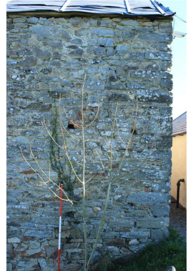
Photo 5: Putlog holes on southwest facing exterior elevation
