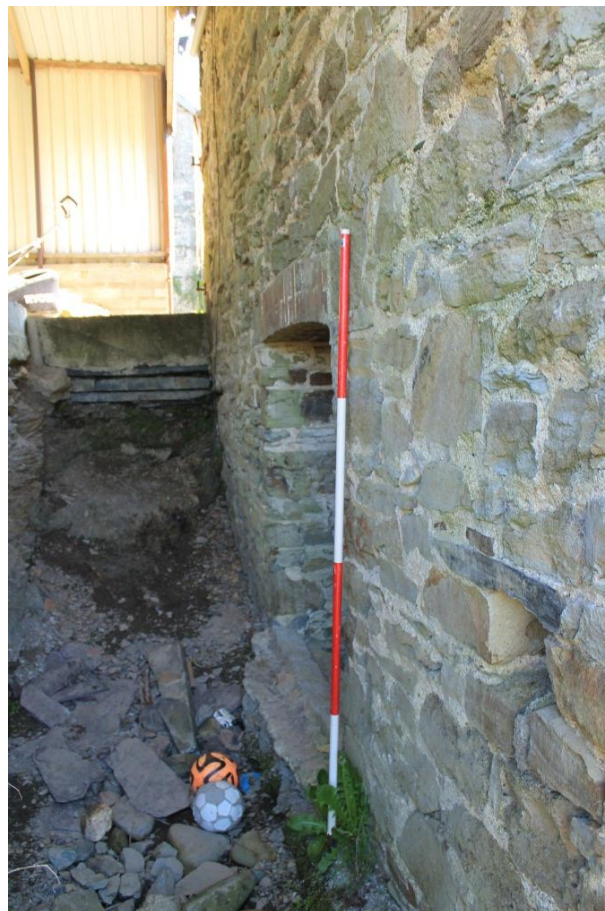
Photo 14: Northwest facing gable end elevation (lower part- possible former wheelpit and later sheep dip), with door opening and possible opening for drive-shaft in wall to right of picture.
