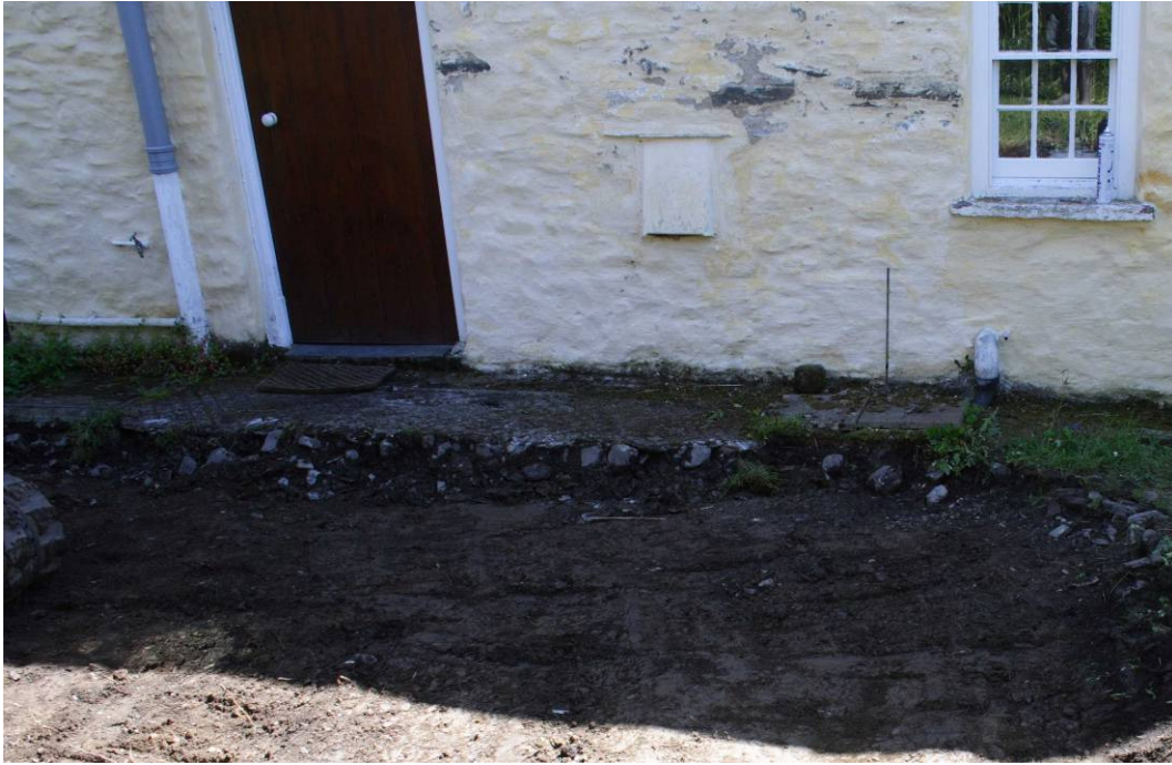
Photo 3: Concrete capped drainage runs adjacent to Lisburne House following removal of cobbles
