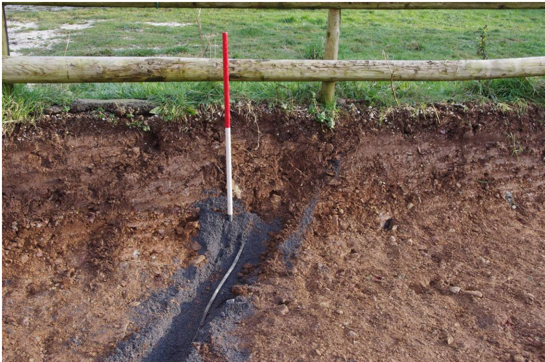
Photo 3: Detail of depth of ground reduction in southeastern corner of site and exposed cable trench
