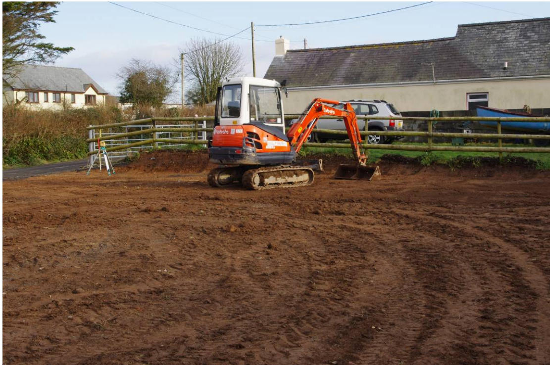
Photo 2: View towards the southeastern corner of the building footprint showing the depth of required ground reduction
