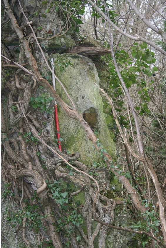
Photo 25: 1 st floor window remains in the southern wall of the Western Tower, also showing surviving timber lintel. 1m scale.
