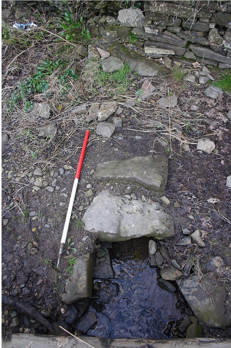
Photo 53: Culverted stream running out from underneath the Southwest Enclosure, looking north. 1m scale.
