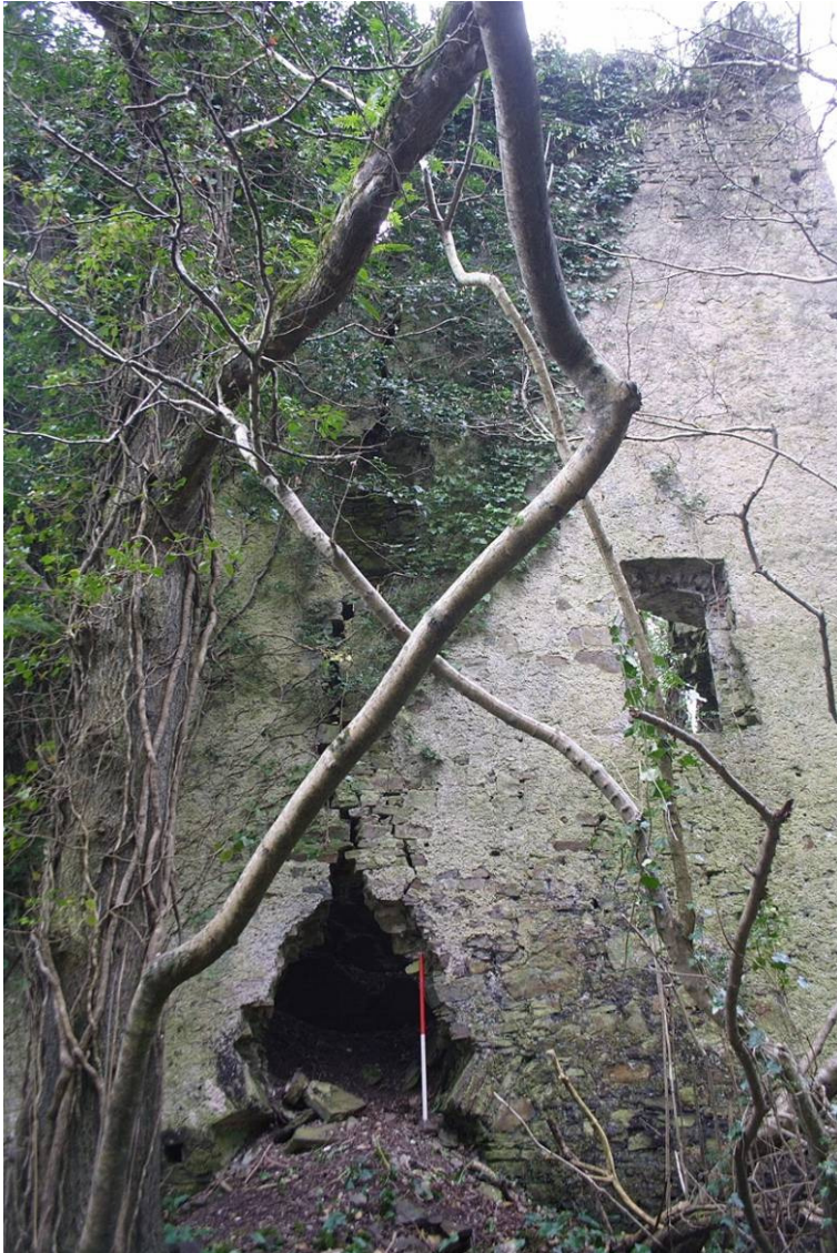
Photo 9: Closer view of the collapsed archway and vertical crack above. 1m scale.
