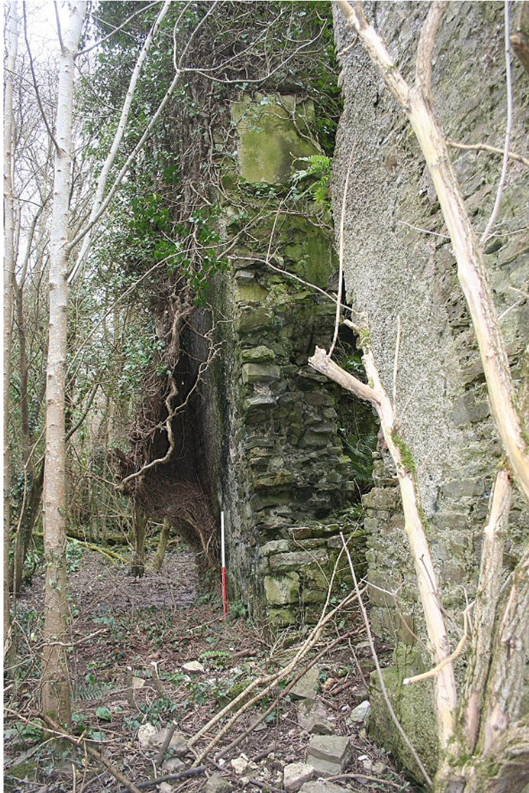
Photo 17: Looking north along the western wall of the Western Tower, showing the outward lean. 1m scale.
