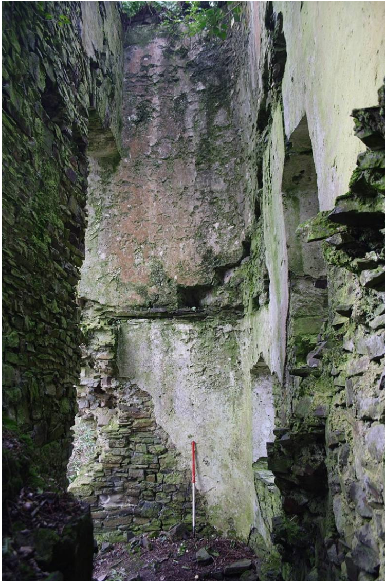
Photo 13: Interior of Eastern Tower showing pinker internal render on 2 nd floor. 1m scale.
