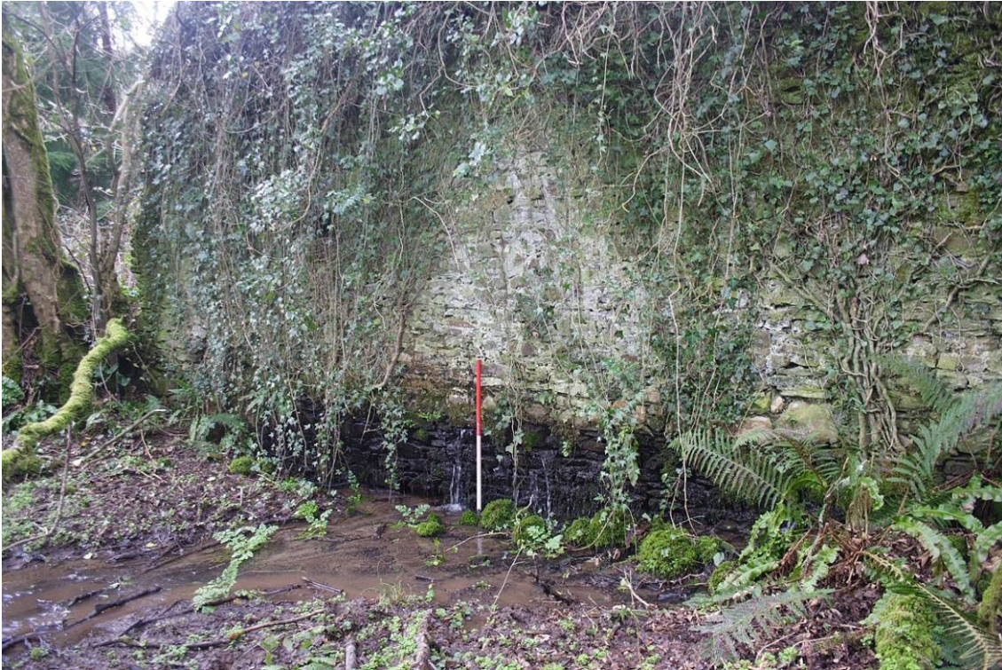
Photo 51: Water seeping through the northern wall of the Northwest Enclosure. 1m scale.
