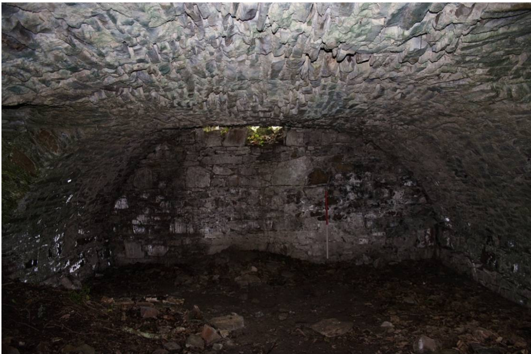
Photo 32: The interior of the undercroft looking west, showing the collapse in the ceiling and upper courses of the western wall. 1m scale.
