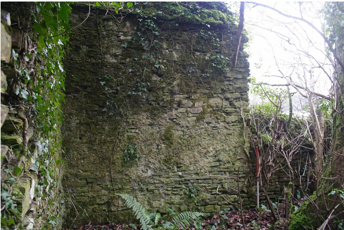
Photo 42: Interior of the southern wall at the southeast corner of the Garden Enclosure. Straight vertical joint visible to the left of the 1m scale.
