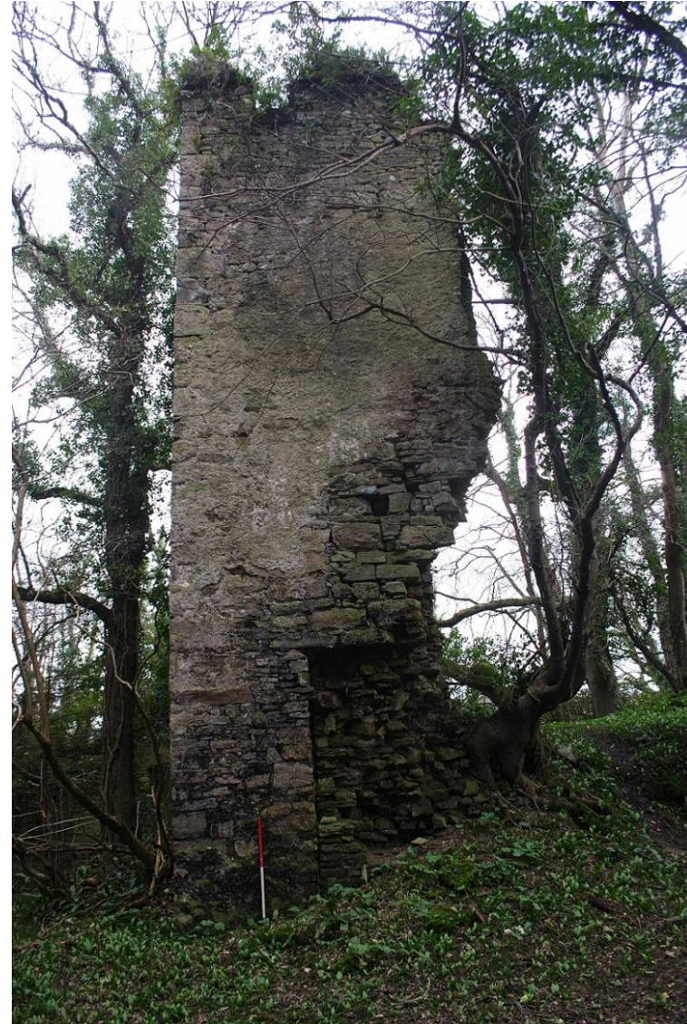
Photo 10: Northern face of Eastern Tower, clearly showing earlier segment of walling. 1m scale.
