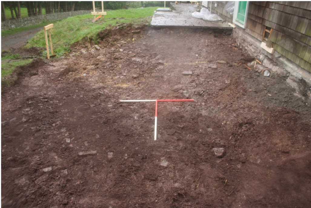
Photo 4: Northern area of extension after initial machining to formation level. Note the rubble spread and stone footings for bungalow to the south.
