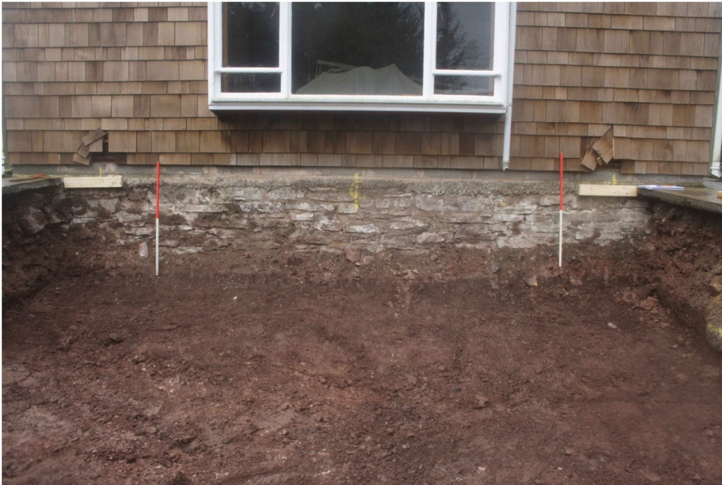
Photo 1: Eastern extension area following machining. Note the stone wall used as footing for bungalow.
