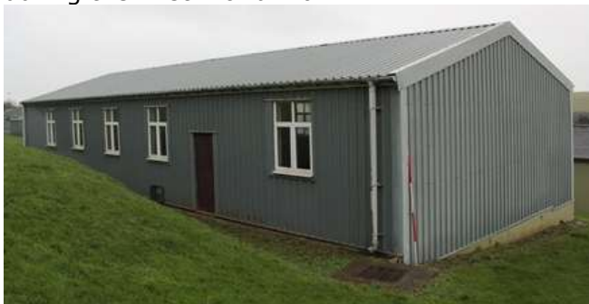
PRN 107812: Lecture room has been re-clad in box-profile corrugated sheeting.
