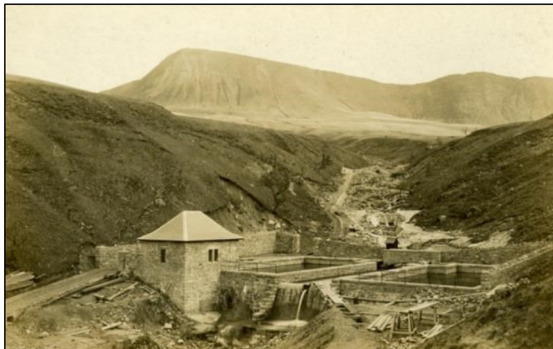
Figure 18: Construction of the filter beds in progress (Mary Walmsley)
