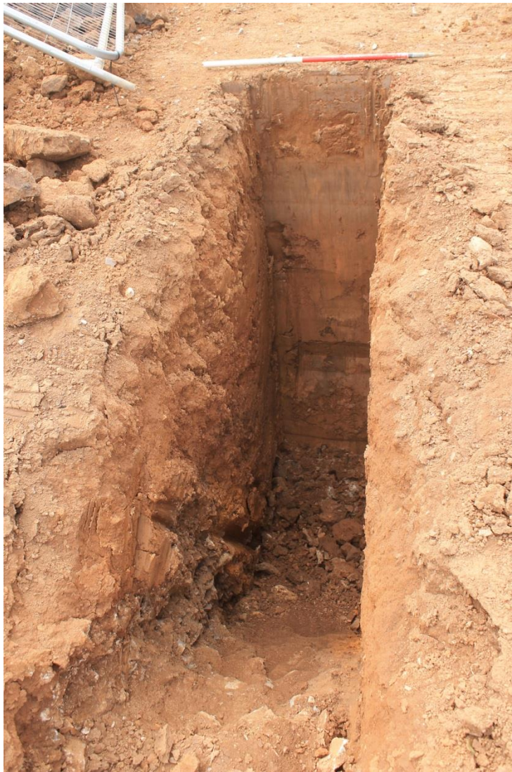
Photo 6: Looking south – showing a section of foundation trench showing an example of one of the silt filled deep fissures present across site.
