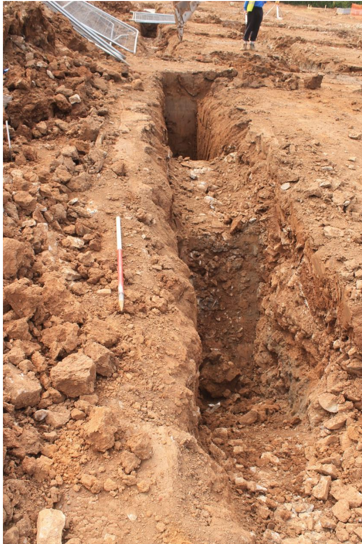
Photo 5: Looking south – showing a section of excavated foundation trench illustrating the undulating nature of the natural bedrock geology.
