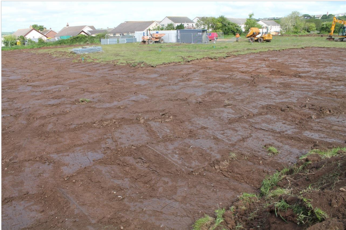
Photo 1: General shot of area topsoil stripped to subsoil interface. Looking northwest towards the contractor's compound.
