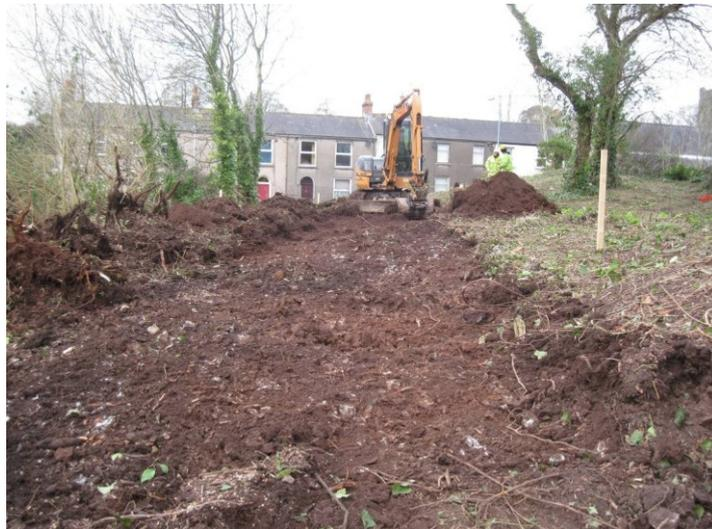
*Photograph of the topsoil strip for the cycle way at Monkton.*
