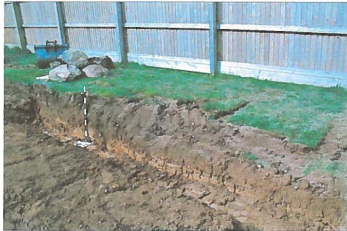
*Kisongo building plot showing topsoil directly over clay geology.*
