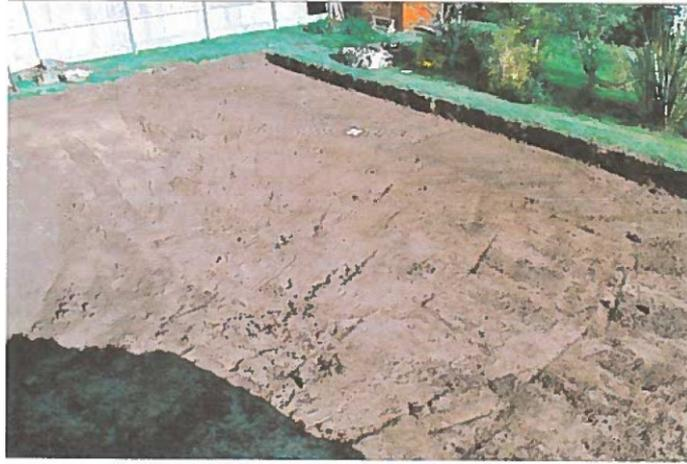
*Topsoil stripped from Kisongo building plot.*
