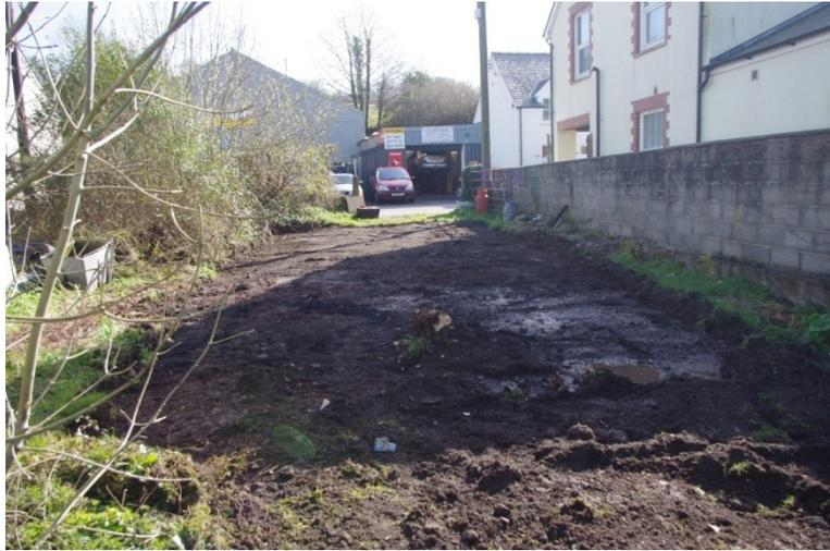
*The completed topsoil strip at Plot 1, Eldon.*
