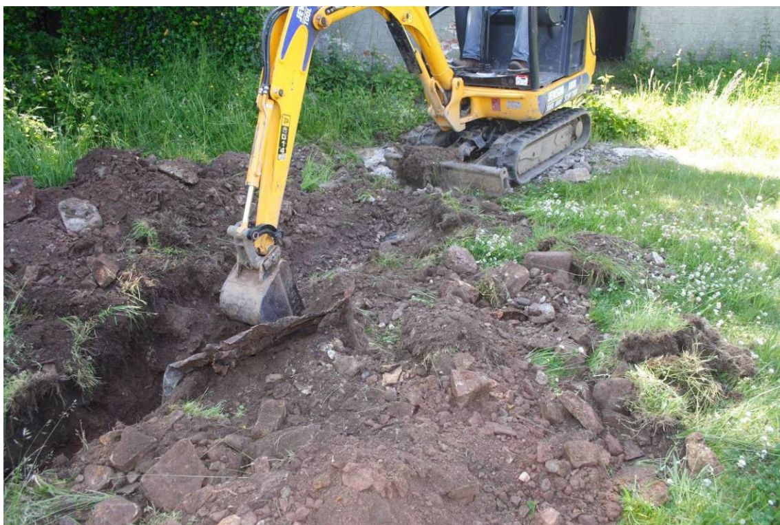
Photo 10: Excavation of south-west aligned drainage trench showing mixed nature of soils containing fragments of stone, metal and other detritus
