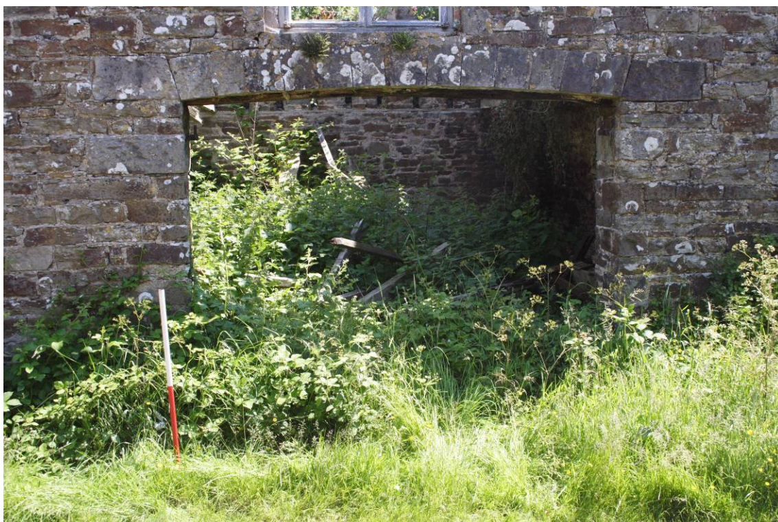
Photo 5: Southern cart entrance (2.8m in width and 2.14m in height)
