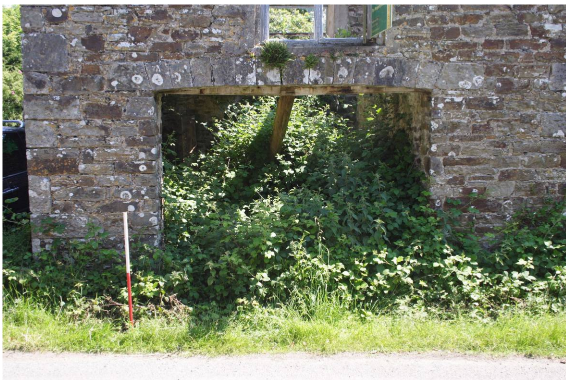
Photo 4: Northern cart entrance (2.6m wide and 2.18m in height)
