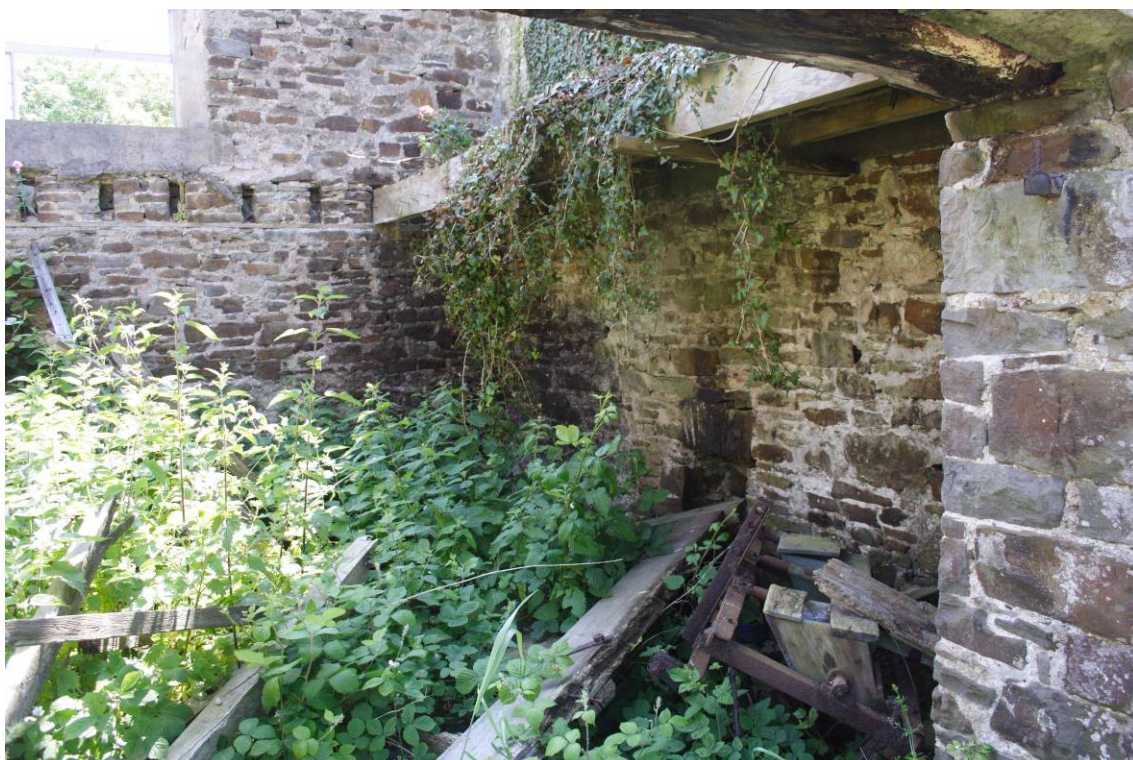
Photo 3: Fireplace on southern gable end of building at ground floor level, showing collapsed roof and floor joists within cart shed
