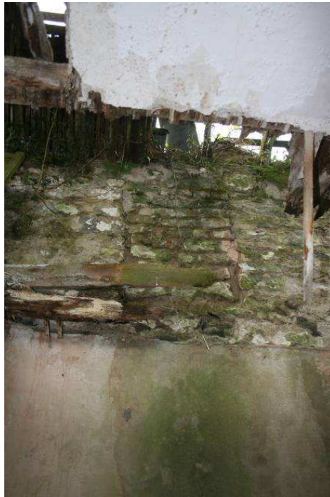
Photo 16: Former first floor window in west wall blocked with stone (see also Photos 8 & 10).
