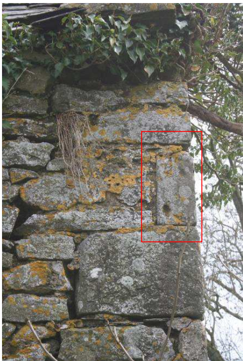
Photo 11: A dressed block with a block with part of a socket
