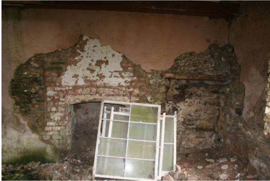
Photo 20: North wall, showing inserted brick fireplace and chimneystack and doorway to right, with wooden lintel and blocked with stone.
