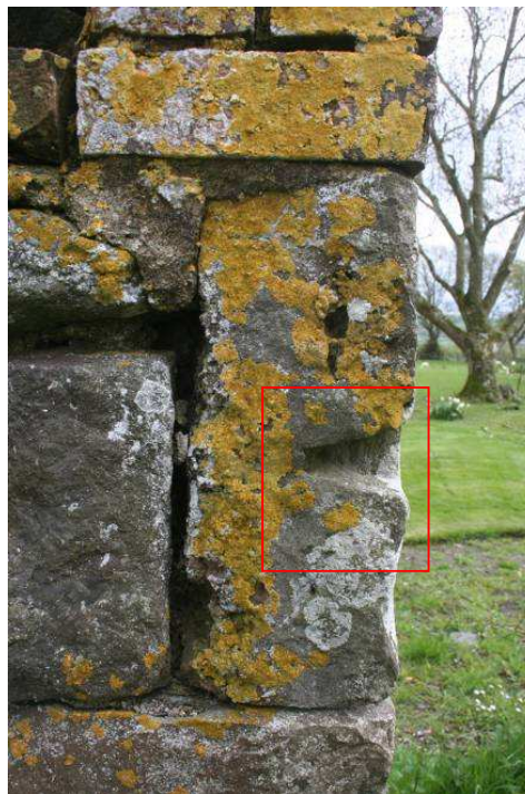
Photo 12: Another dressed possible shallow socket
