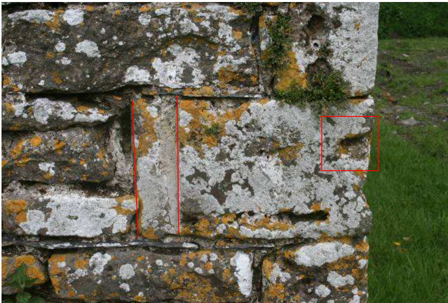
Photo 6: Stone with carved moulding. This stone may be part of a former window opening
