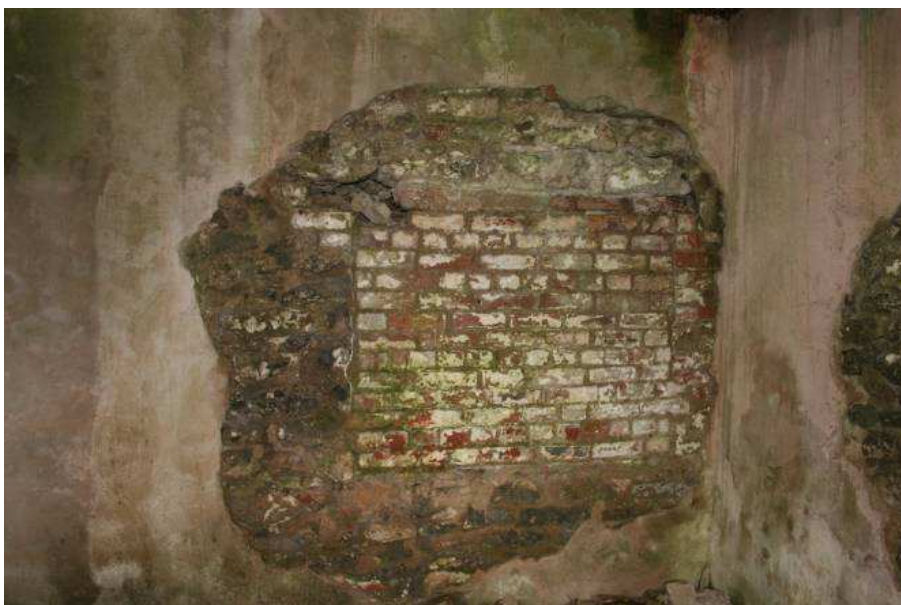
Photo 23: Brick-blocked window at the north end of the western wall (see also Photo 9).
