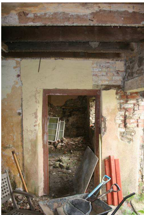
Photo 17: Ground floor dividing wall, constructed of brick
