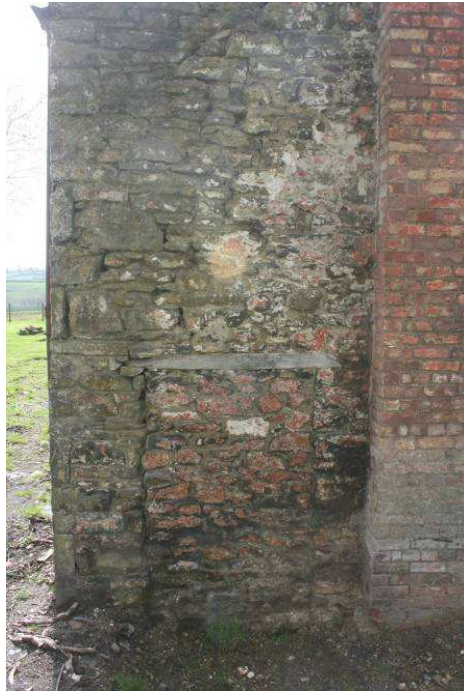
Photo 14: Blocked doorway in north gable end
