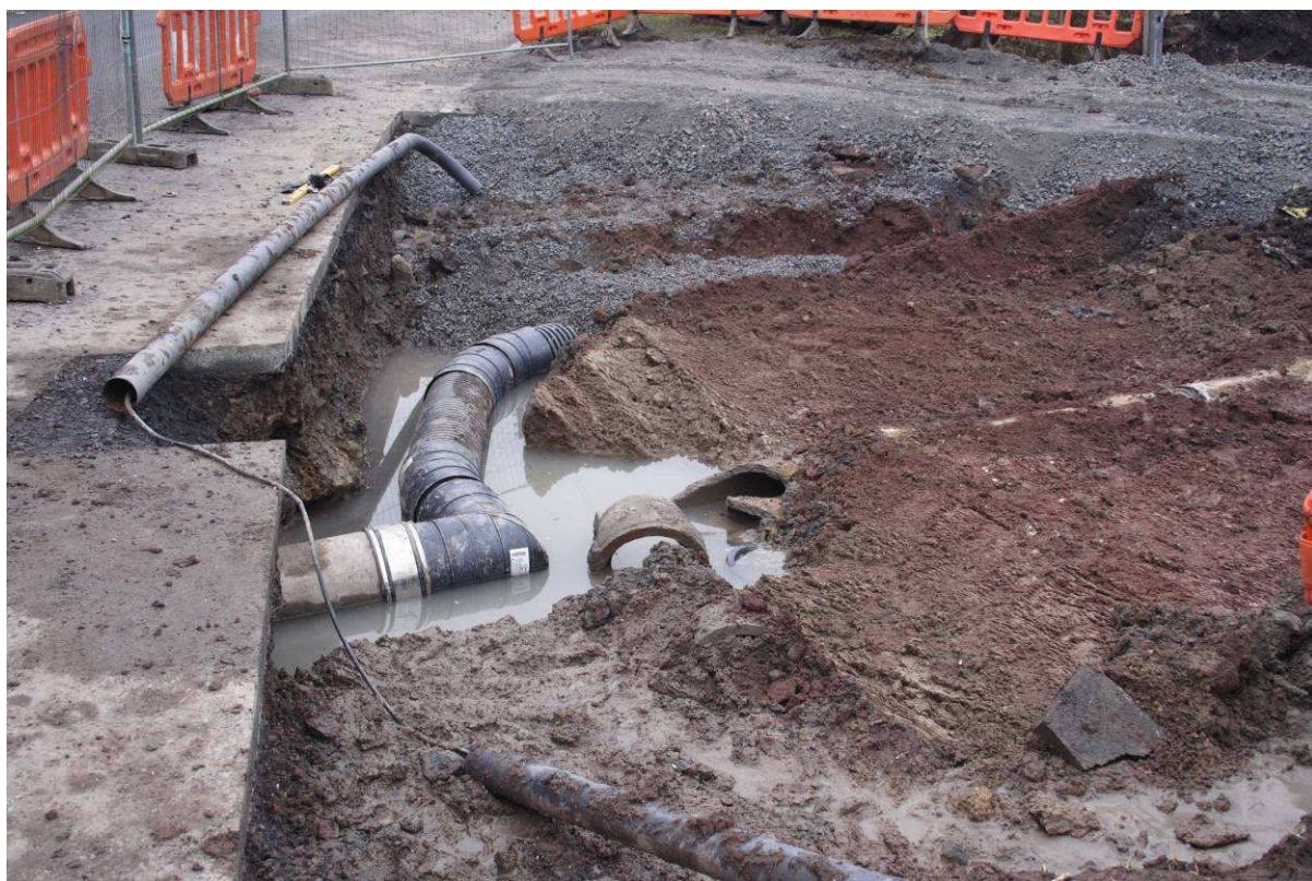
Photo 5: Working area of CSO following soil strip to top of existing sewer and showing replacement sewer pipe connection, view north
