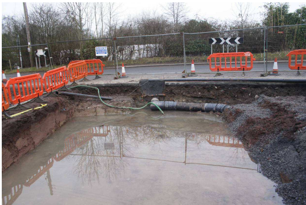
Photo 7: CSO working area stripped into natural substratum, view west
