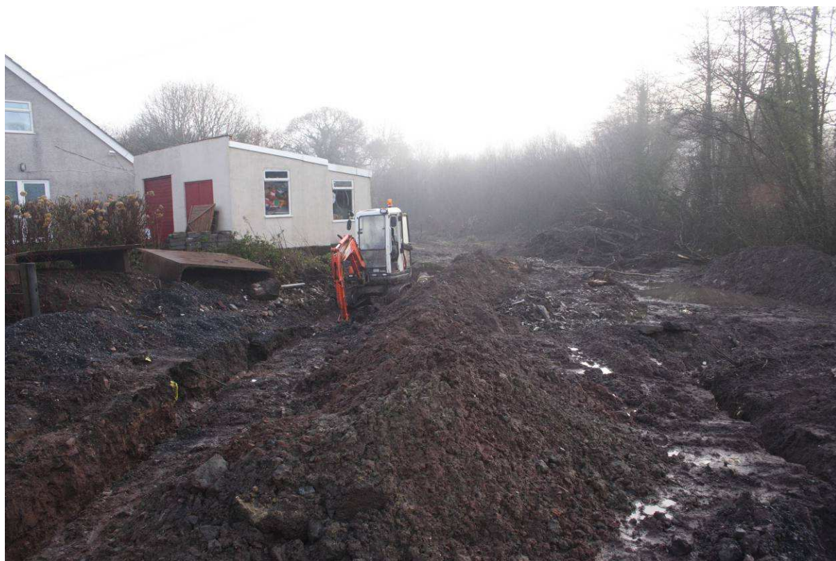
Photo 1: View east along line of existing sewer, showing waterlogged ground conditions
