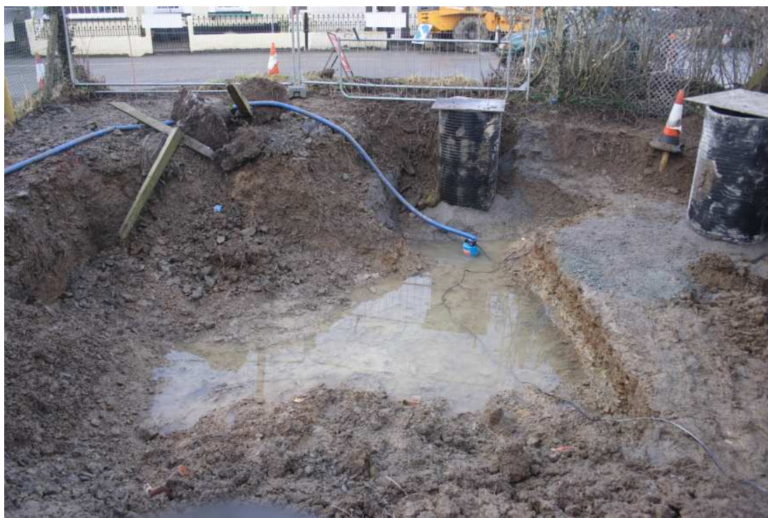
Photo 1: Photo south west showing excavated footprint for sewage pumping station.
