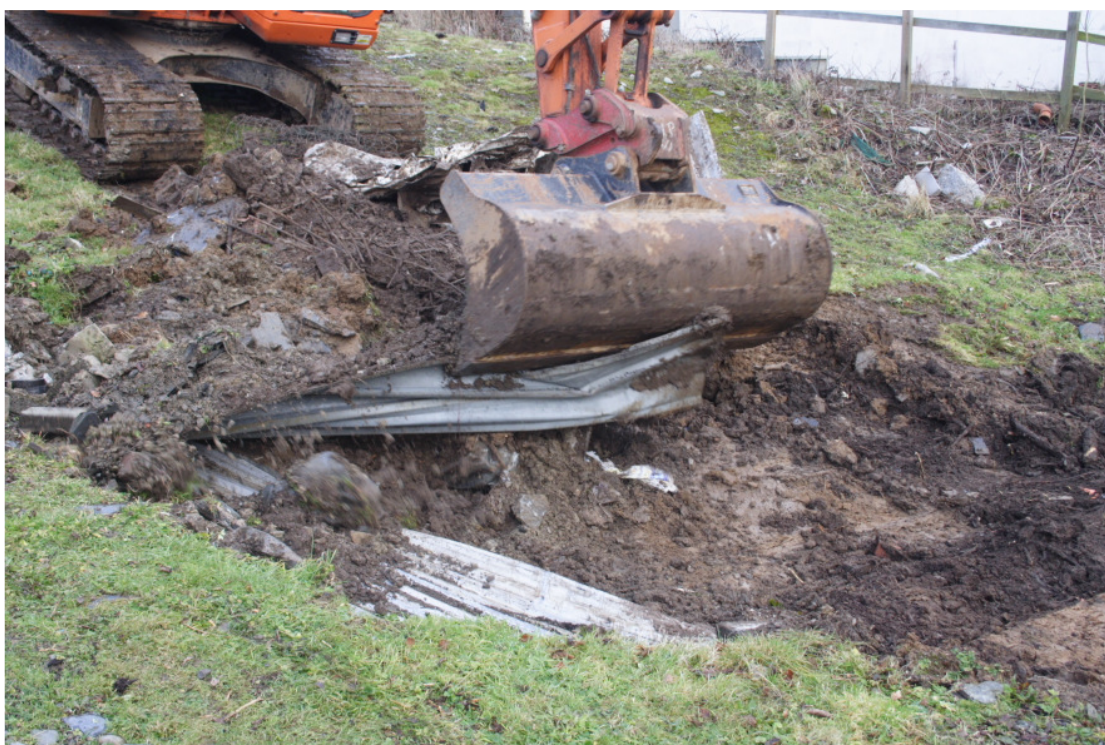
Photo 2: Photo showing removal of modern debris.
