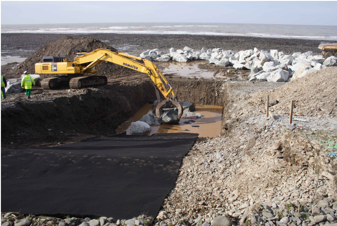
Photo 7: Laying boulders to form sea defences within trench
