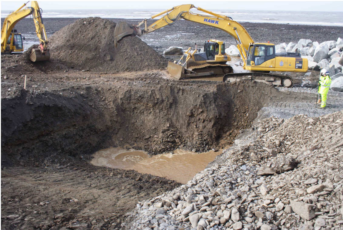
Photo 5: Excavation of trench close to Castell Cadwgan to lay new sea defences
