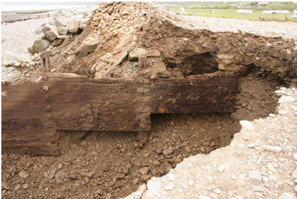
Photo 2: Exposure of existing groyne prior to removal
