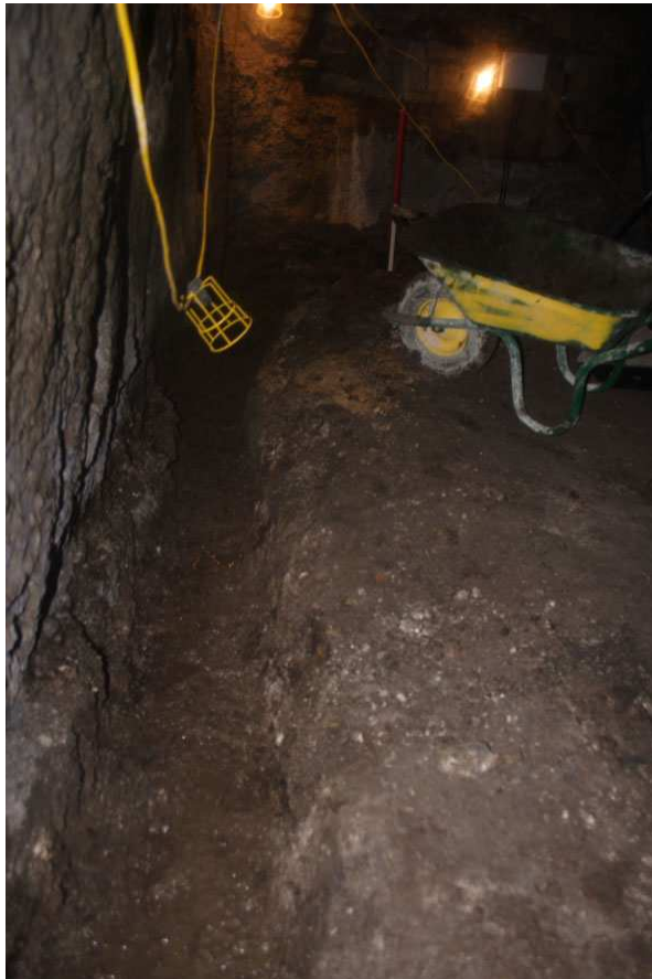
Photo. 5: Looking north along western wall of undercroft showing rock cut drainage channel.
