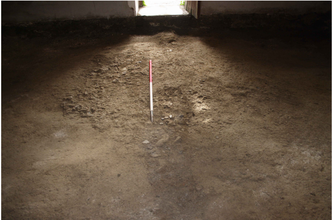
Photo 11: Line of root damage through clay and mortar floor, which caused damage during 20 th century to tiled floor above
