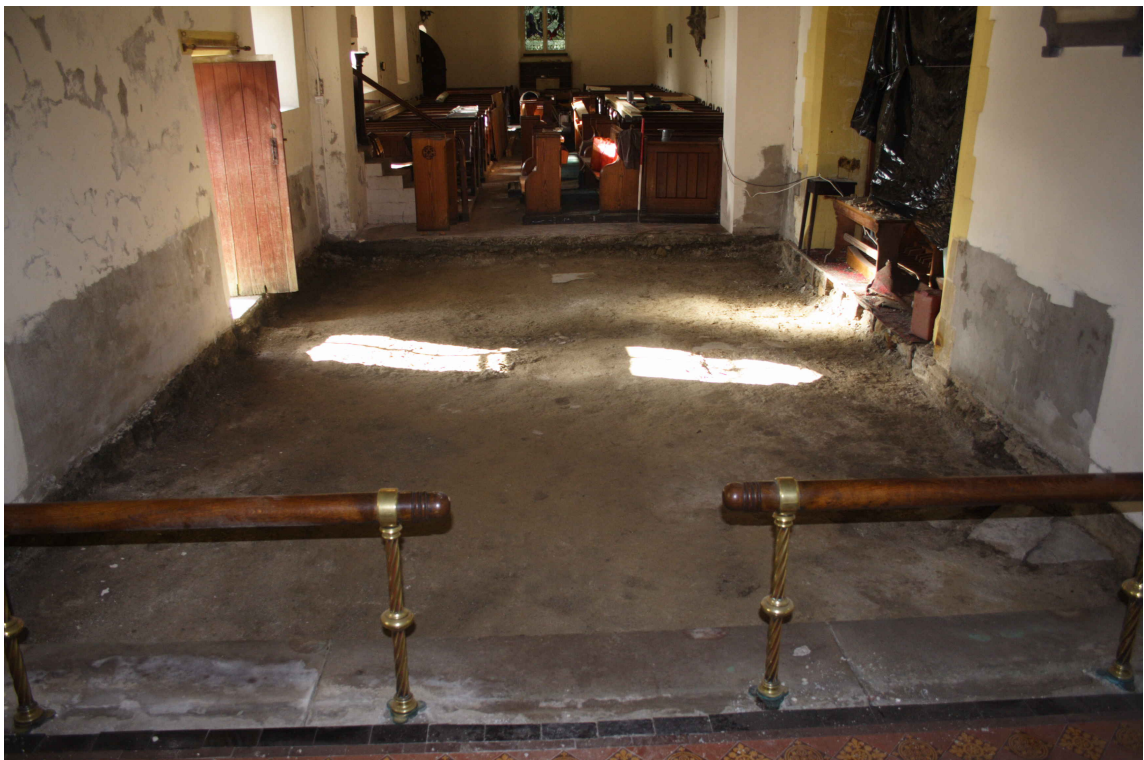
Photo 12: Overall view facing west of chancel following excavation of concrete floor and rubble, immediately prior to backfilling with material for new flooring
