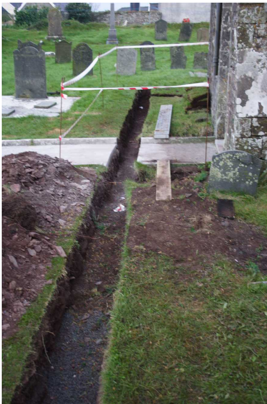
Photo. 1: West facing section of Drainage pipe cut.
