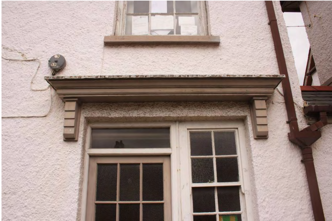
Photo 24: Stone cornice above doorway entrance of western building on Caradoc Road frontage
