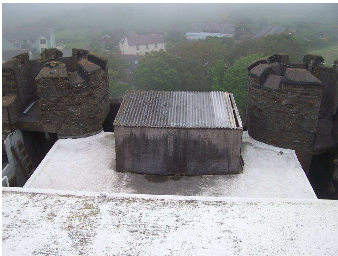
Photo 26: Asbestos structure housing water tank above Room 11, viewed from the modern roof above Room 12. The two turrets are visible in the background.
