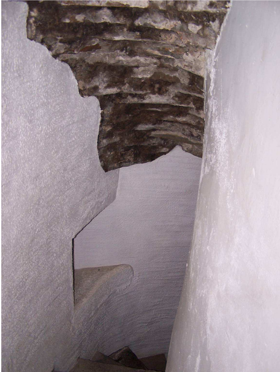
Photo 24: View south down staircase on southeastern part of castle, showing underside of original staircase above
