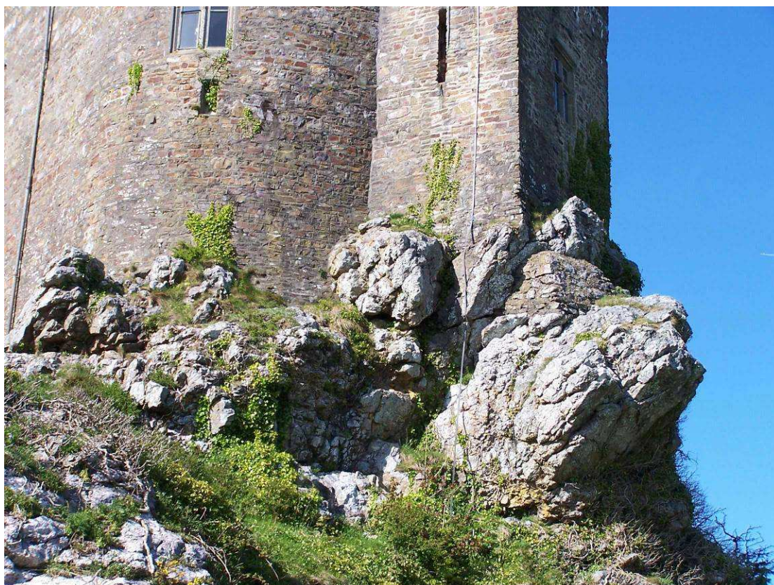
Photo 36: Southwestern elevation of Roch Castle showing how walls have been built directly upon the rock outcrop.
