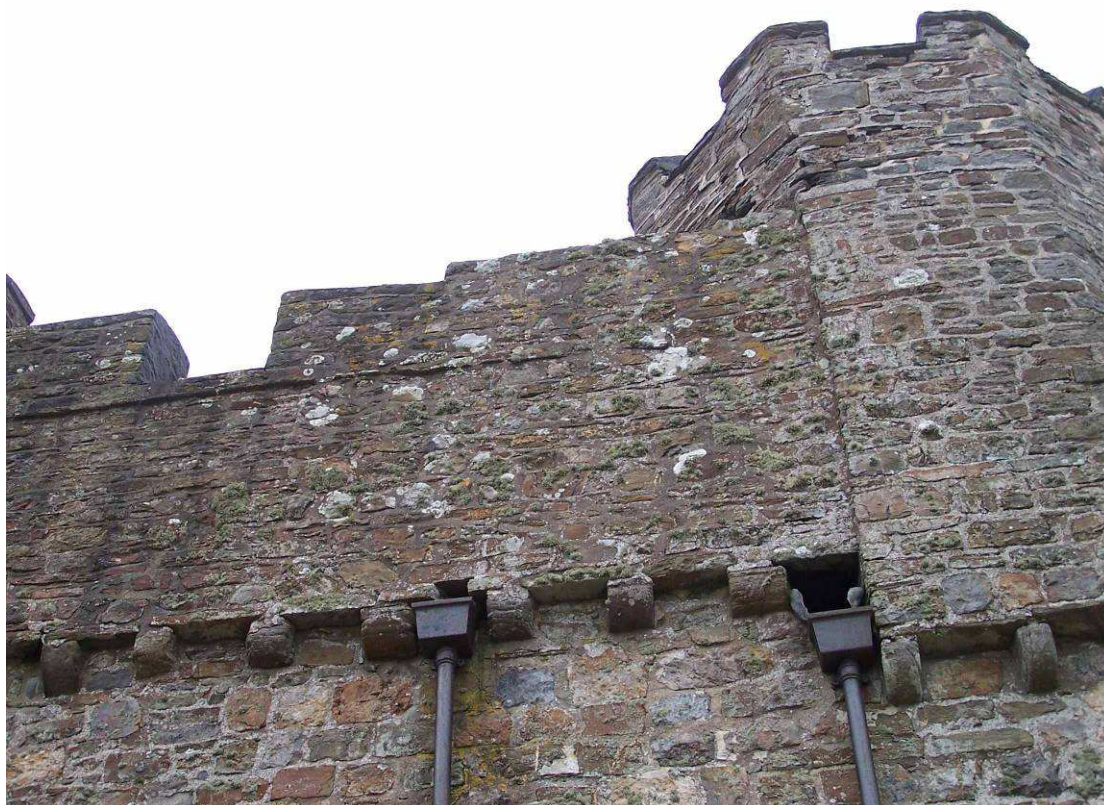
Photo 43: Western side of Northern elevation, showing Western Turret and corbel course
