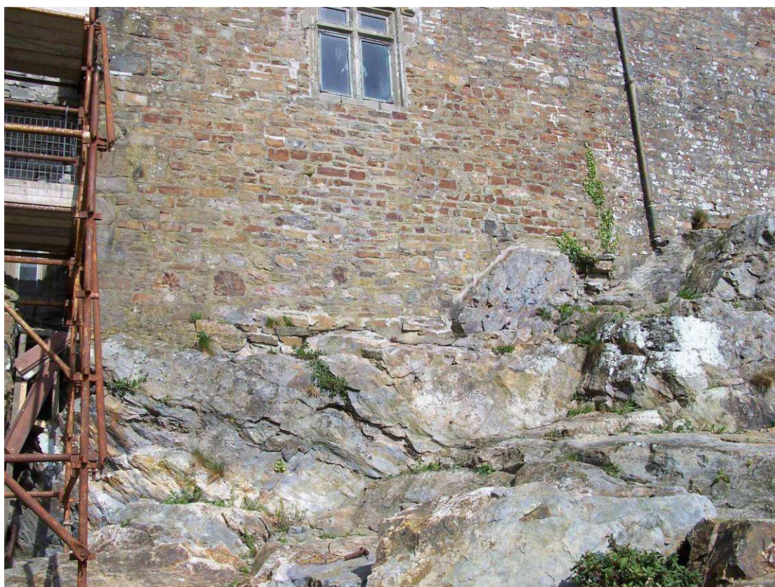
Photo 32: Lower part of western elevation built directly upon bedrock
