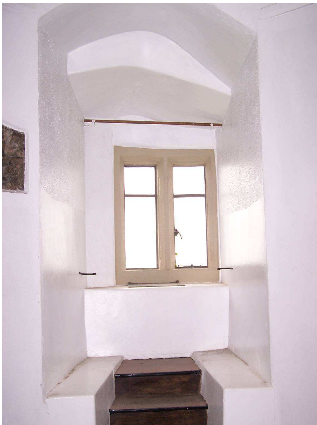
Photo 19: Window opening in southern part of west wall of Court Room (Room 3), an original medieval opening with modern window inserted
