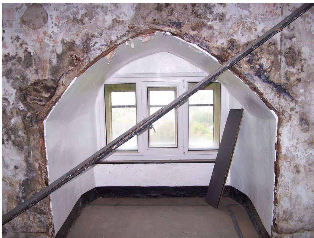
Photo 21: Arched window opening in west wall of Room 6, with stone voussoirs visible on left hand side of photograph above arch
