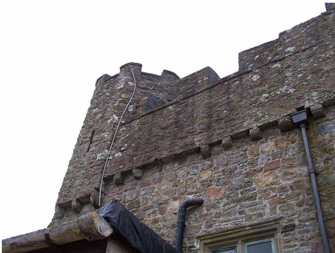
Photo 42: Eastern side of Northern elevation, showing Eastern Turret, part of central window and corbel course
