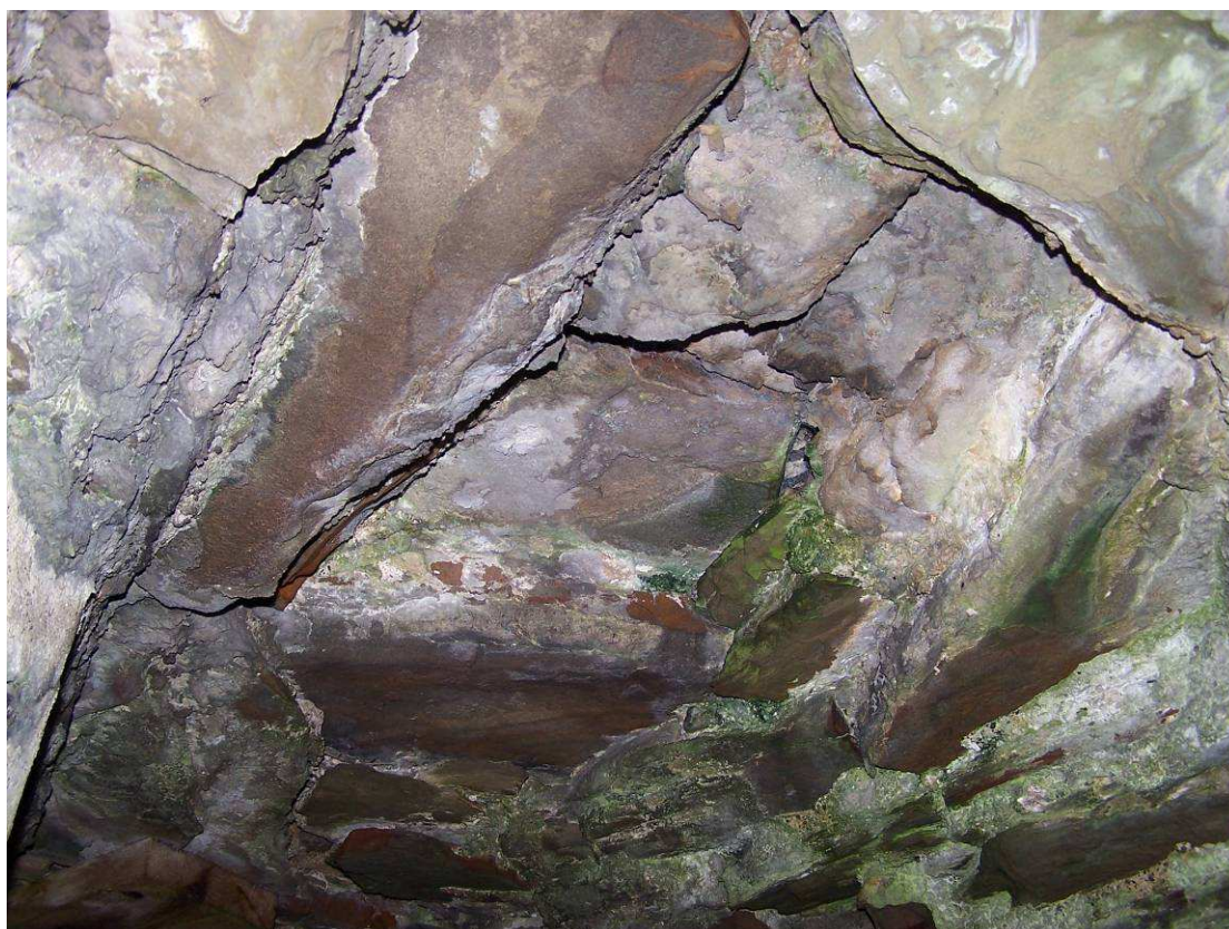
Photo 29: Underside of turret floor showing stone corbelling suggesting original medieval fabric
