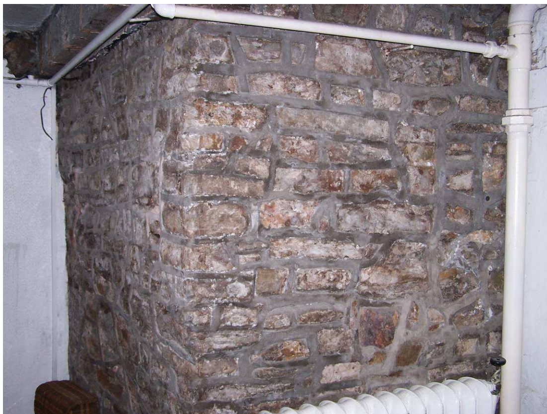
Photo 18: View of northern wall of Court Room (Room 3) showing exposed stonework, and modern breach on left hand side of photograph
