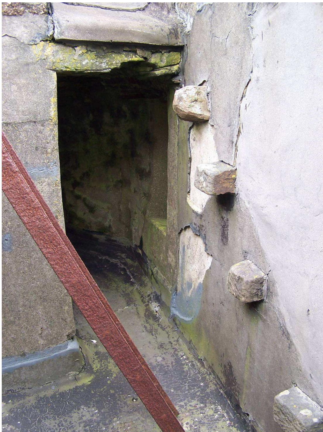
Photo 30: Projecting stones on the eastern side of the castle to carry steps to allow access to the turret floor.
