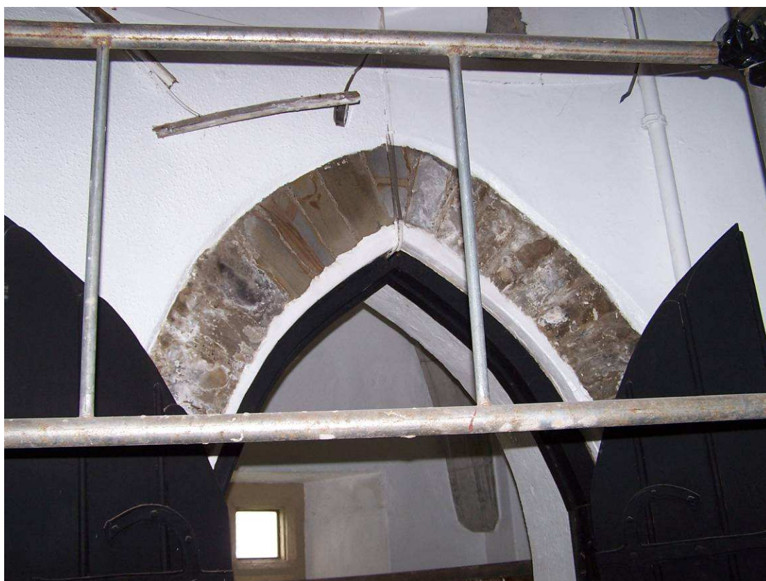
Photo 20: Arched doorway through to Room 5, with both original and replacement voussoirs, showing white imitation vaulted ceiling and modern sandstone ribs inside the room
