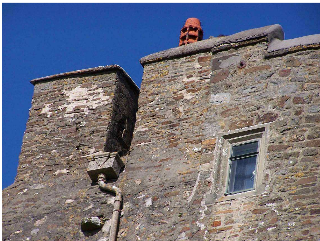
Photo 33: Evidence of Phases of Rebuilding in Crenellations
