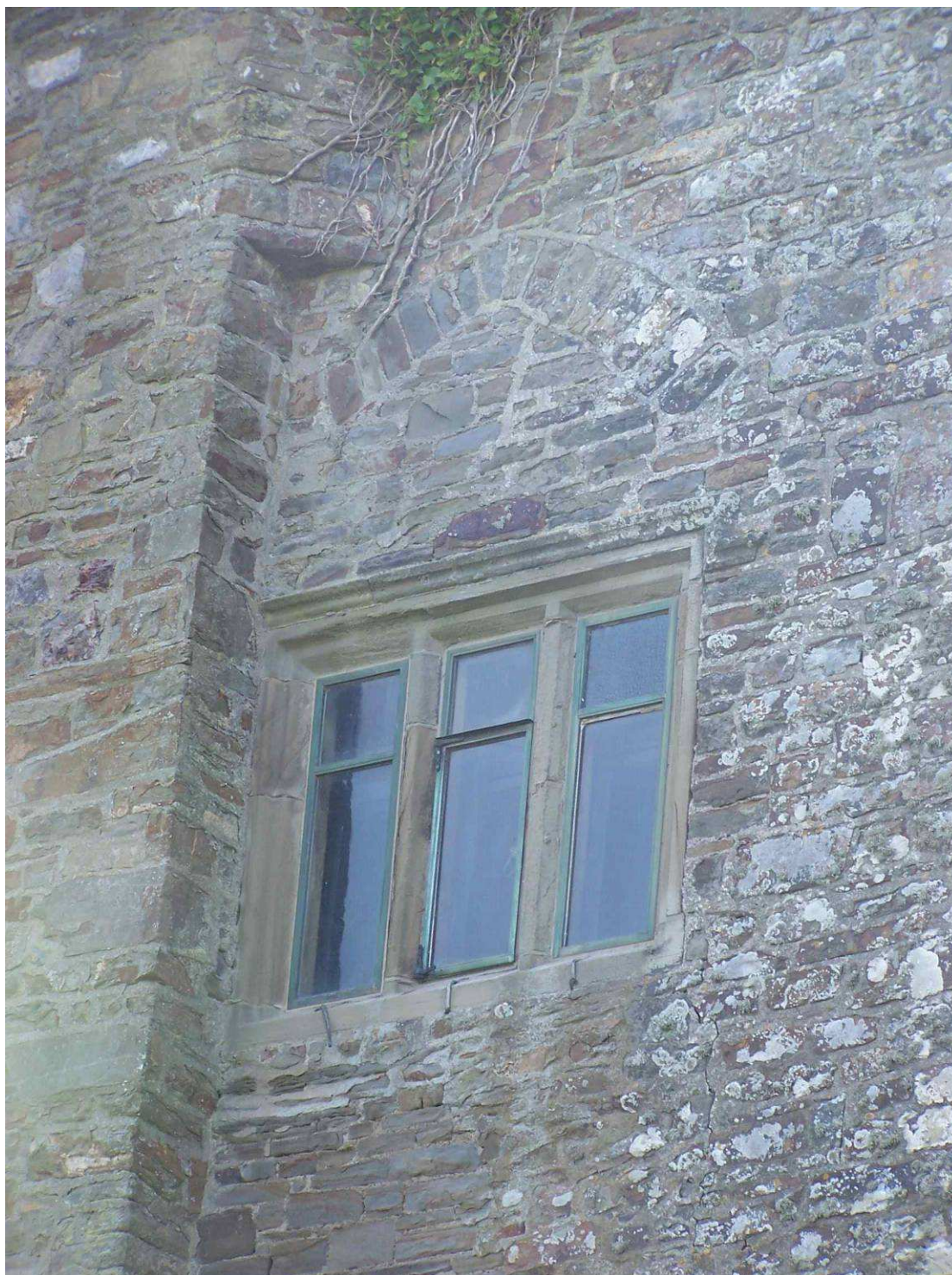
Photo 40: Former arch above replacement and rebuilt window in eastern façade
