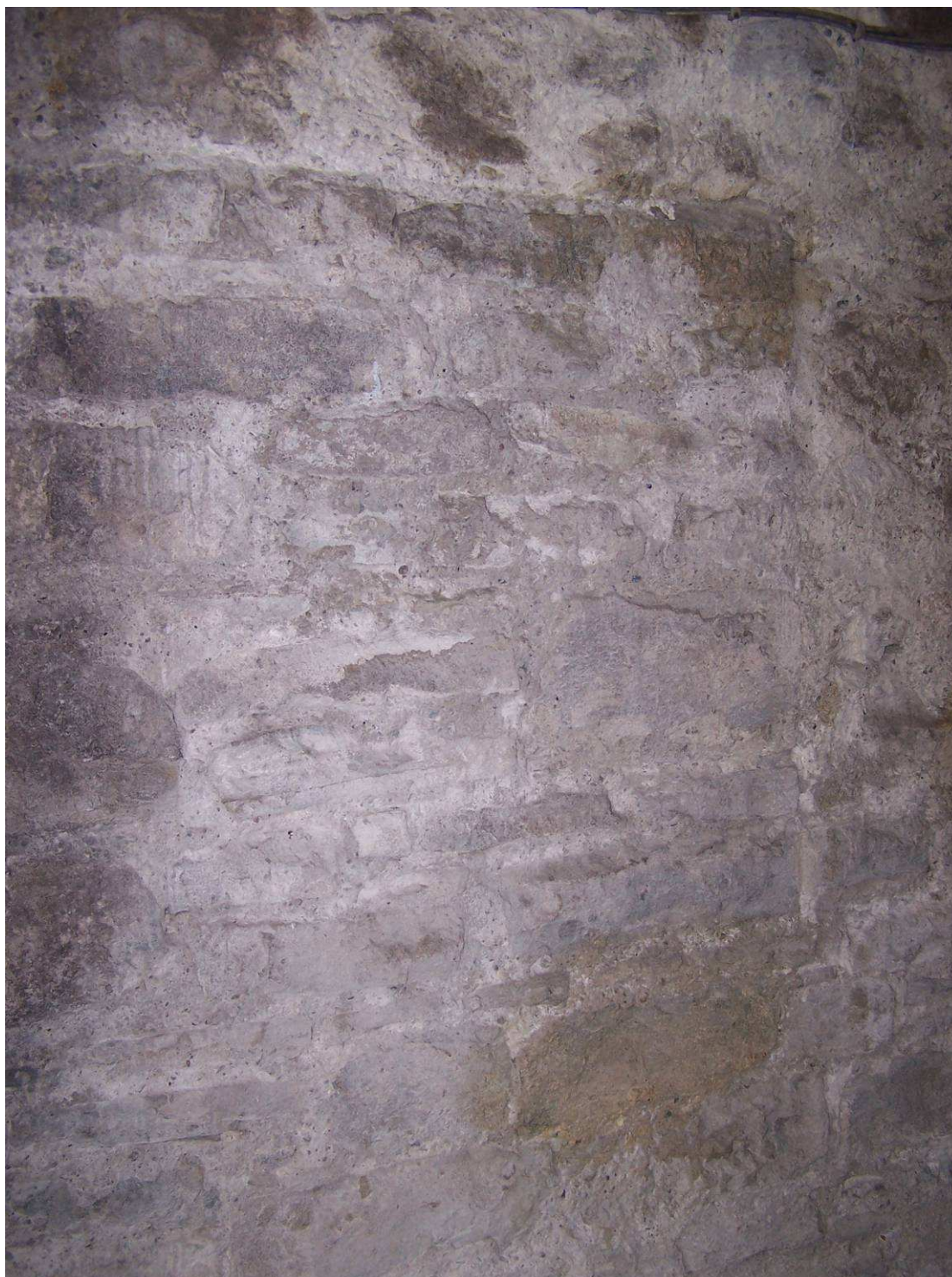
Photo 25: View of eastern wall above Room 10 (Garderobe) which shows infilled window or alcove as seen by straight joints in the stonework
