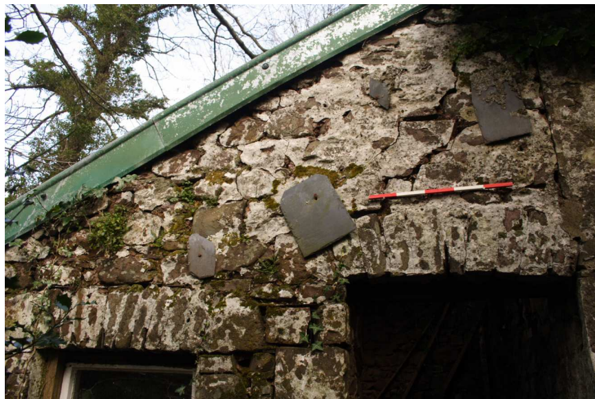
Photo 8 a & b: South facing external wall of addition, with remnant slate cladding
