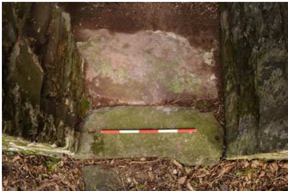
Photo 11: Threshold to addition. Stone slab with hinge or bolt sockets
