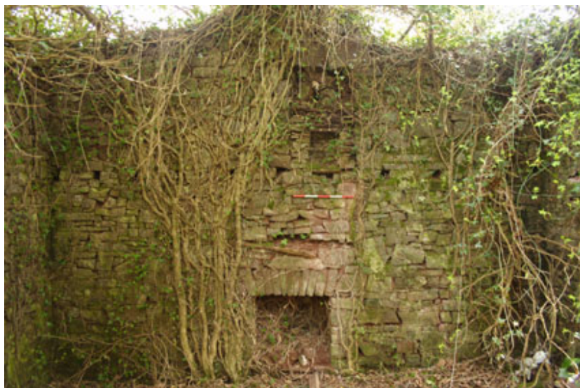
Photo 17: Ground and first floor fireplaces on east gable wall
