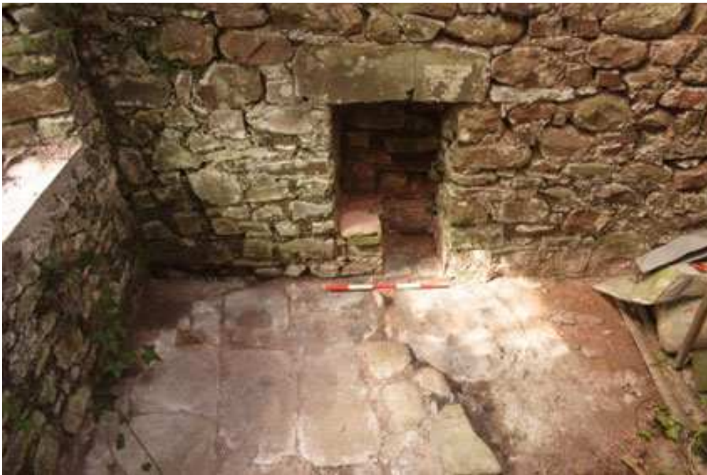
Photo 10: Fireplace and stone floor slabs in the addition
