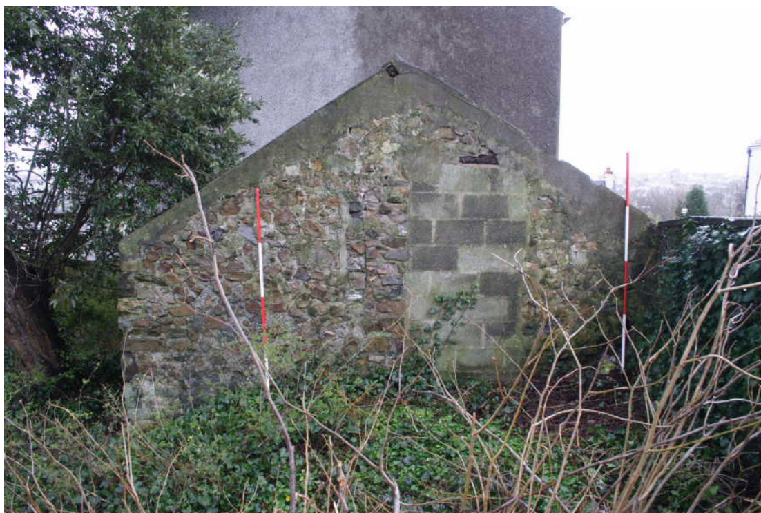
Photo 6: Gable end of 'garage' building at east end of wall (101) showing blocked original opening. View east (IMG_9937).
