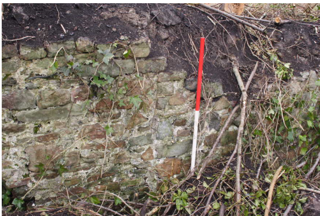
Photo 10: Wall (102), detail of butt joint c.0.3m left of 1m scale. View northwest (IMG_9941).
