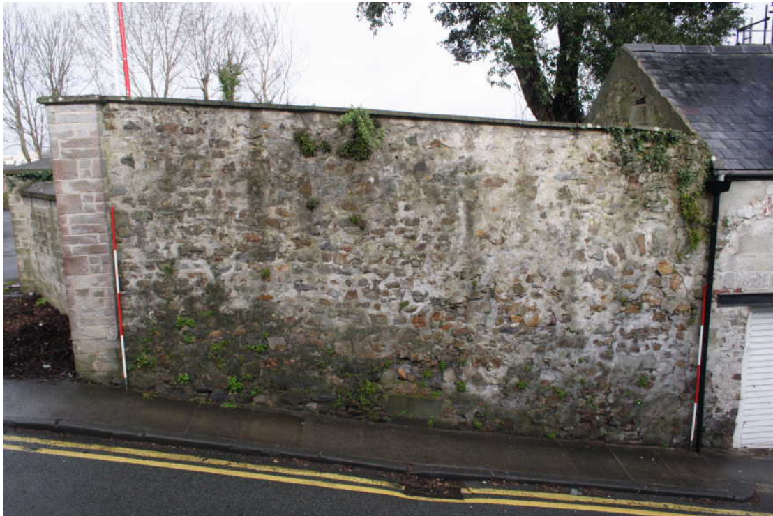
Photo 3: Wall (101), 2 x 2m scales. Note arch of blocked entrance just visible at east end of wall. View north (IMG_9932).
