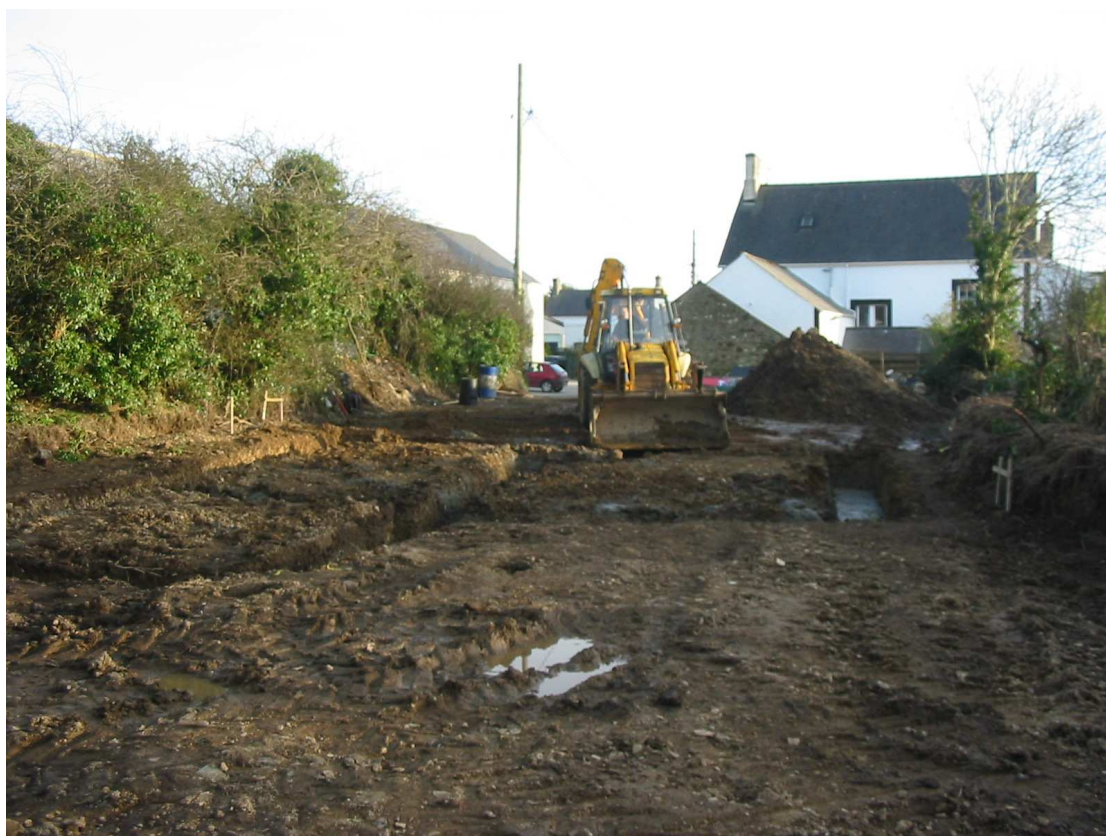
Photo 3: Footing trenches. View south.
