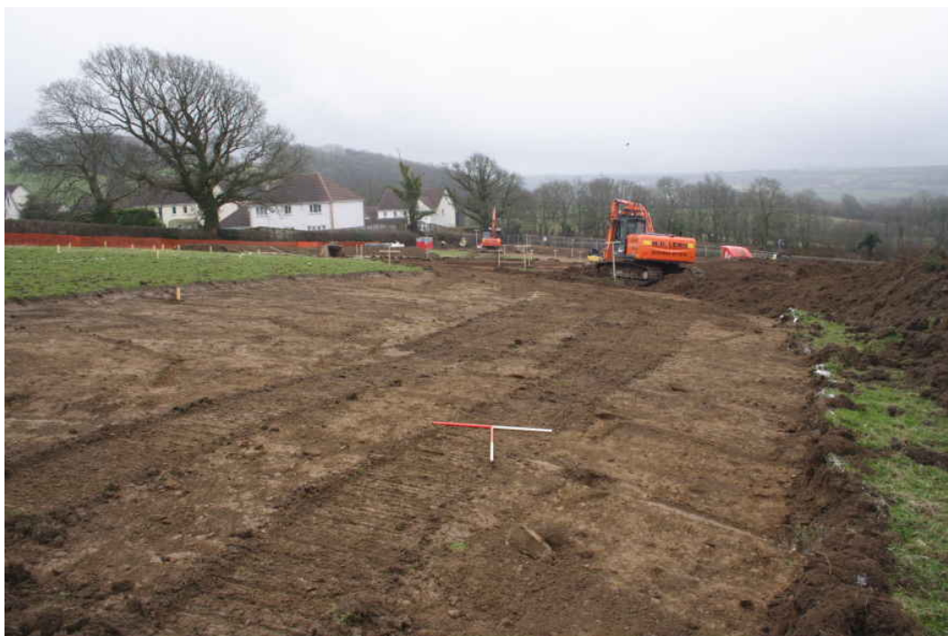
Photo 6: Site during topsoil stripping, facing SE.
