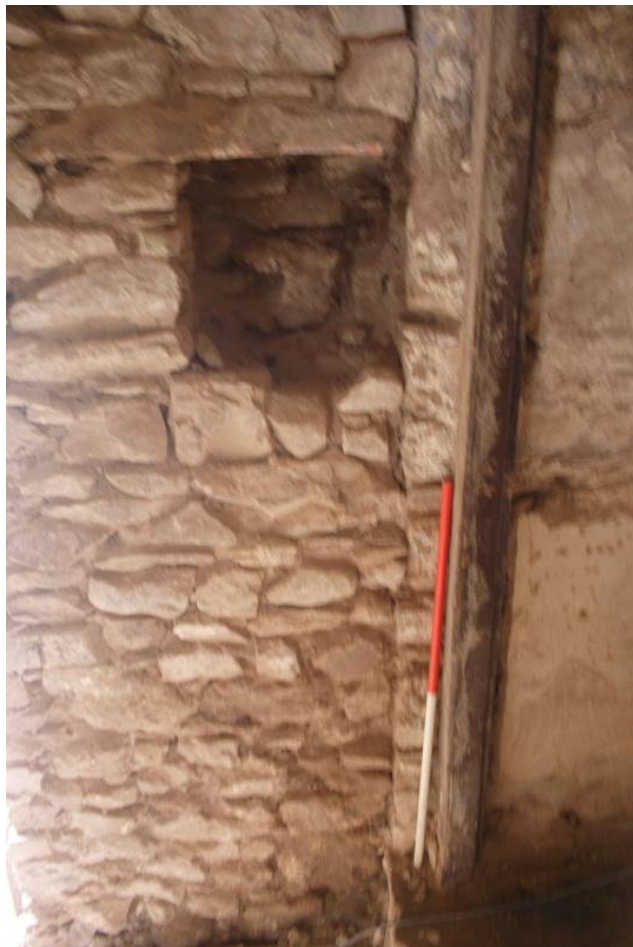
Photo 9: Straight joint in masonry with recess, Room 3
