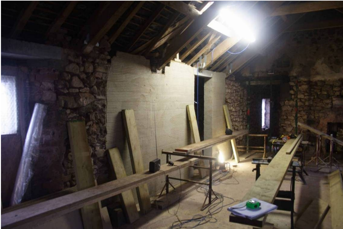
Photo 24: Lime rendered east wall, Room 11
