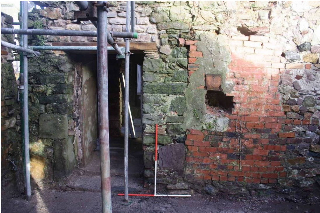
Photo 5: Brick infill and doorway, north wall room 2
