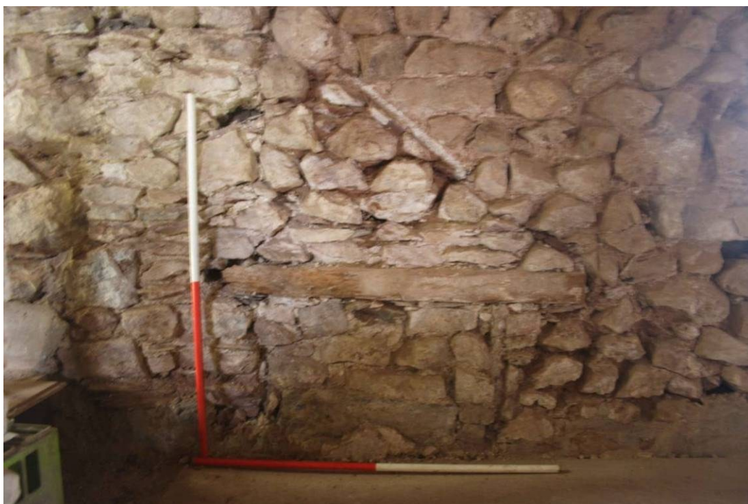
Photo 22: Detail of blocked window and former roof line, west wall Room 10
