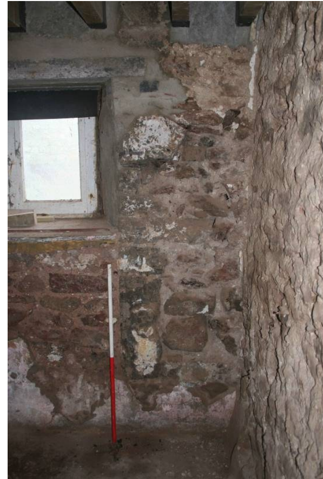
Photo 15: Possible straight joint in north wall, Room 7
