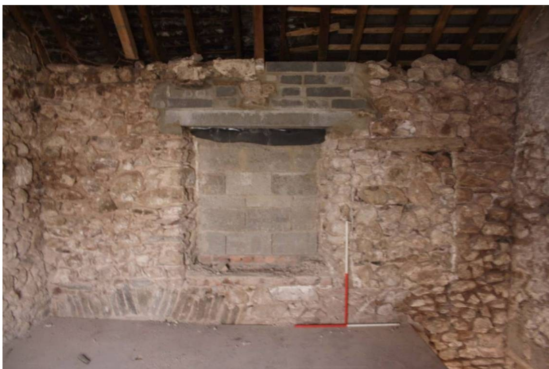
Photo 21: East wall Room 10 showing blocked windows and relieving arch
