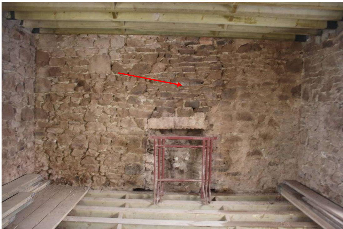
Photo 13: Fireplace, chimney reworking highlighted by arrow, north wall Room 5
