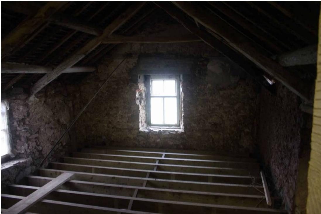
Photo 29: Four paned sash window, east wall Room 13
