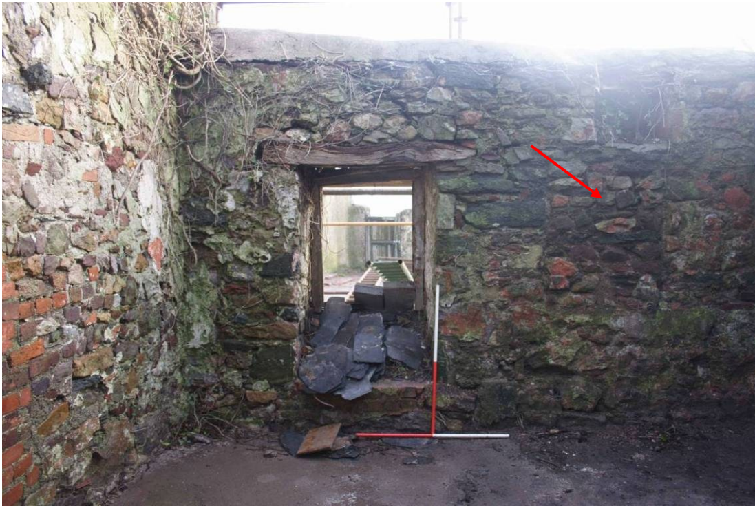
Photo 4: Window in east wall Room 2, blocked opening highlighted with arrow
