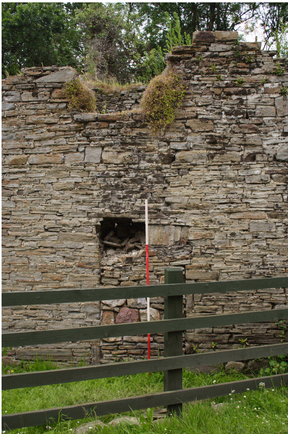
Plate 38: Extension gable end from southwest showing blocked doorway with window above. Shot 3.
