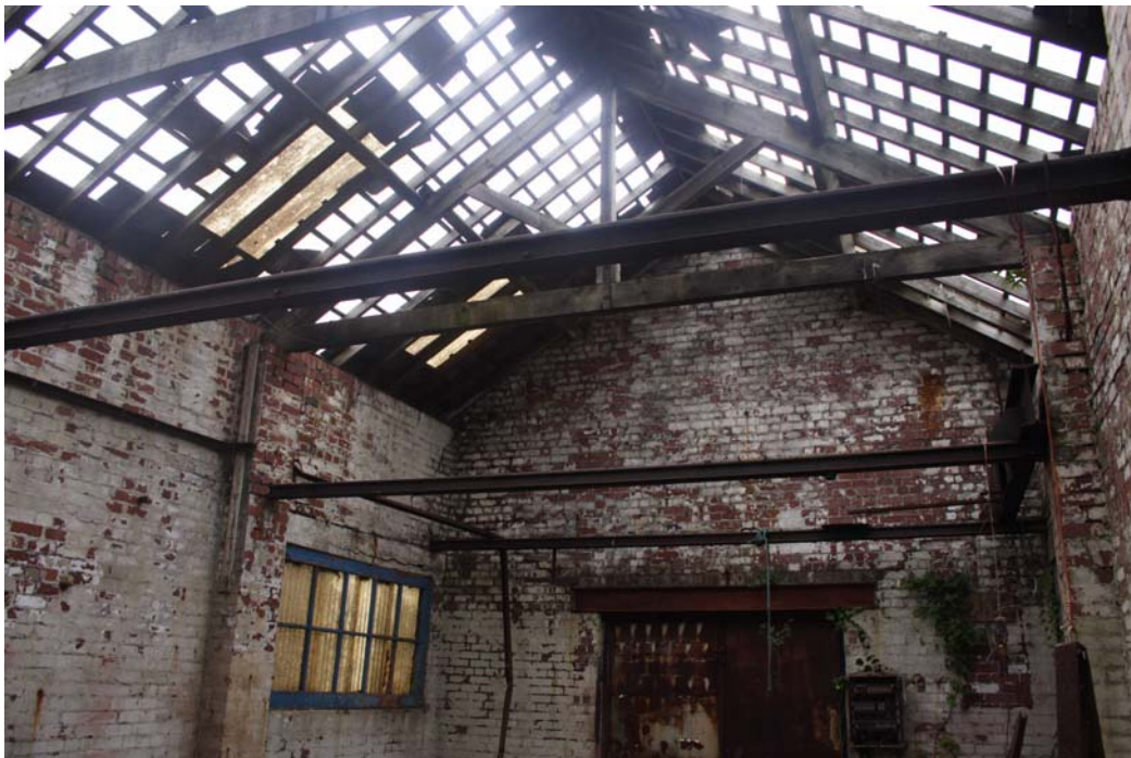
3990: Brick addition. Railway lines reused as cross beams
