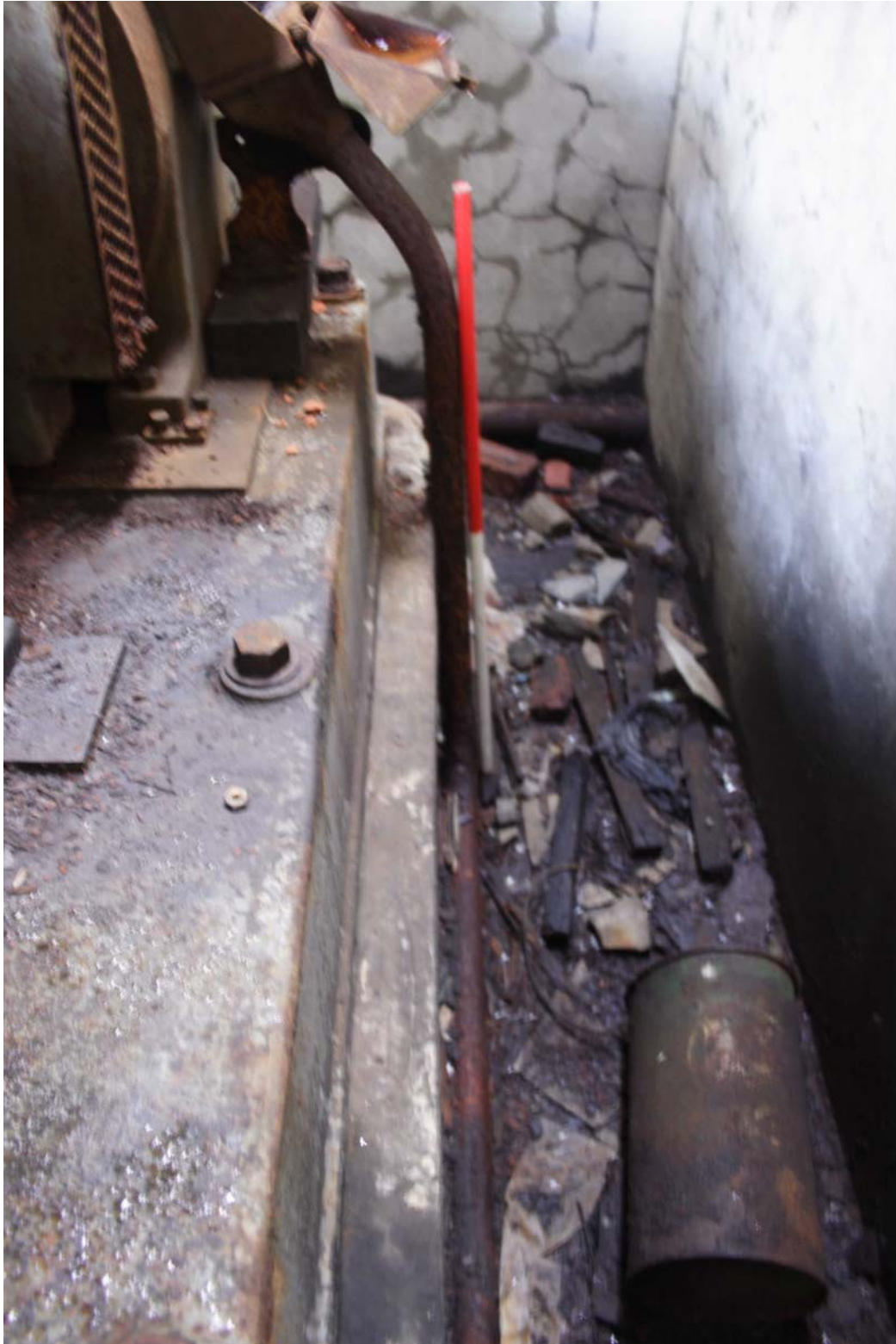
3911: Later pump room. Pump 2 cable duct attached to junction box
