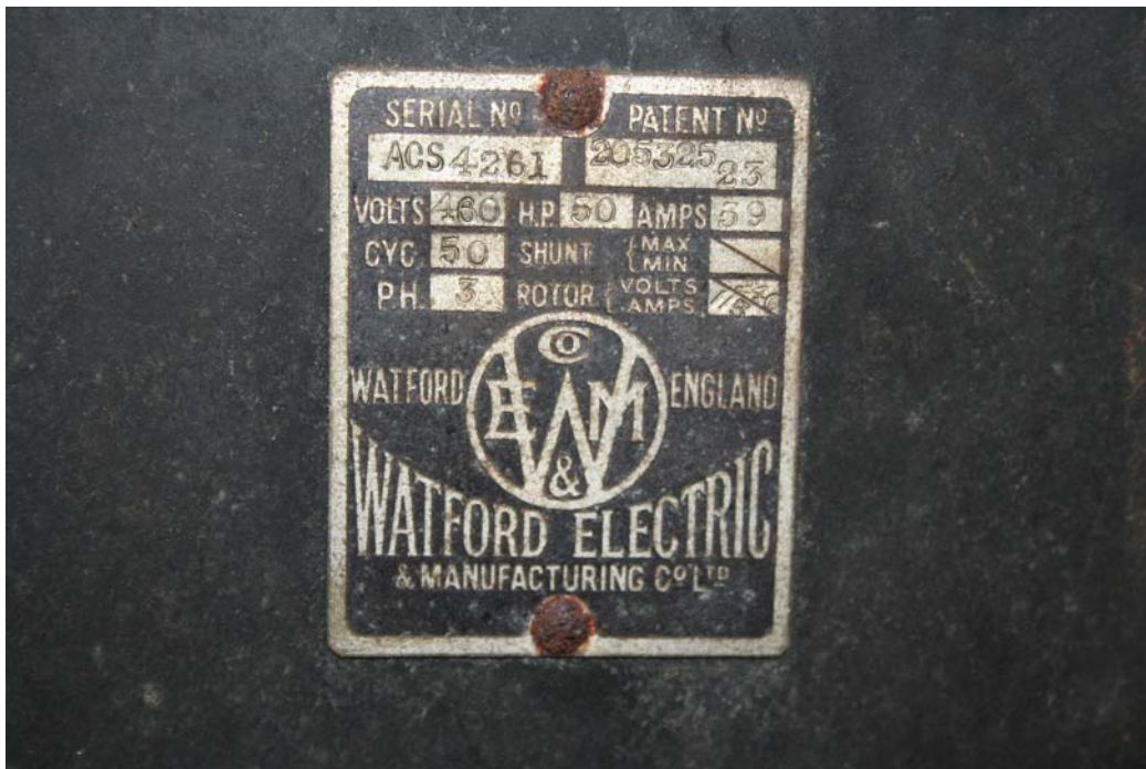
3916: Later pump room. Pump 2 switch box Watford Electric makers plate
