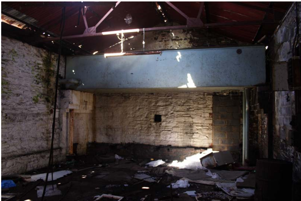
Plate 3946: Engine house. Cast iron water tank
