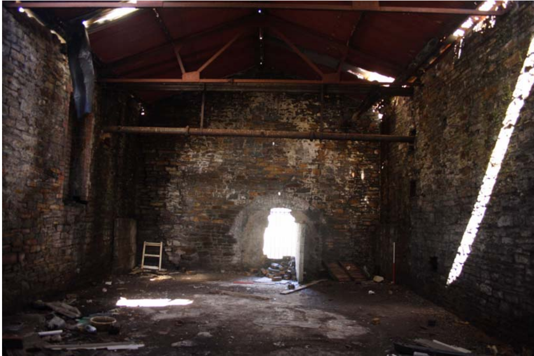
3938: Boiler house. Gable end with arched opening to site of chimney
