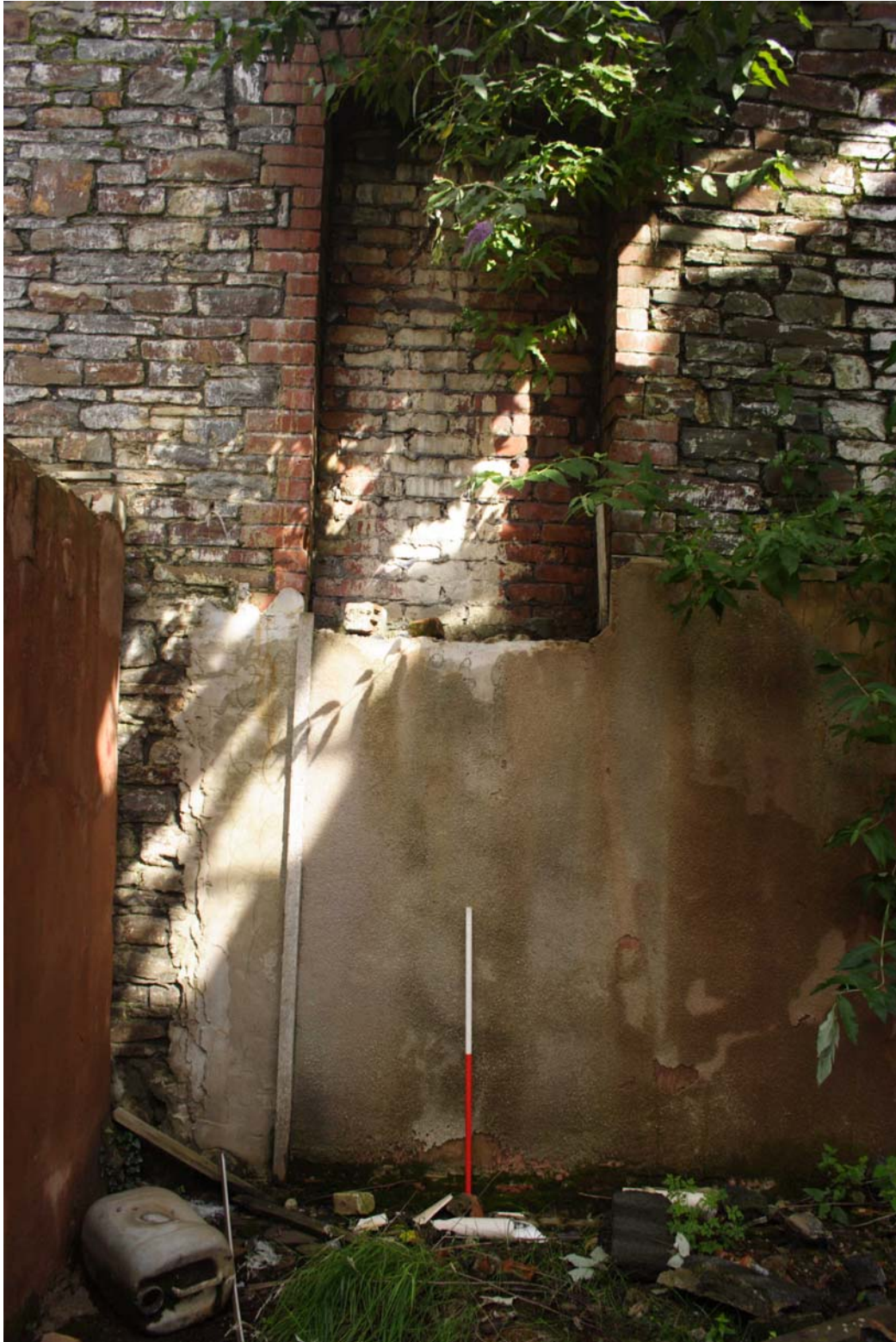
4005: Maintenance shed. Blocked southernmost window to boiler house
