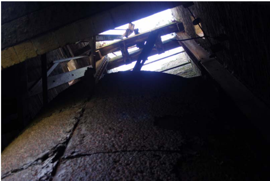
3957: Accumulator tower. Guide rails and frame to hold weight. Collapsed cylinder below
