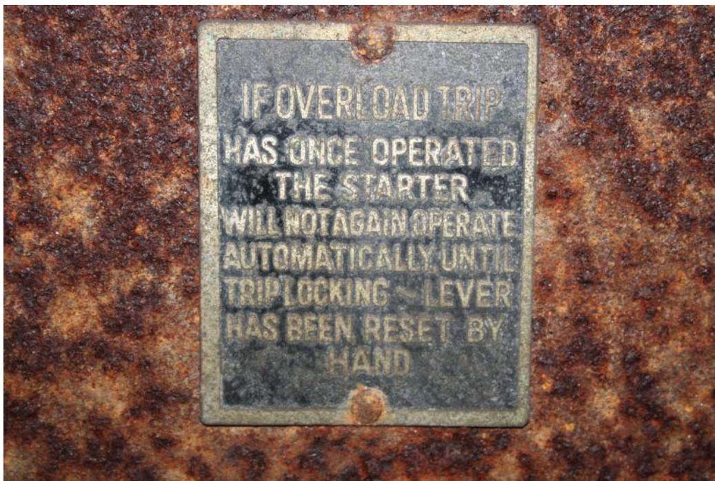
3918: Later pump room. Pump 2 switch box overload trip plate
