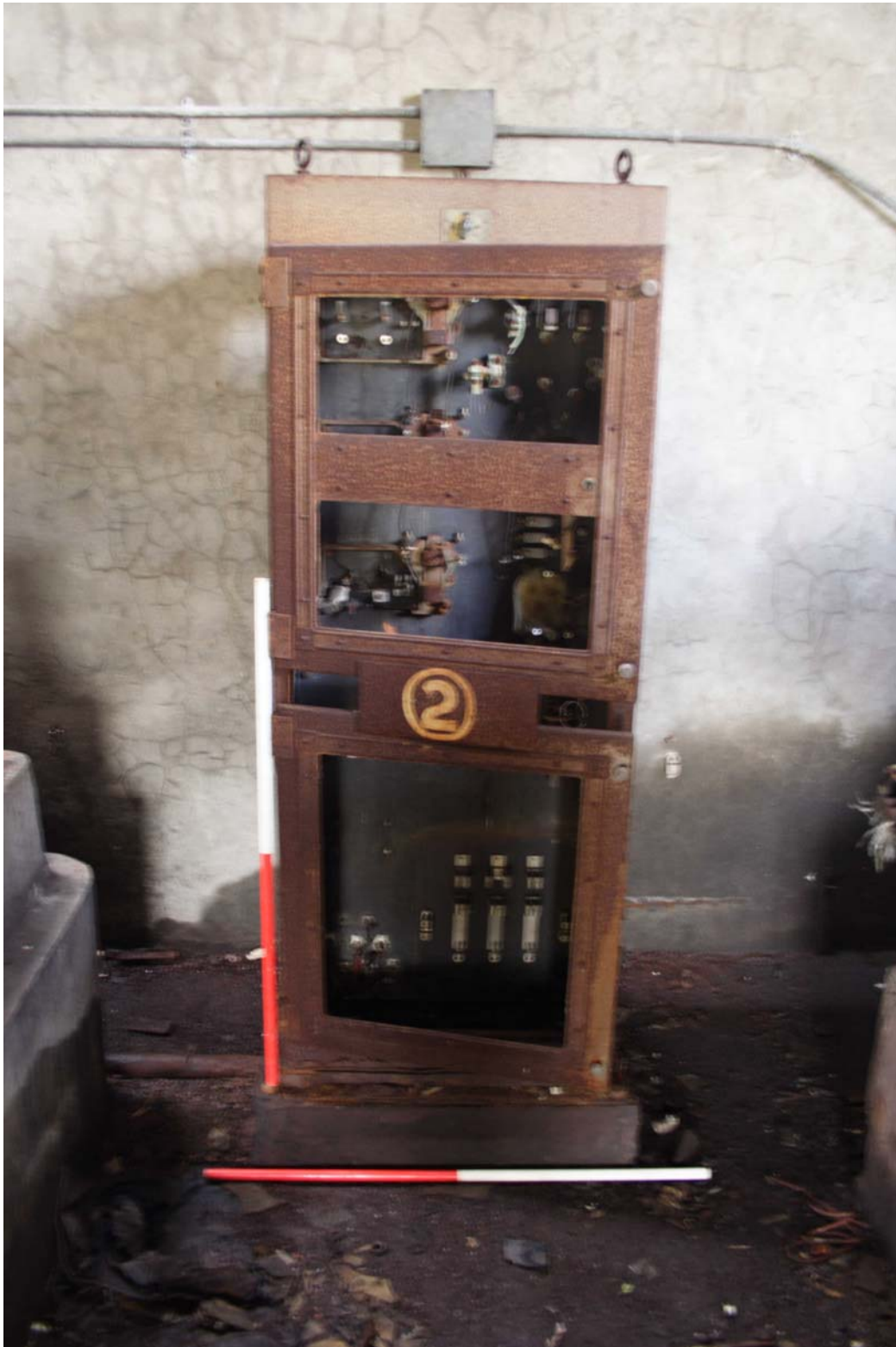
3912: Later pump room. Pump 2 switch box door closed
