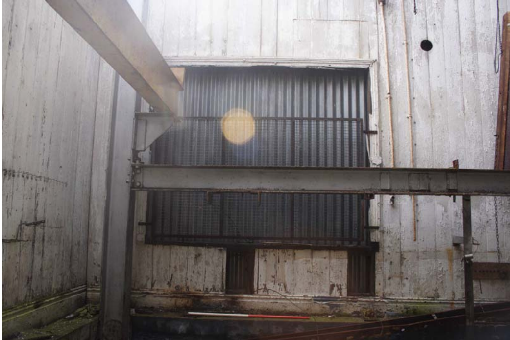
3967: Metal shed. Blocked window and original timber lining.
