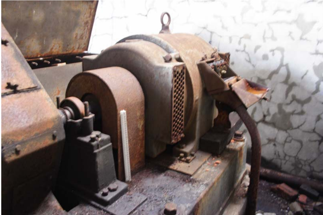
3908: Later pump room. Pump 2 motor/ dynamo
