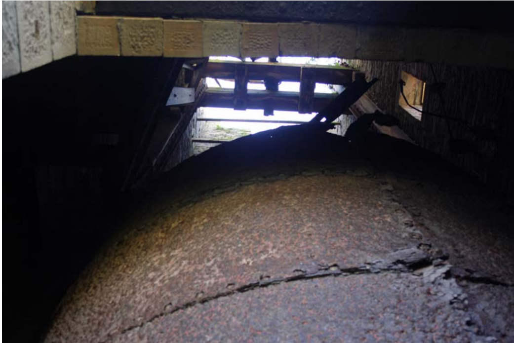
3956: Accumulator tower. Guide rails and frame to hold weight. Collapsed cylinder below
