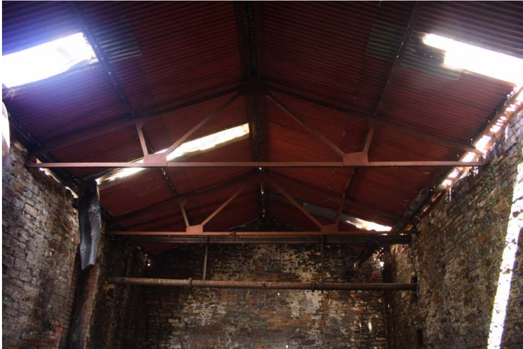
3941: Boiler house. Corrugated iron and steel roof
