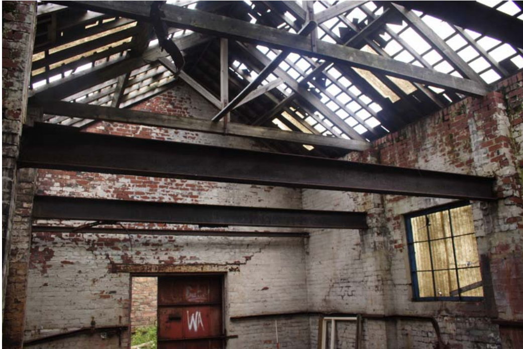
3989: Brick addition. RSJ cross beam.
