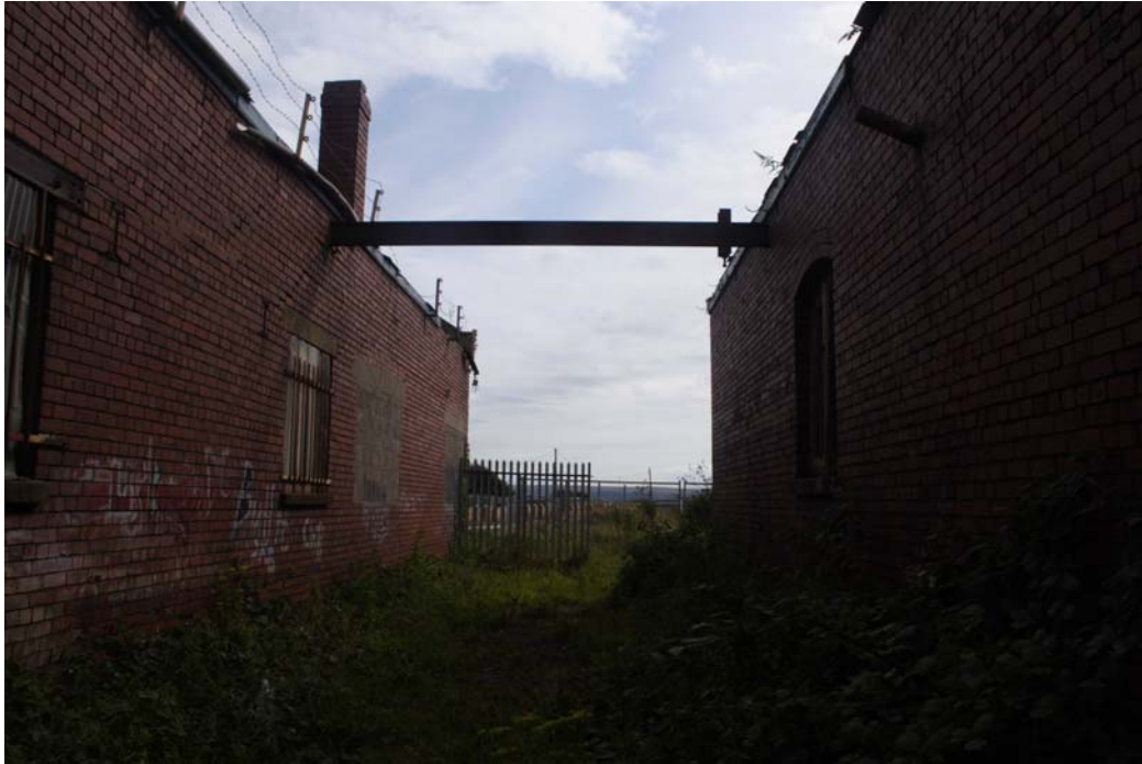
4011: Former hoist between brick maintenance shed addition and brick addition
