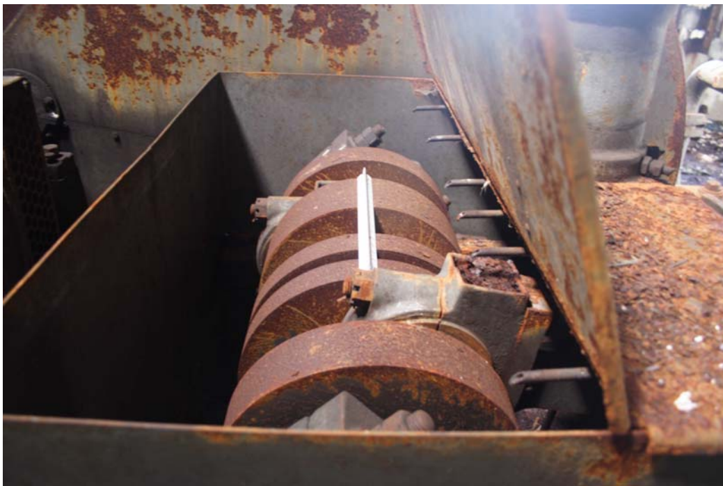
3907: Later pump room. Pump 2 crankshaft and case
