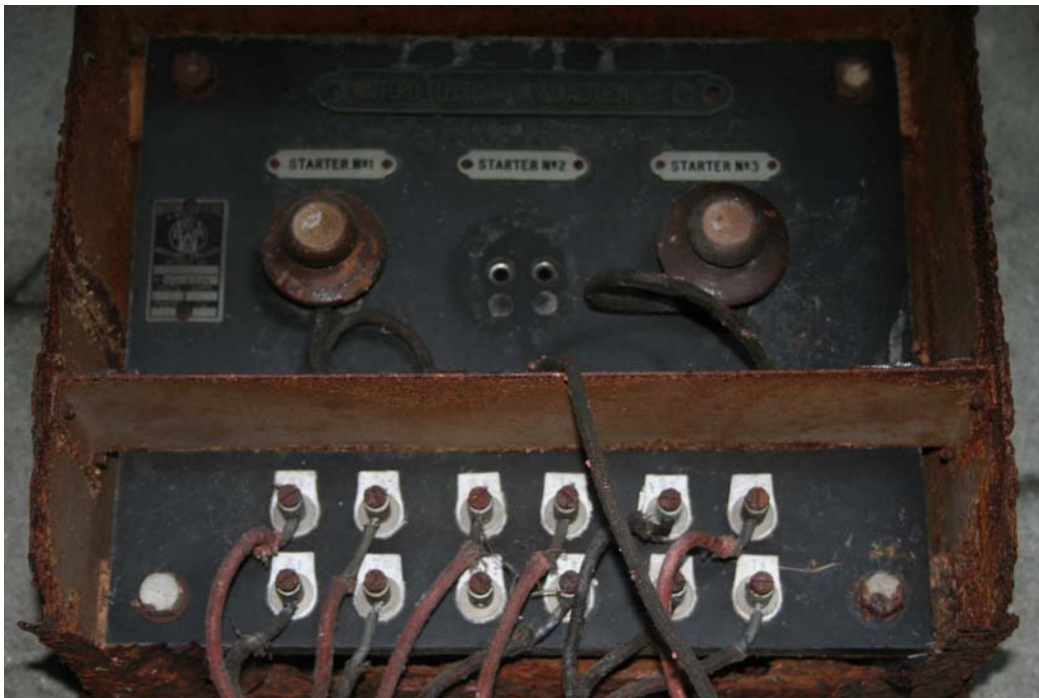
3926: Later pump room. Pump starter box close up
