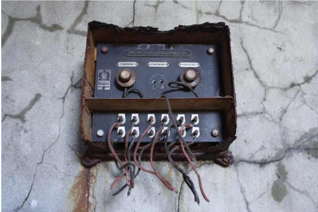
3925: Later pump room. Pump starter box
