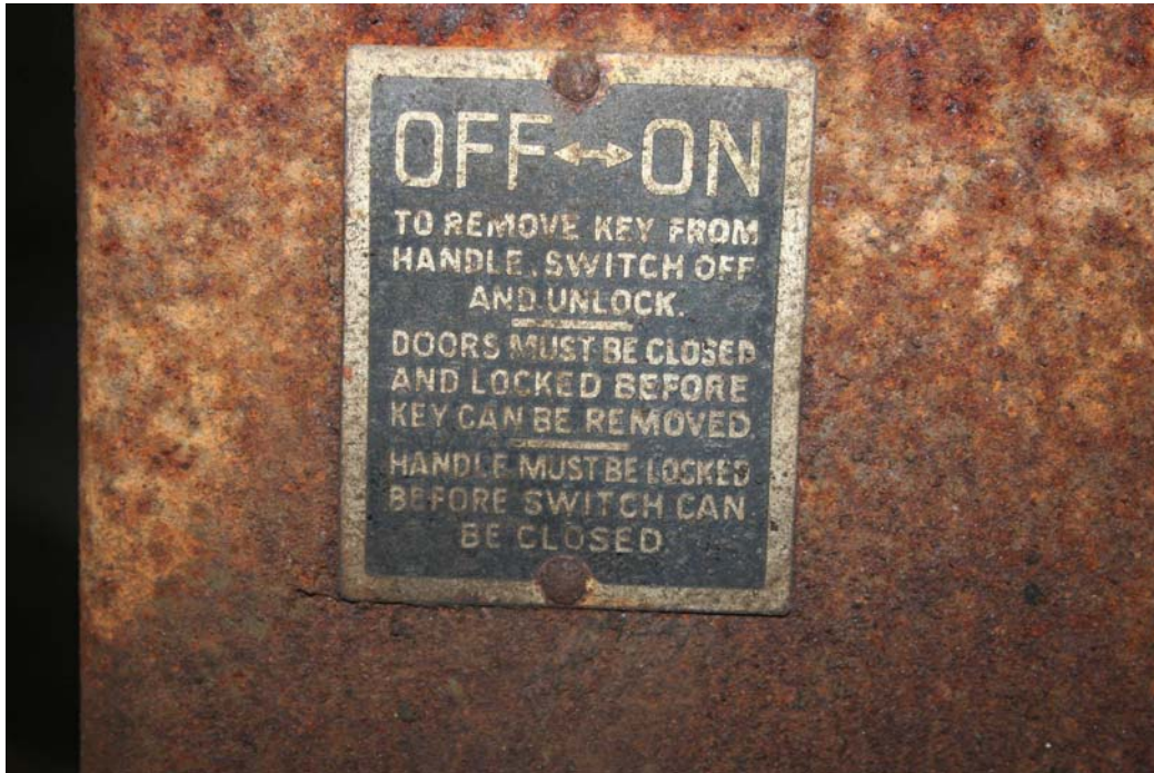
3919: Later pump room. Pump 2 switch box switch plate
