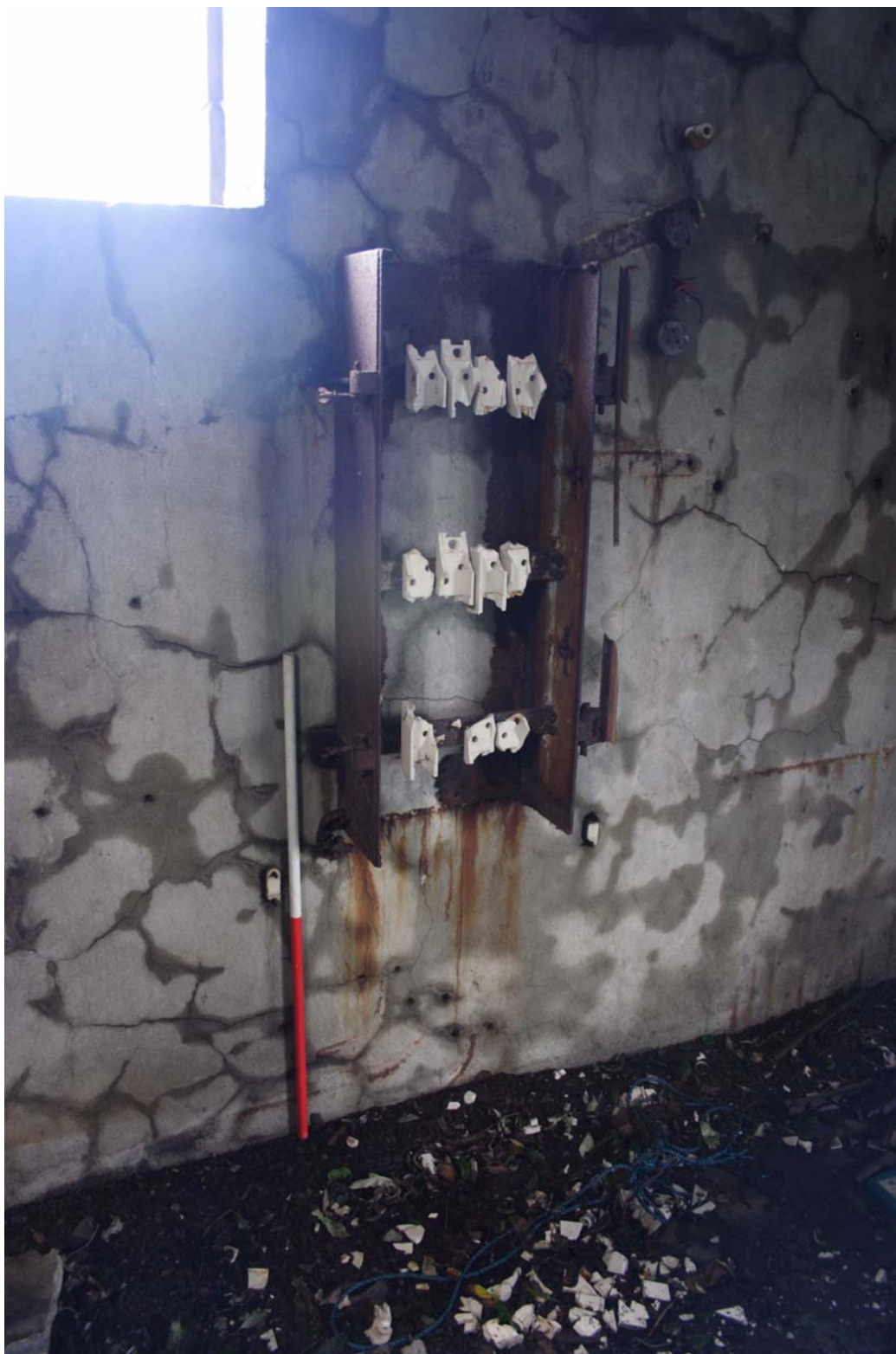
3930: Later pump room. Fuse box with remains of stoneware fuse mountings
