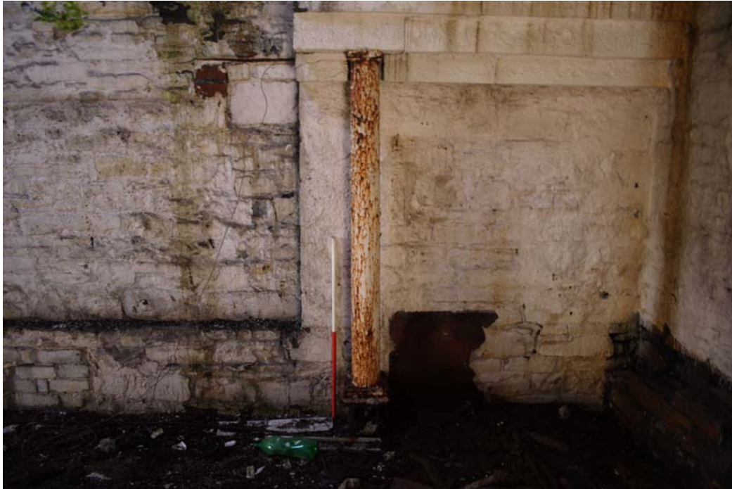
3947: Engine house. Cast iron supporting column beneath water tank
