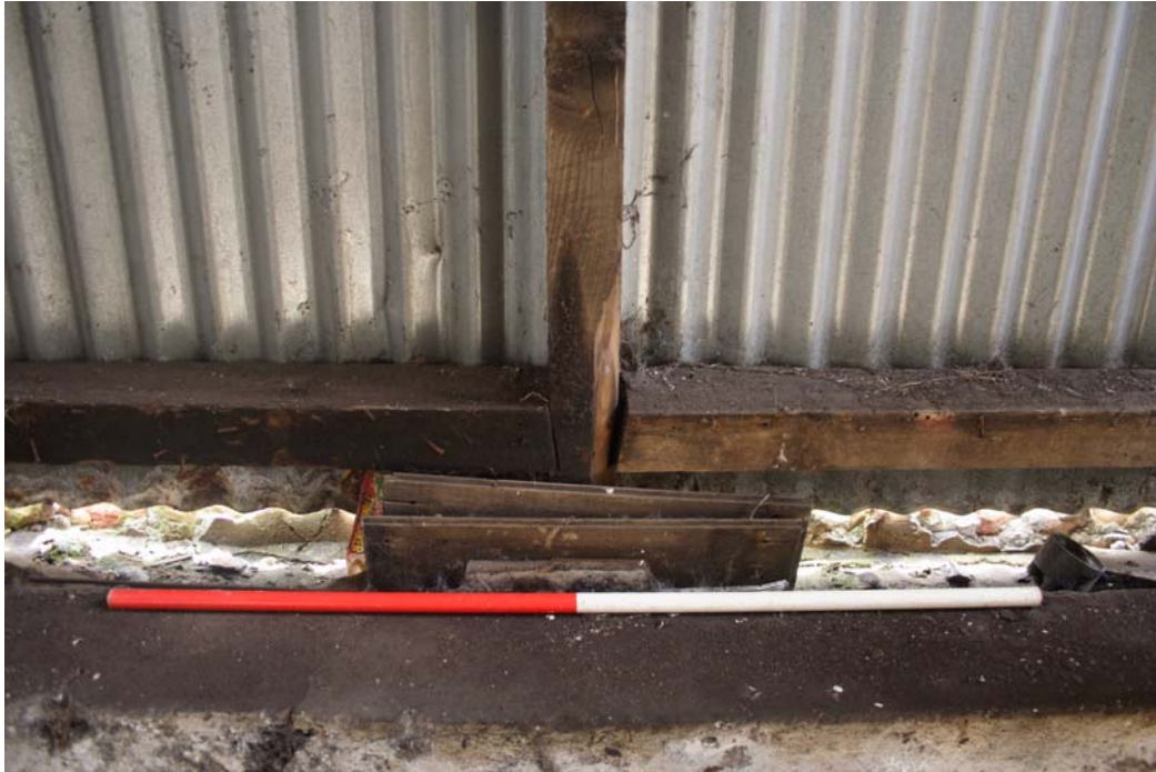
3969: Metal shed. Detail of timber frame joint
