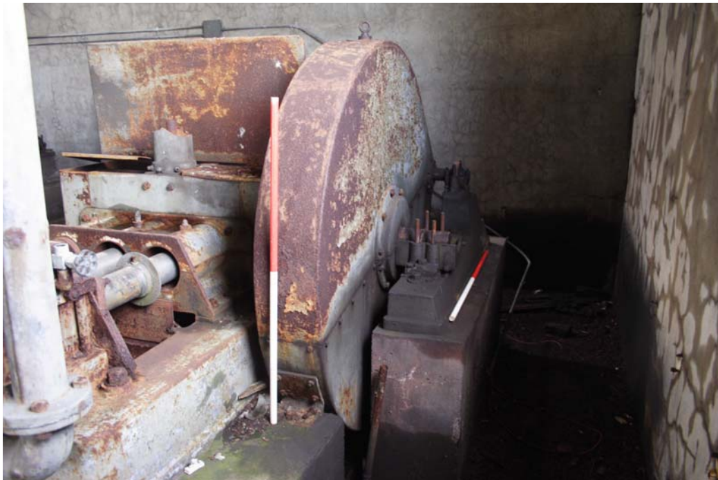
3896: Later pump room. Pump 1 gearwheel
