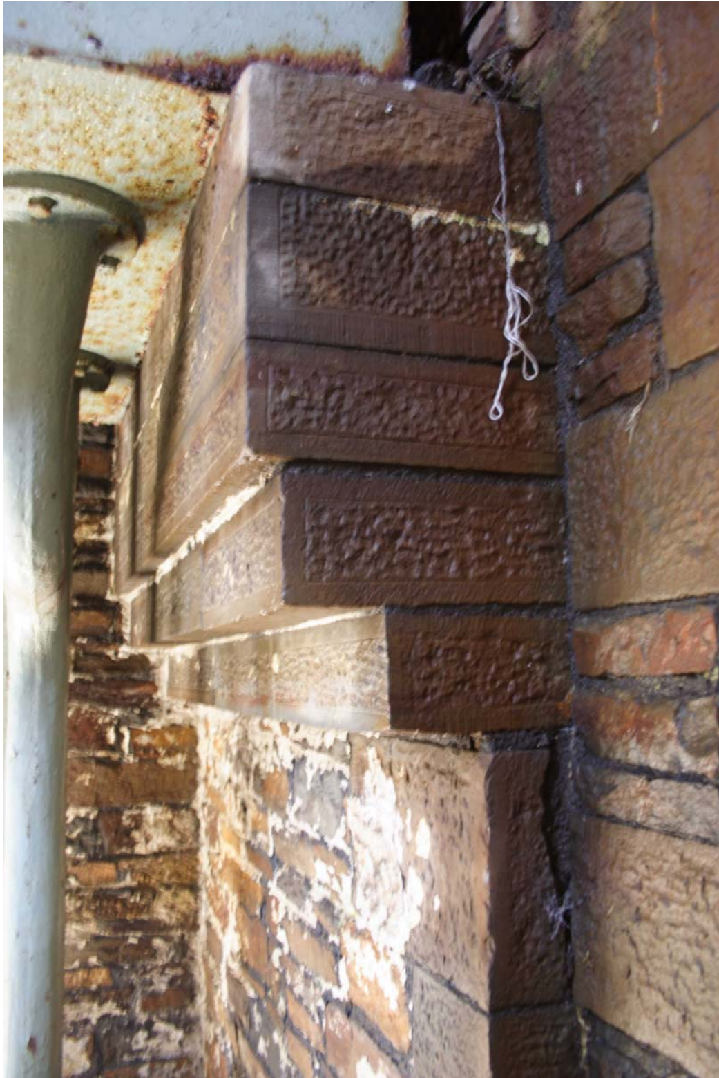
3949: Engine house. Dressed sandstone corbelling beneath water tank
