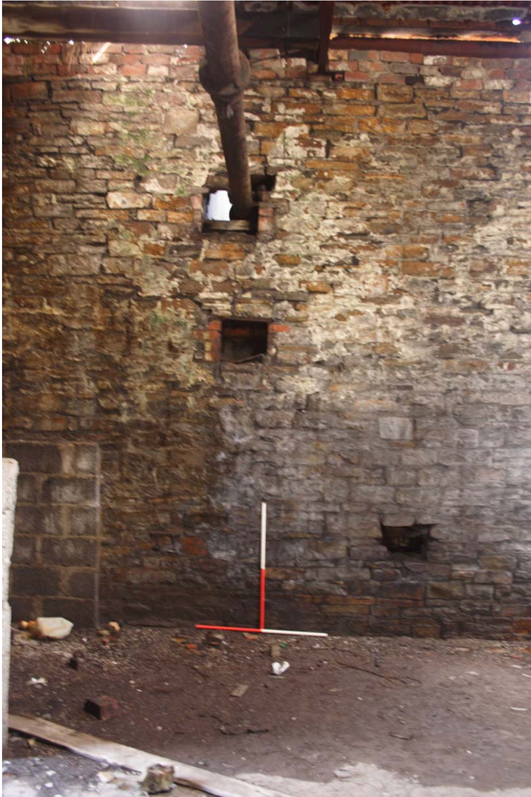
3940: Boiler house. Openings in wall. Uppermost carrying pipe from later pump room
