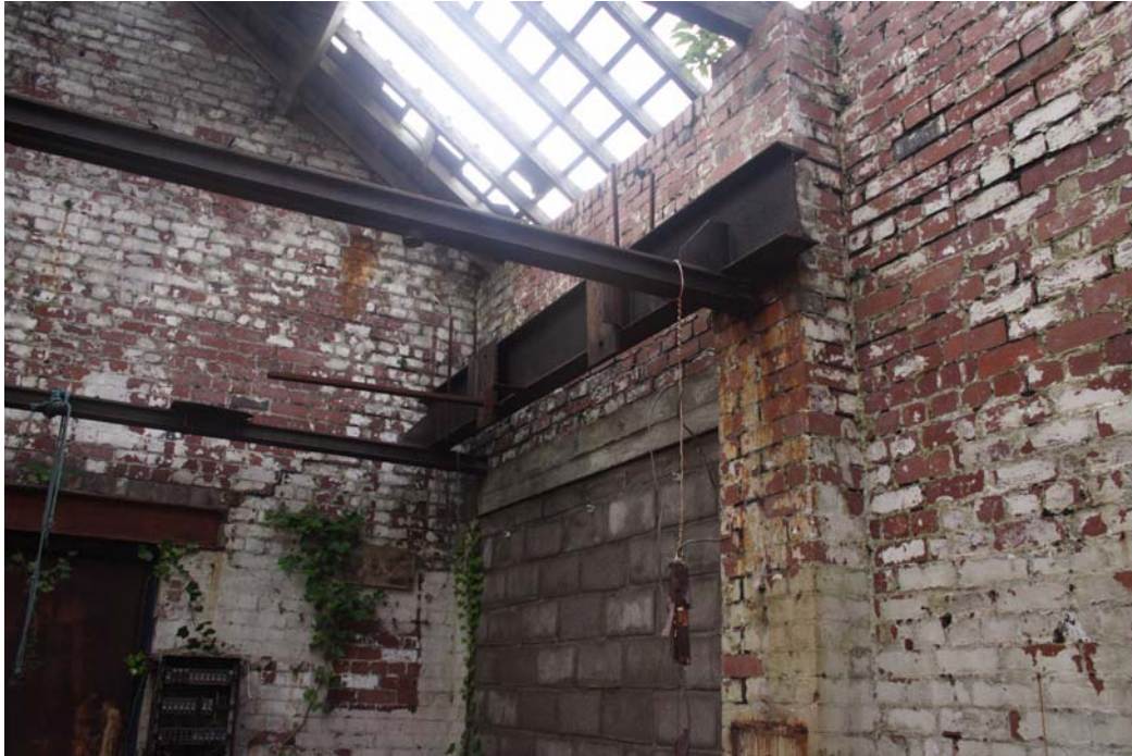
3983: Brick addition. Railway line reused as cross beam
