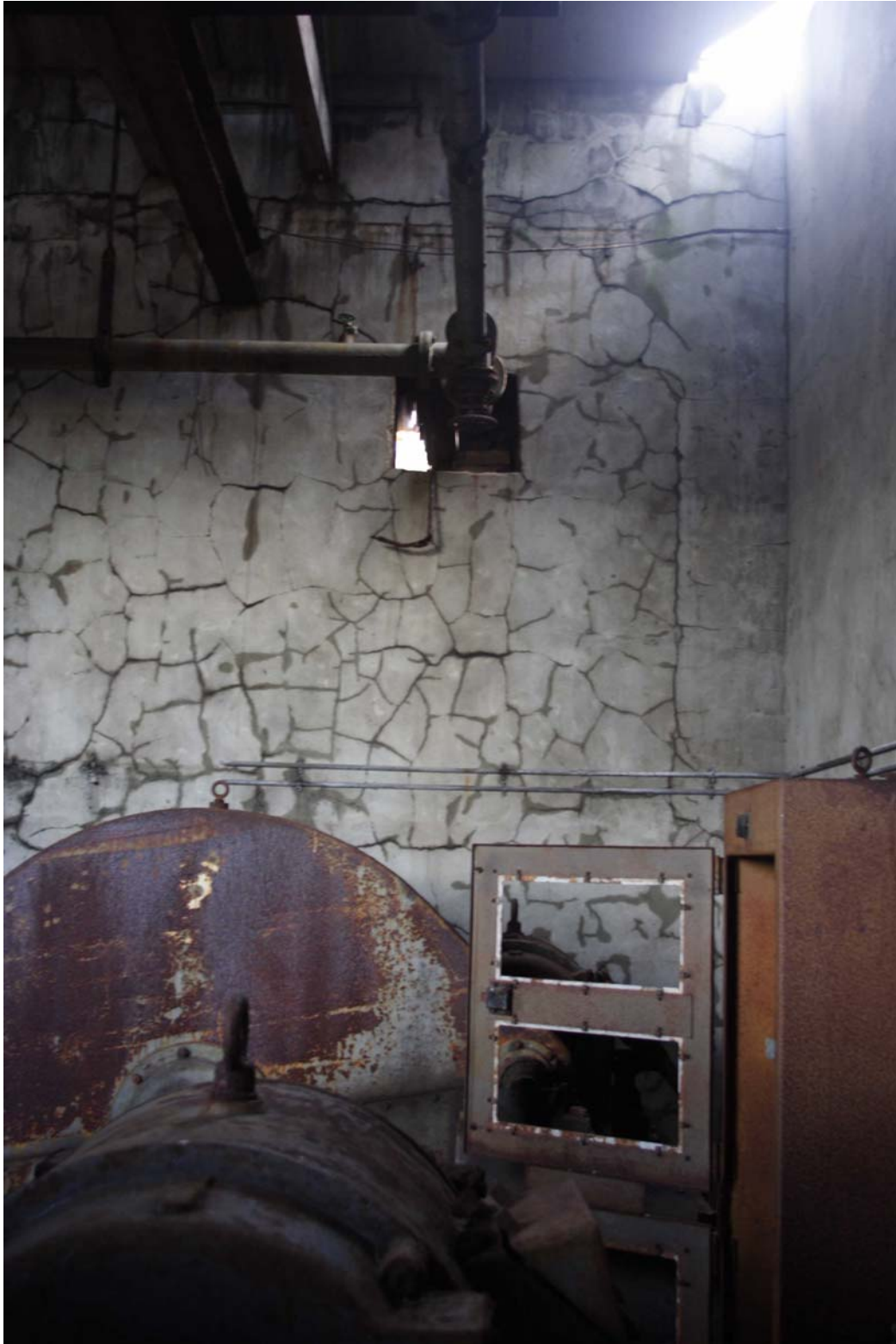
3922: Later pump room. Opening in wall carrying cast iron pipe to boiler house
