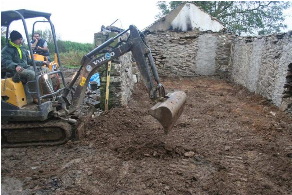
Photo 2. Cleaning the natural natural soil within the building after removal of the concrete floor. View south.
