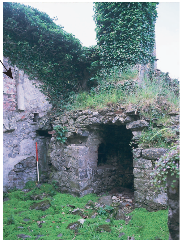
Plate 23: Bread oven and fireplace in tower
