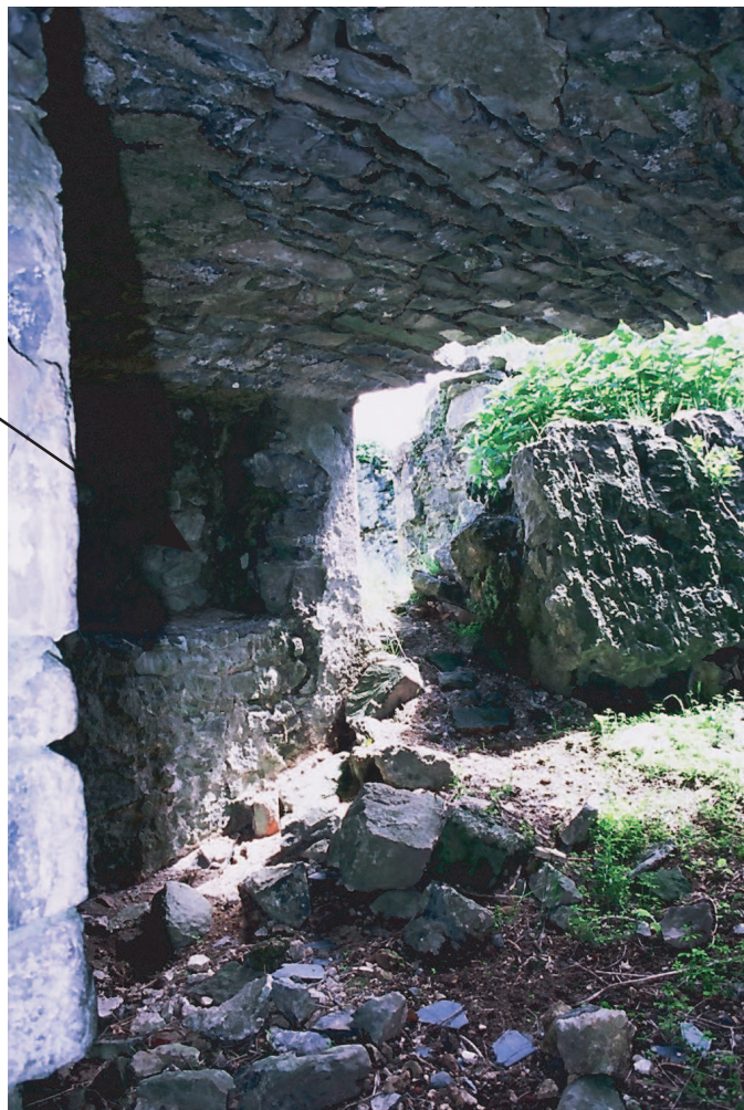
Plate 7: Southeast service room showing collapsed vault Wessex Archaeology
