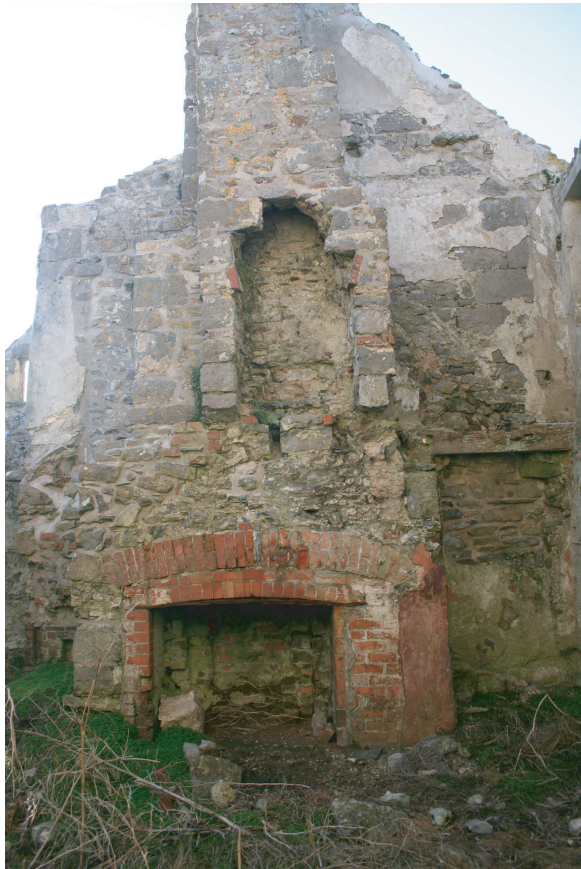
Plate 20: Northwest wall of the kitchen showing fireplace and chimney inserted into tower Wessex Archaeology
