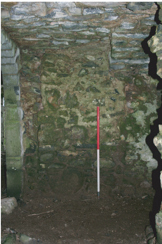
Plate 5: Blocked opening between the service rooms
