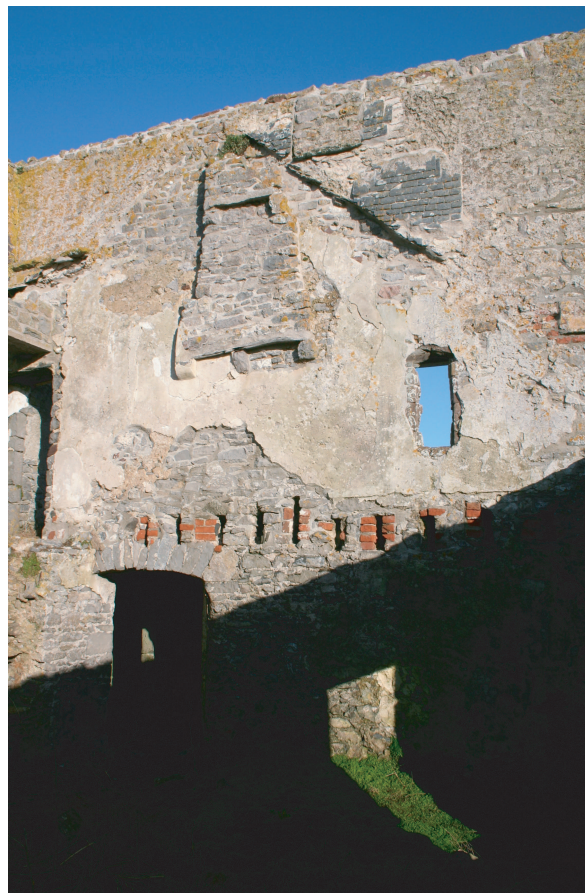
Plate 16: Exterior of northwest wall of the solar showing corbelled chimney
