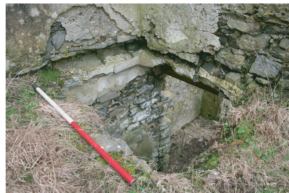
Plate 19: Break in floor of solar above cross passage
