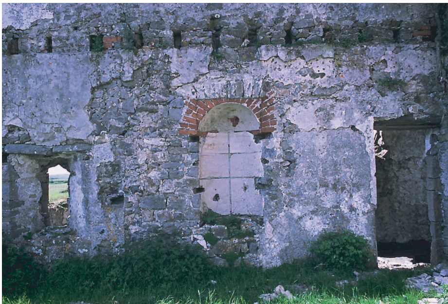
Plate 15: Northwest wall of the solar showing trefoil headed window and semi-circular niche - corbelled chimney behind Wessex Archaeology
