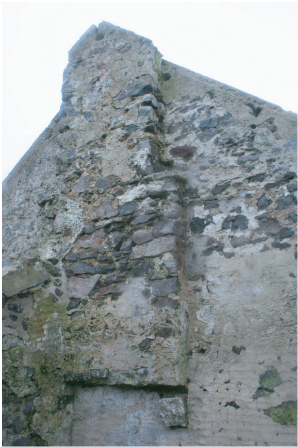
Plate 29: Corbelled chimney on southeast gable of northeast range
