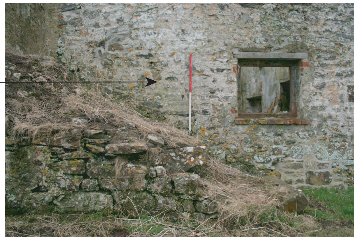
Plate 33: Northeast wall of northeast range, showing blocked opening behind steps
