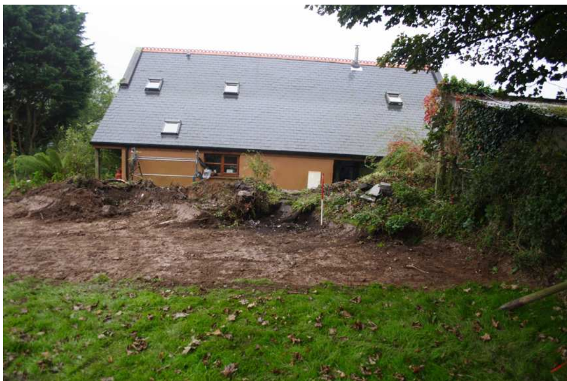
Photo 1: View south across the site during the topsoil strip.
