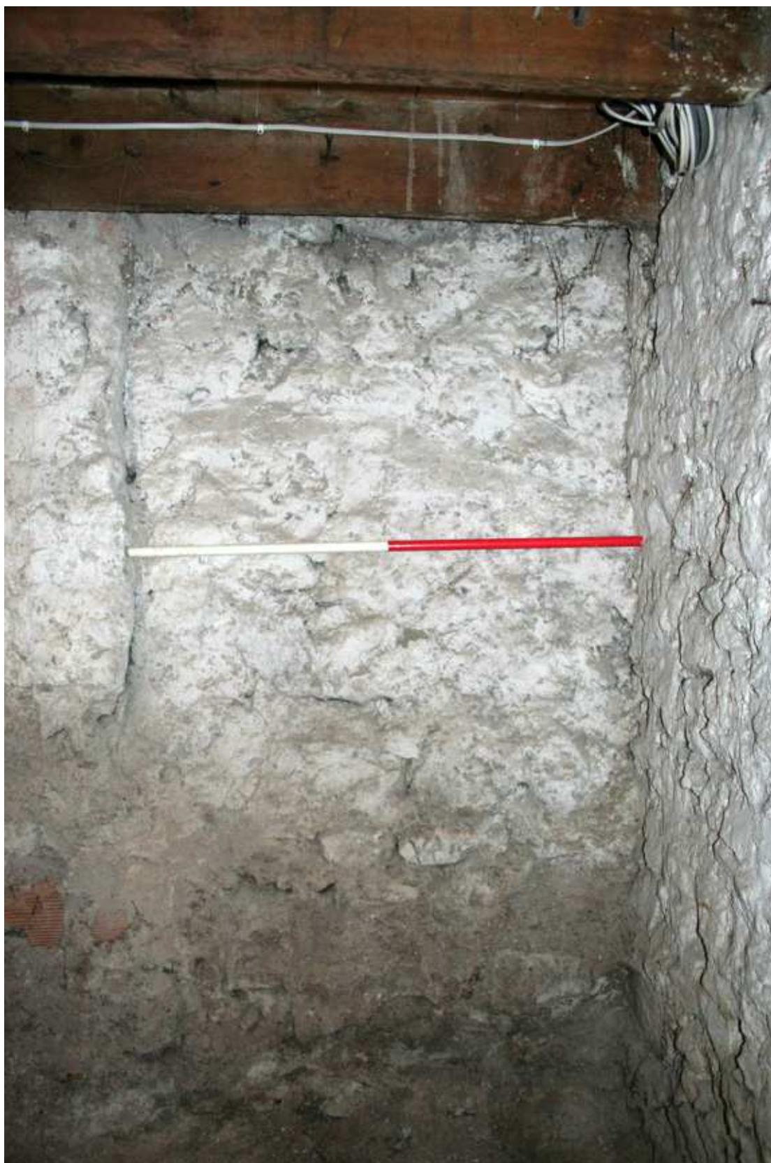
Photo I. Detail of blocked opening at the northern end of the west wall, the 1m scale is horizontal (8875).
