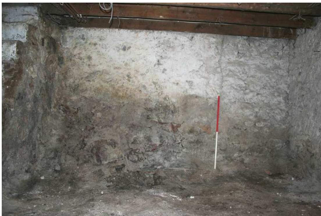
Photo H. West wall, note the vertical line of the blocked opening marked by the scale (8874).
