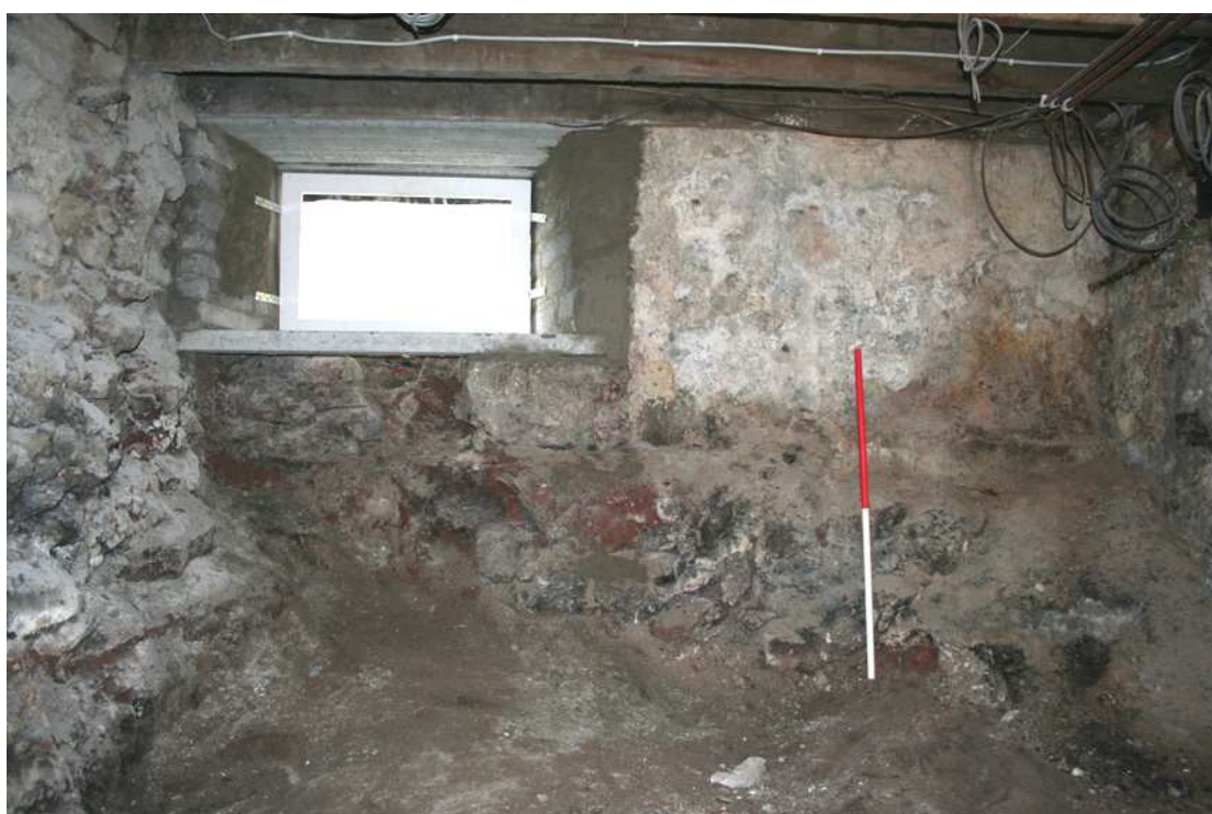
Photo D. East wall, with new window opening inserted (8866).
