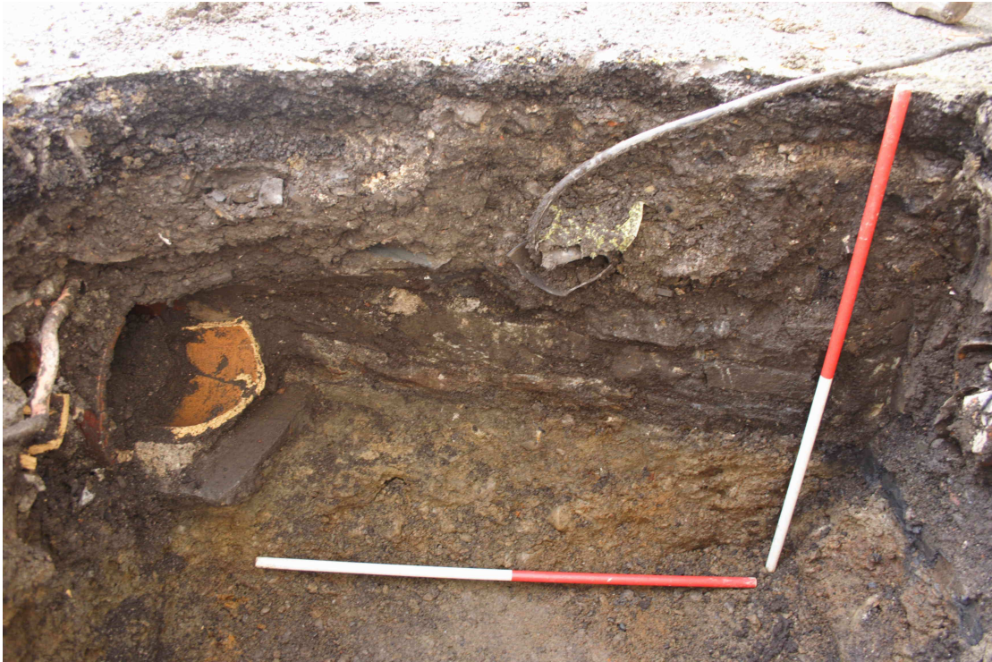
Plate 8: Stone built former drain showing later stoneware pipe.
