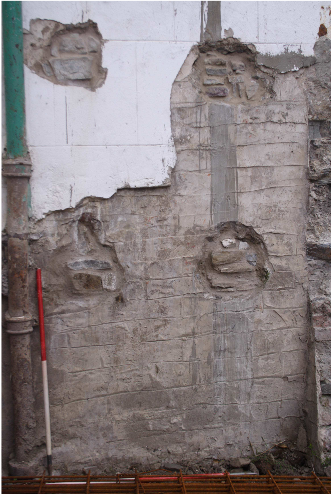
Plate 29: Lower section of southwest end of retaining wall showing concrete render and pinning scars, shot 11.
