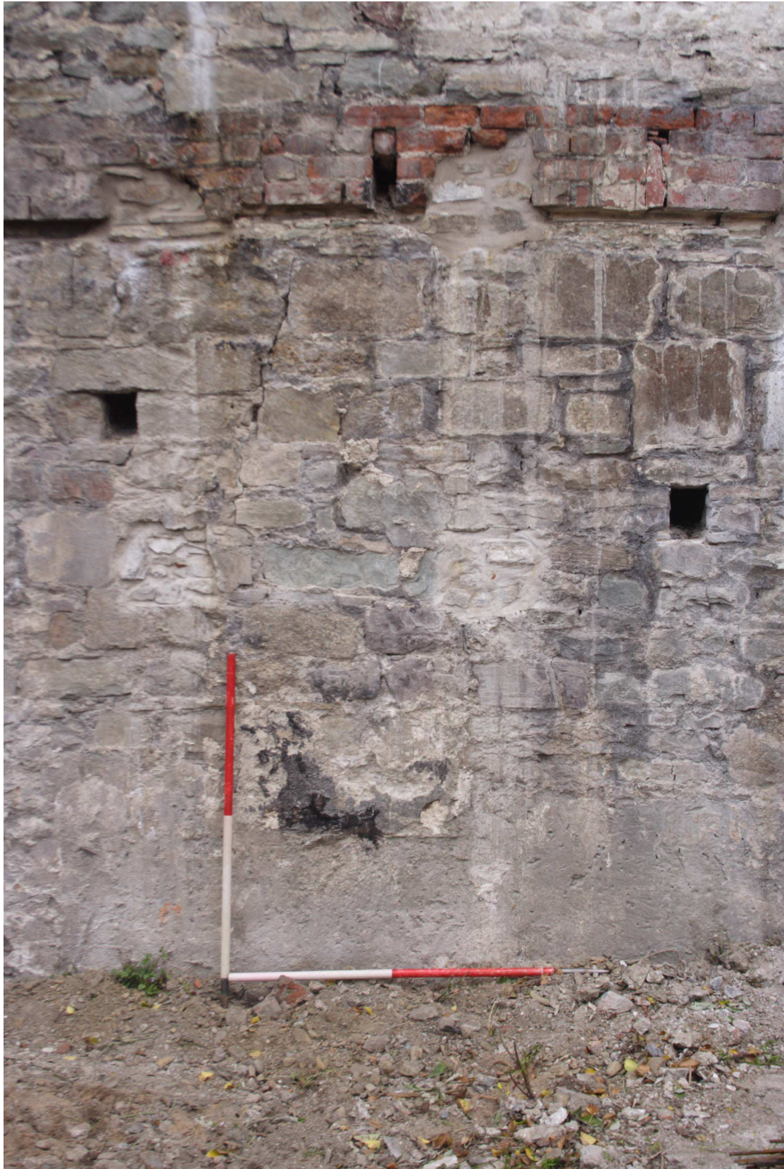
Plate 21: Lower section of retaining wall with putlogs visible. Floor joist slots of former cottage visible in upper image shot 3.
