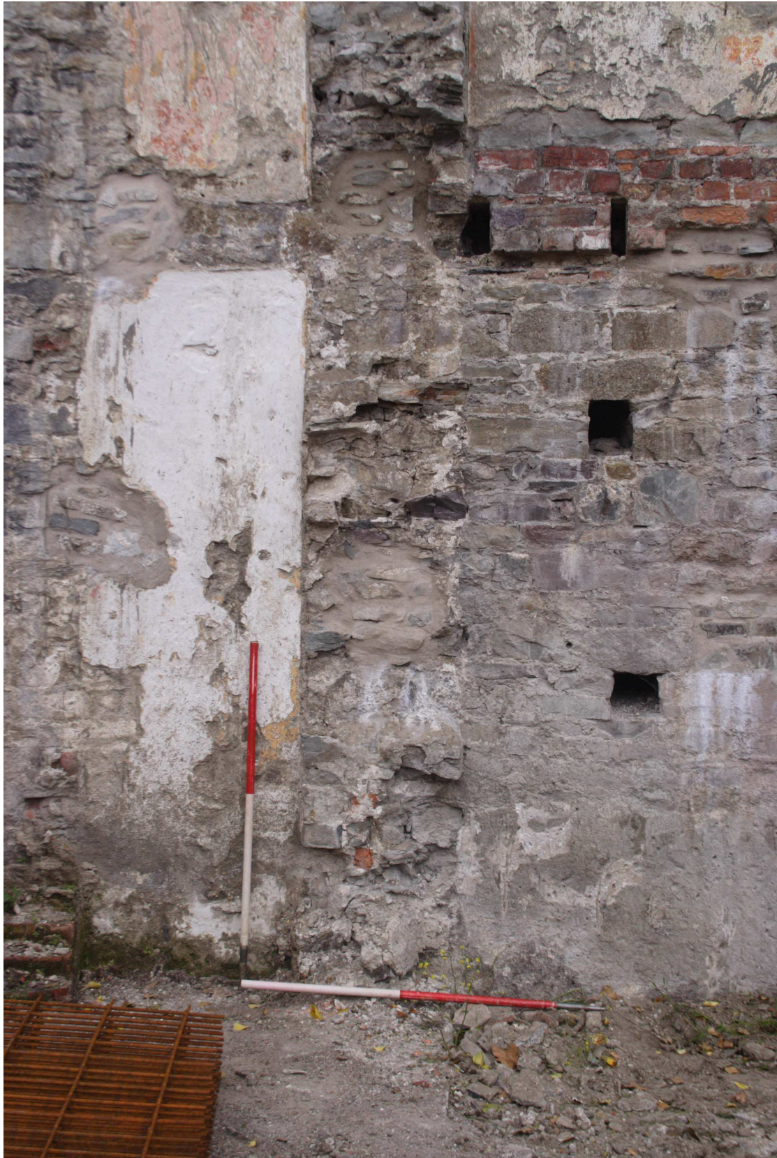
Plate 25: Lower section of retaining wall showing former gable end of cottage. Put logs visible to right along with floor joist slots of former cottage, shot 7.
