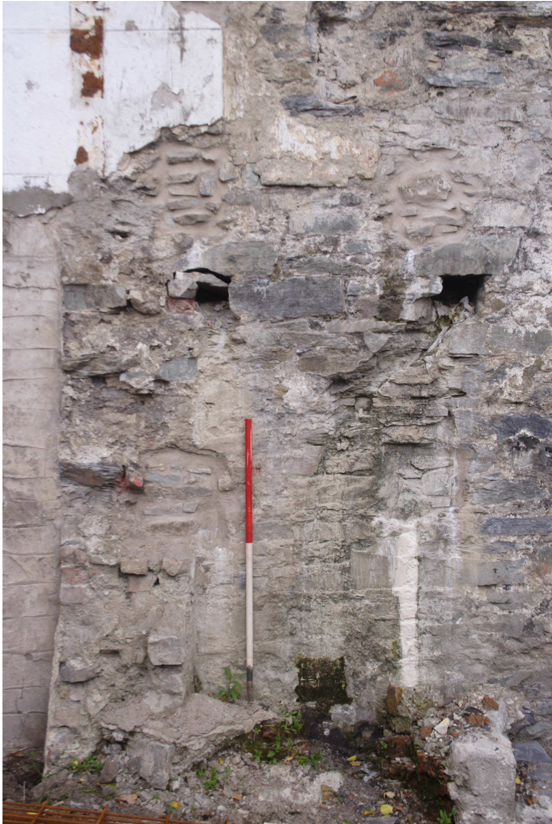
Plate 27: Lower section of retaining wall showing damaged putlogs. Former cottage wall to left of centre. Concrete render visible in upper left, shot 9.
