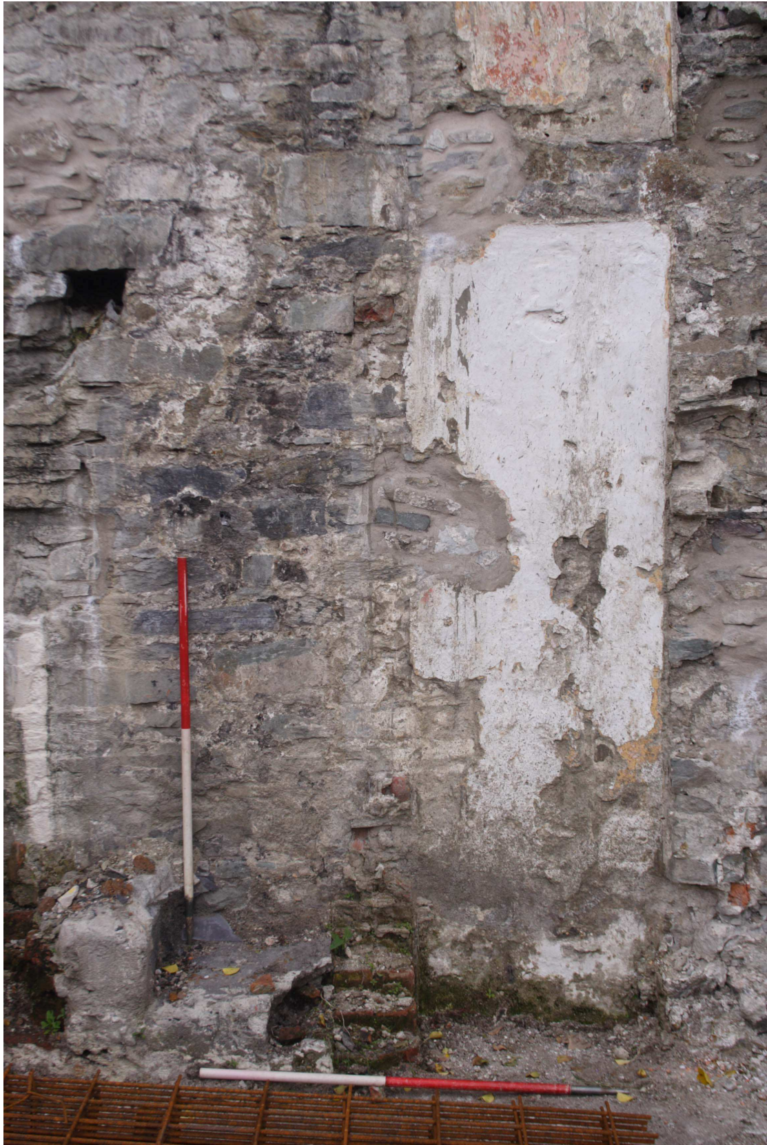
Plate 26: Lower section of retaining wall showing concrete render and unknown feature relating to cottage. Damaged put log in upper left hand edge of image, shot 8.
