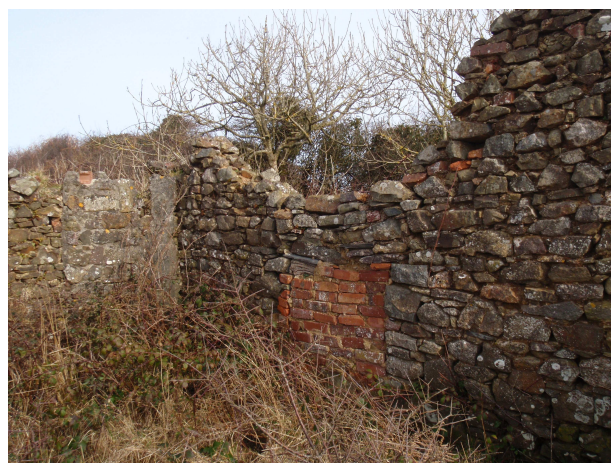
Looking southeast, blocked doorway and shored-up fireplace within Blaen-Llyn cottage
