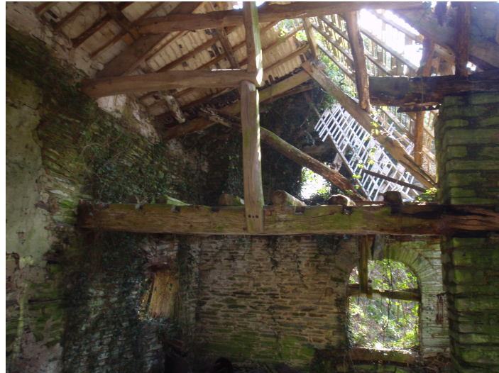
Collapsed timbers within northeast corner of Trefach Mill
