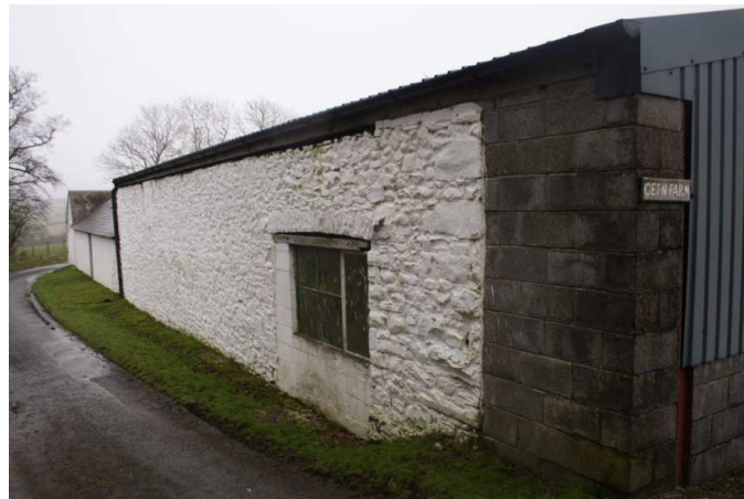
Looking northeast, rear wall of possible stable with blocked-up cart bay, with cow shed and cart shed in background
