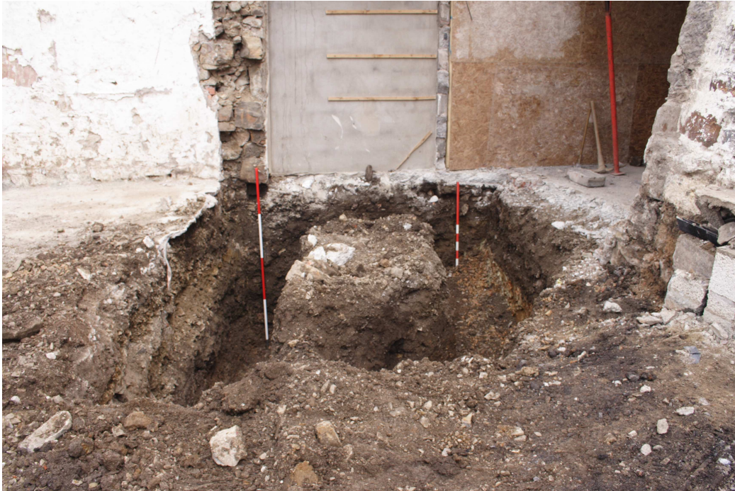
Photo. 2: Rear extension footing trenches and the east end (left) of the rear wall footing trench. View E. Scales 2m and 1m
