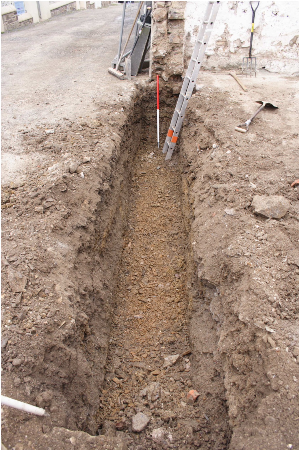
Photo. 4: Front wall footing trench, note clean shaley stone deposit in the bottom View E. Scale 1m
