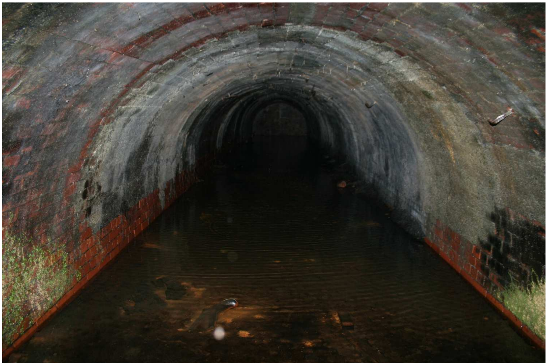
Plate 14: Interior of brick lined slant/ drain to west of Llwynceilyn
